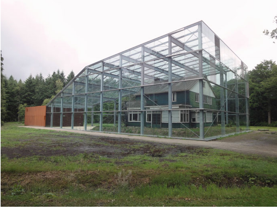
Fig. 11.3 The wooden house of the second World War Nazi camp commander in Westerbork the Netherlands. The original house and its contents are too fragile to be exposed to the harsh outdoor conditions. A display case was designed with a natural ventilation to maintain temperatures and relative humidities that will help preserve the building for future generations. The house can be visited on invitation only, while inside the display case on the back of the house special events, such as small classical music concerts, are to be organized
