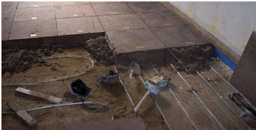
Fig. 10.4 Installing floor heating in the central hall of Amerongen Castle (Photo: Jos Snoek)
