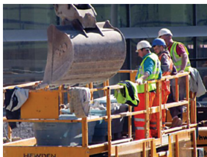
Filling containers with limestone from scissor platform
