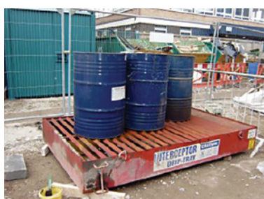
Oil spillage platform for the location of fuel drums, avoids fuel spillage problems
