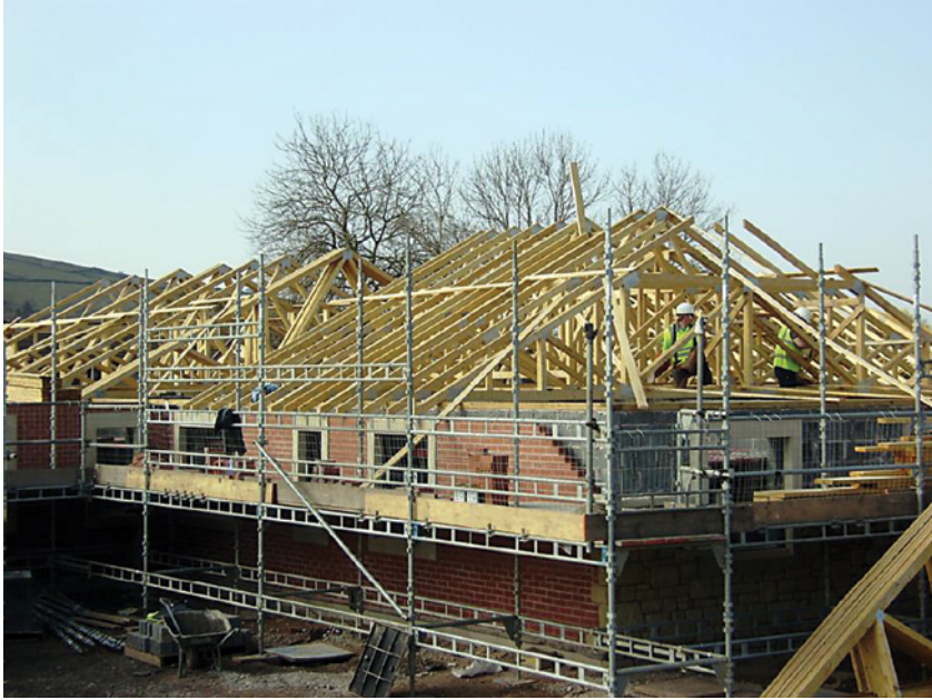
Work in progress in Area One. Progress after 5 days of work
