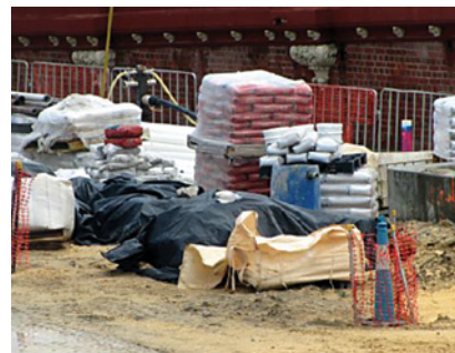
Materials stored on prepared ground adjacent to access roads
