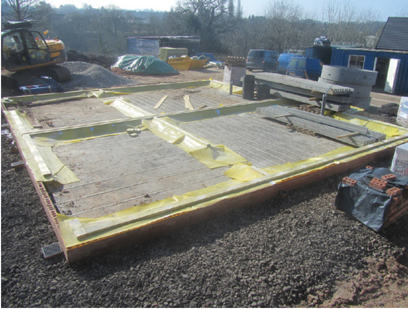
Beam and block ground floor slab
