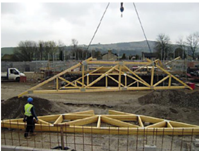
Unloading and lifting of 10m span trusses into position
