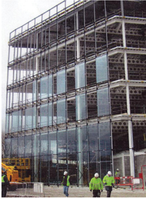
Glass curtain walling in progress to side elevations
