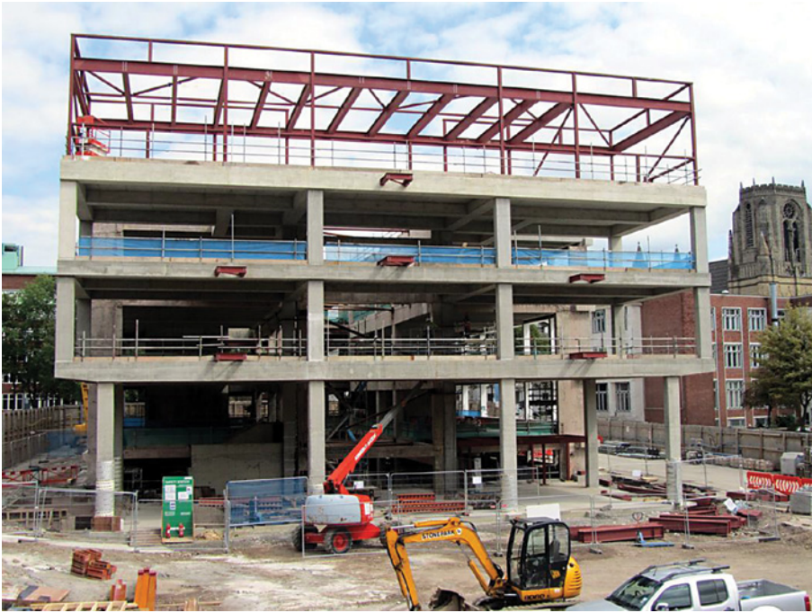
View of completed fourth floor steelwork
