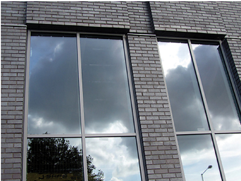
Brickwork in recessed panels above windows – an excellent quality finish
