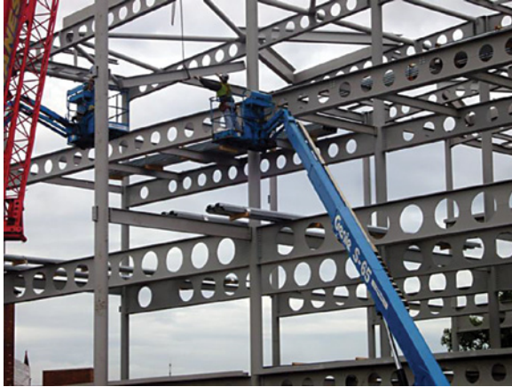
Four-storey steel frame
