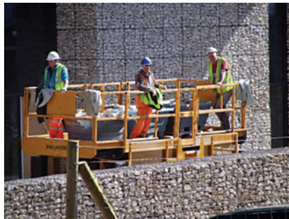
Transport of scissors lift platform to wall location
