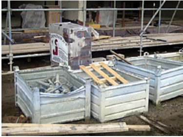
Use of storage container bins – easy to stack and handle containers of scaffold parts
