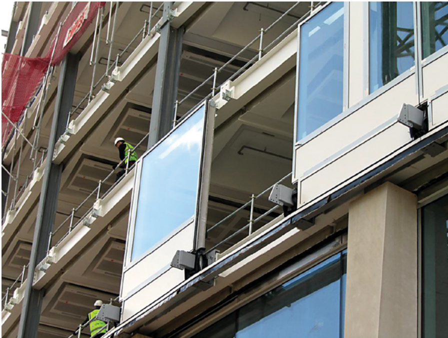
Curtain wall panel in position
