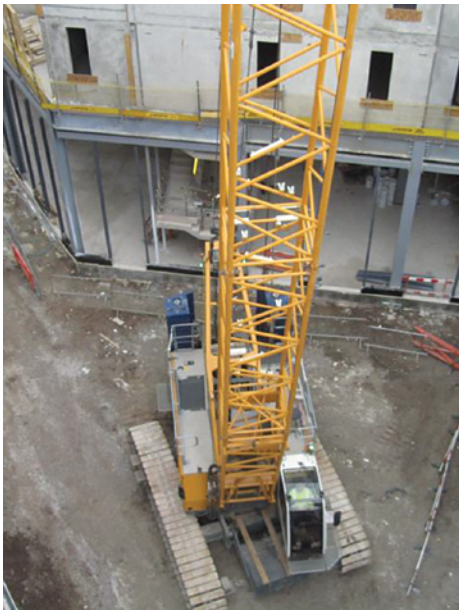
Large tracked mobile crane with fly jib between two buildings
