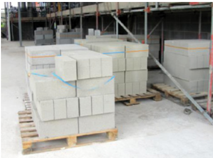
Blocks stored on pallets at each floor level in the office block
