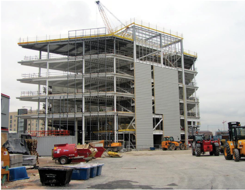
View of office block with cladding to rear elevation in progress
