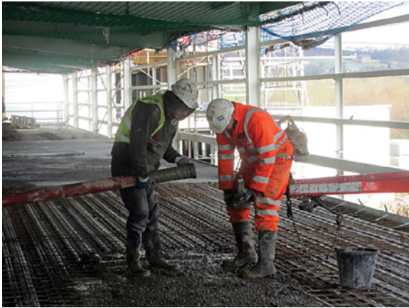
Setting up steel delivery pipes across deck to pouring location
