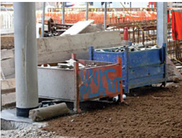
Scaffold and formwork fittings, stored in containers
