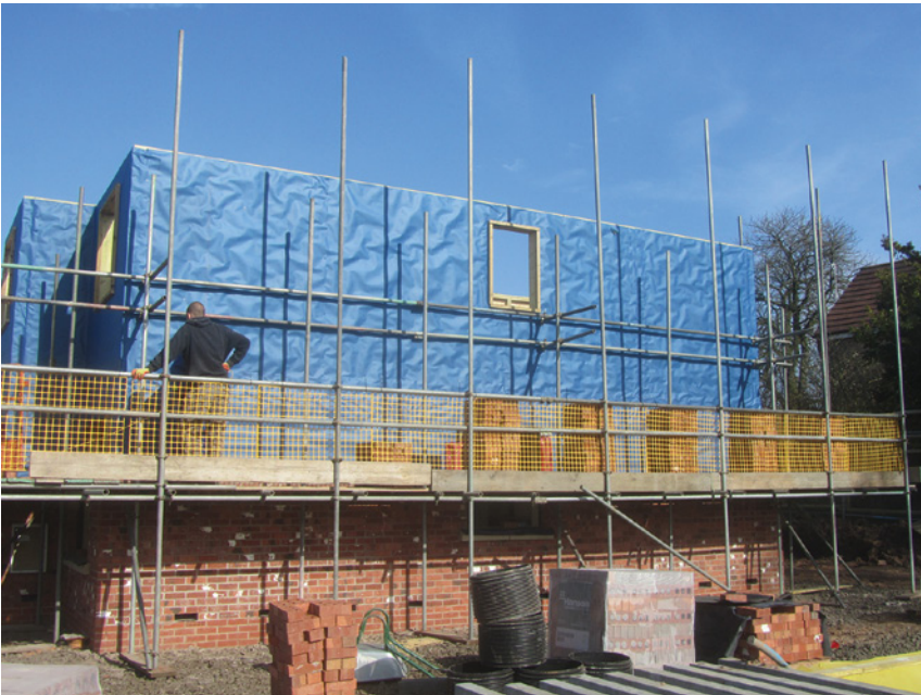
Wall panels to upper floor of semi-detached frame
