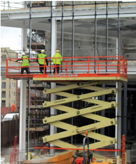
Use of aerial work platform (hydraulic scissors lift) capable of lifting to 5 or 10 storey
