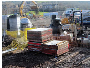
Wall panel formwork, stacked clear of ground after use
