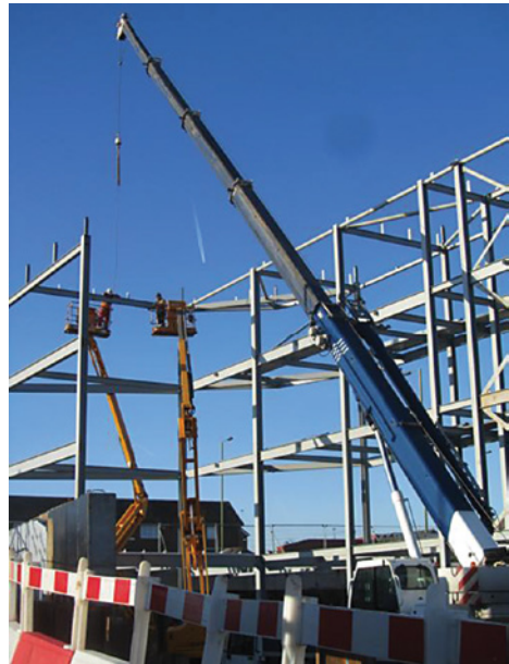
Lorry mounted crane with hydraulic jib
