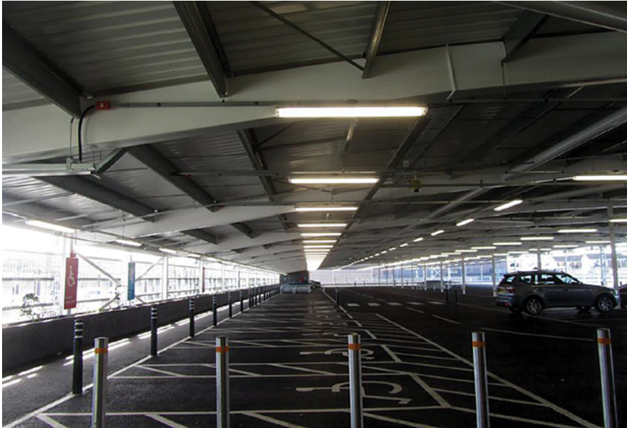
Roof to car park building
