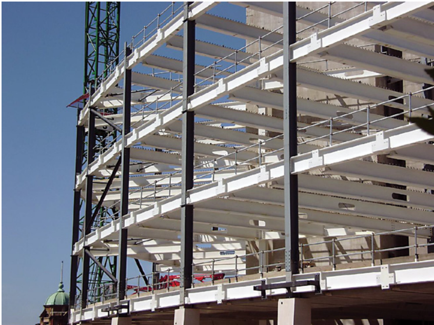
General view of floor steelwork
