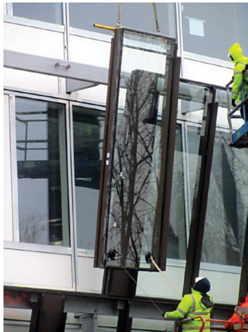
Lifting over cladding panels with tower crane
