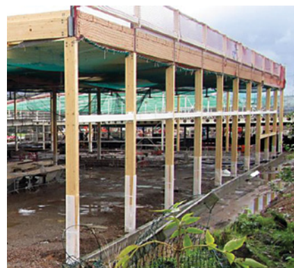
10 bays of timber laminated columns at 6 m centres
