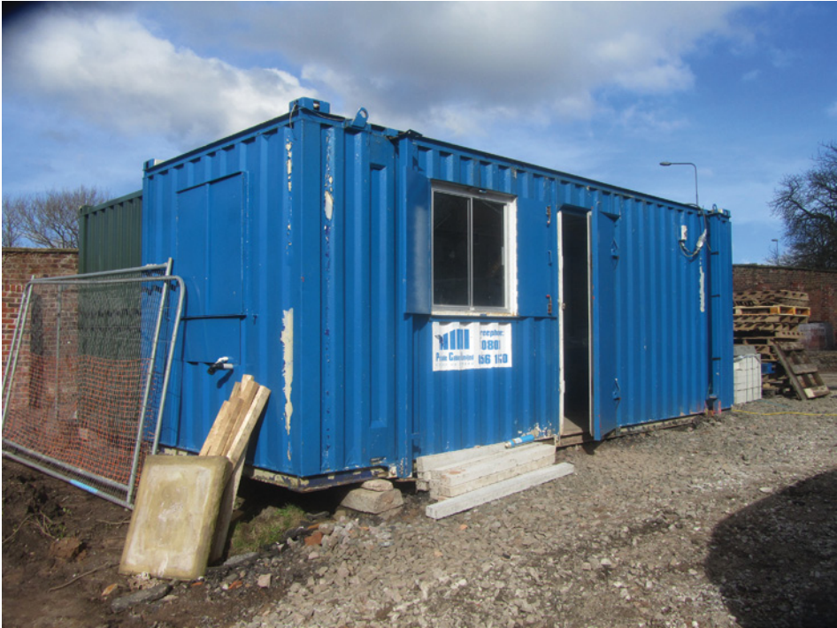
View of site office facility
