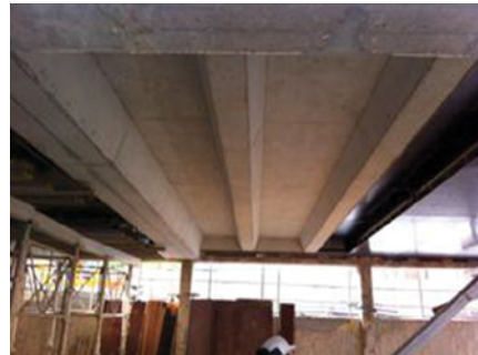
View on underside of floor slab showing prestressed troughed beams
