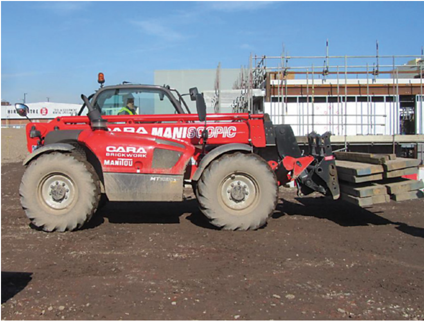
Used for moving materials around the site
