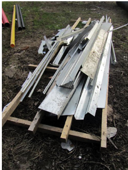
Surplus materials lying around the site at the contract completion – surpluses again created by over-ordering of materials during the contract Readers are advised to assess the cost implications of the four images shown.
