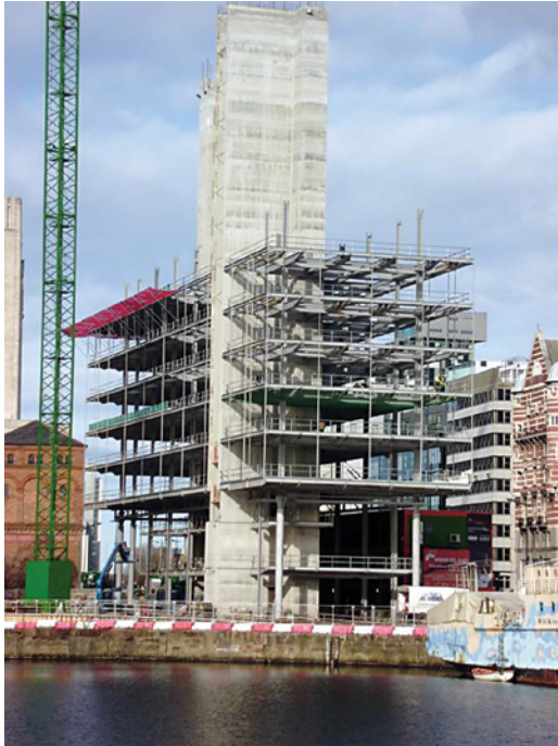
General view of staircase towers and steel frame
