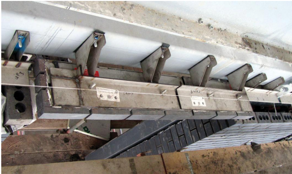
Brackets required to support the brickwork over the window openings
