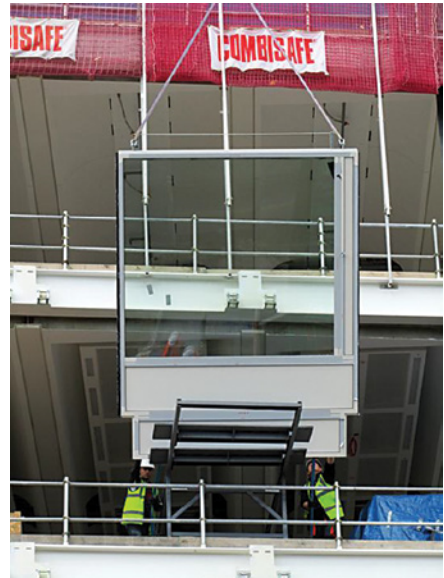
Panel guided clear of building frame
