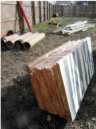
Surplus materials lying around the site at the contract completion – surpluses again created by over-ordering of materials during the contract Readers are advised to assess the cost implications of the four images shown.
