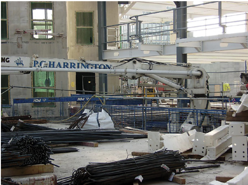
View of SCHWING mast pump (P C Harrington – work package contractor)
