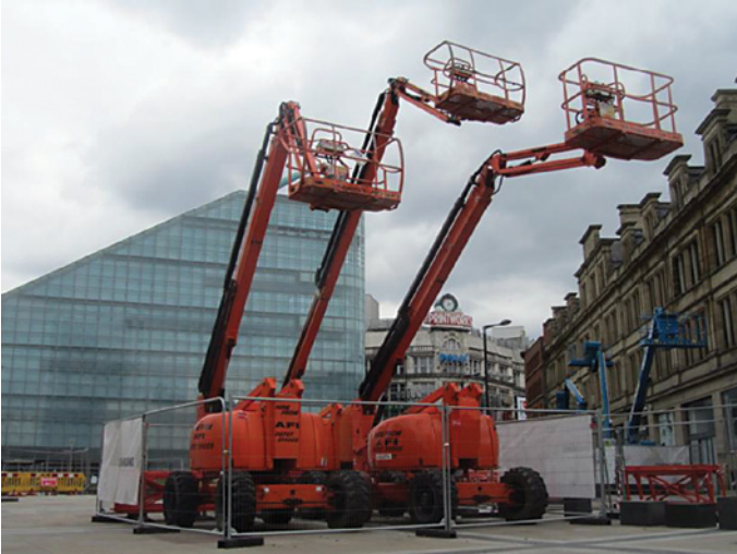
Three hydraulic lifters in a site compound
