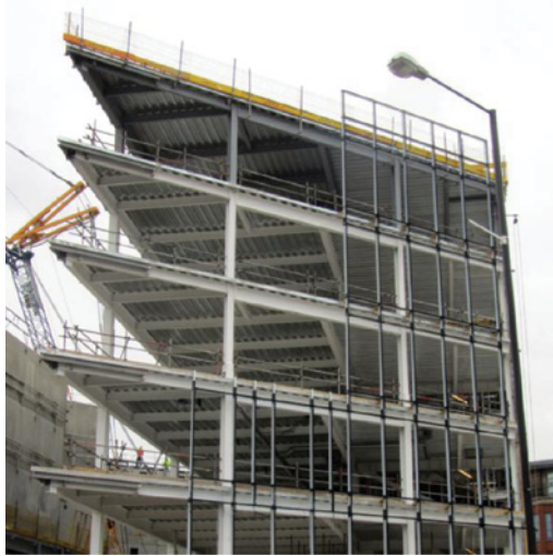
Steel frame with metal deck floors
