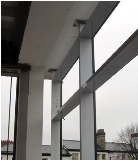
Aluminium framing bracketed to existing concrete frame at ground floor levels, floor edge beams and soffit to roof beams
