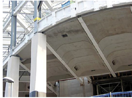
Second floor coffered precast units
