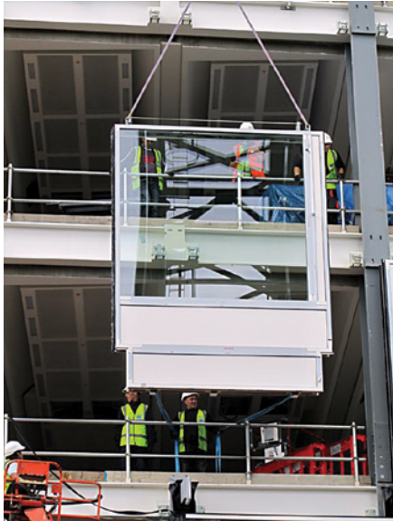
Panel lowered into position
