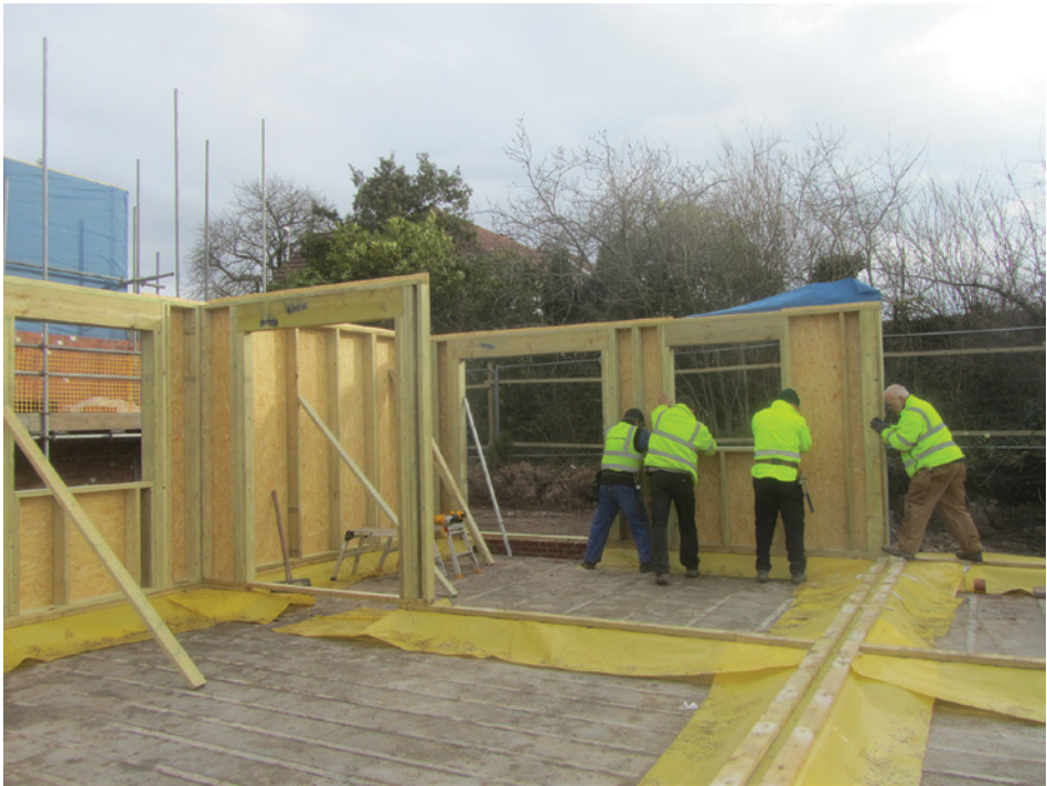
Commencement of erection of panels at ground floor level
