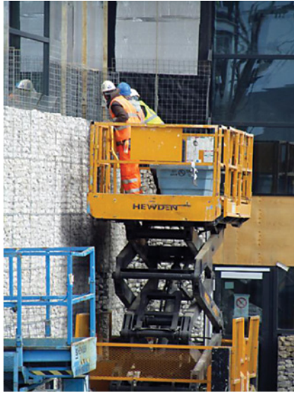
Filling gabion cages by hand in final position
