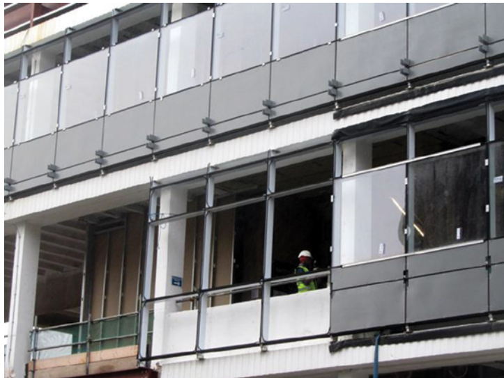
Image of side elevation of building
