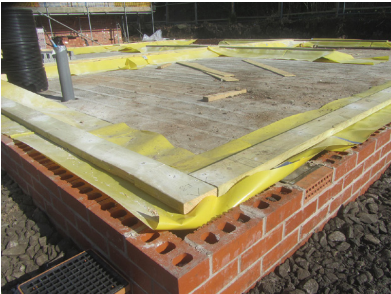
Sole plates for wall panels 150 mm x 40 mm
