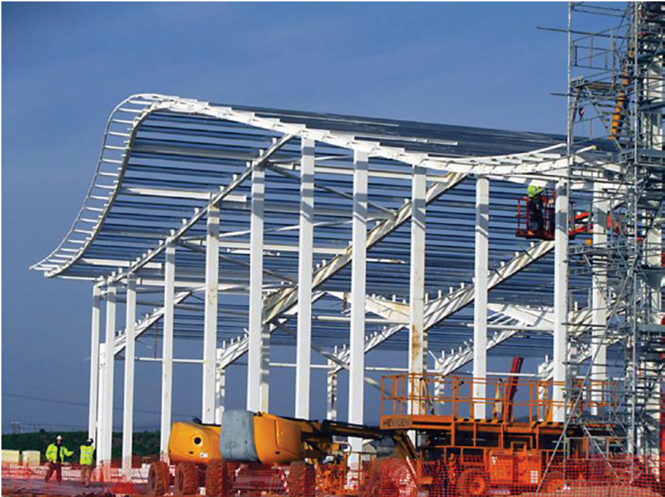
View of wave roof as purlins and overhang are completed
