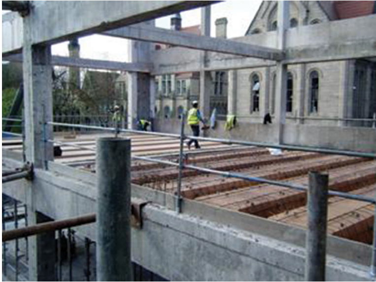
Stripped back frame with new floor formwork in position
