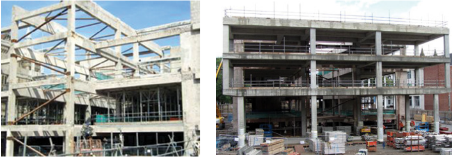
Images of the “striped back” reinforced concrete frame
