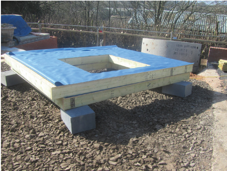
Site fabricated 150 mm wide internal and party wall panels
