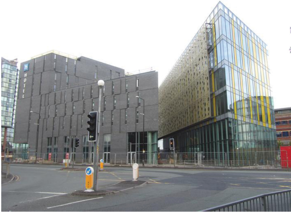
View from the road elevation of the hotel and office block complex
