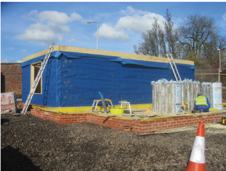
Erection of ground floor panels to plot 1
