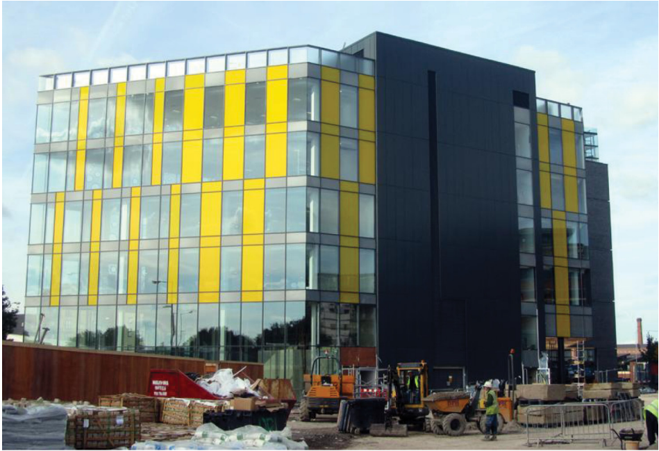
Six storey steel frame office building with front and side elevation finished in feature yellow panels, and two-storey retail unit to ground floor area
