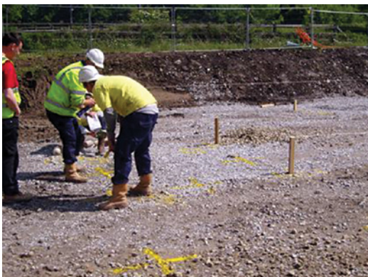
Engineer and foreman setting out pile position from string lines
