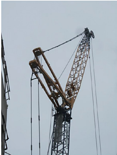
Track mounted mobile crane fitted with an extended fly jib
