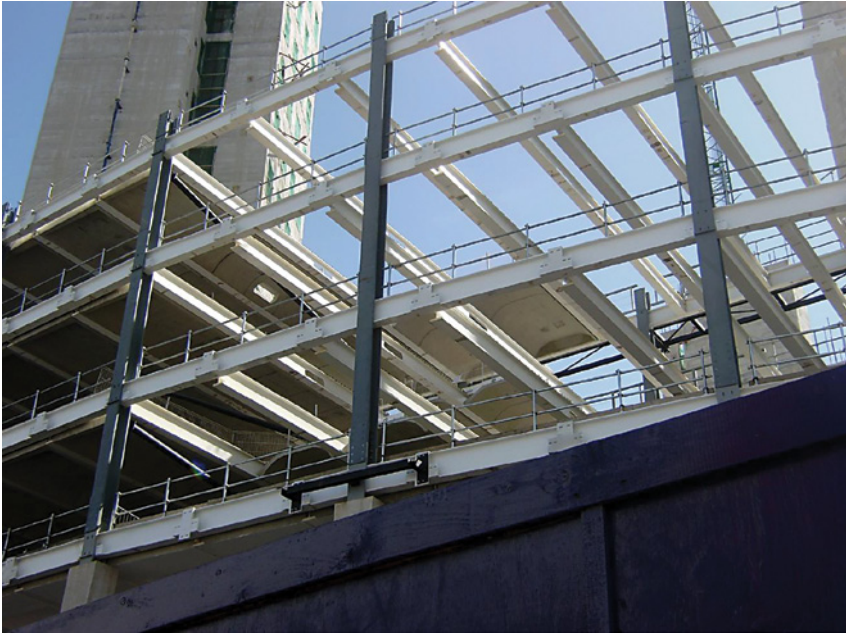
Position pre-cast coffered units between steelwork to floors 3,4 & 5
