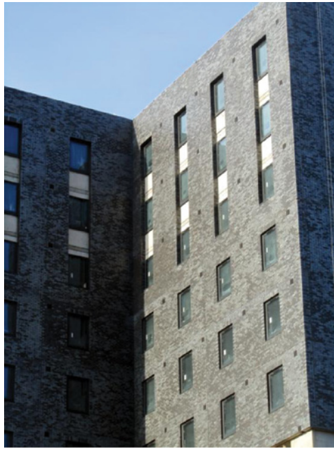
Example of composite wall panels on a similar hotel project, with composite blue brick external storey-height panels
