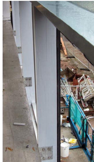
Aluminium framing bracketed to existing concrete frame at ground floor levels, floor edge beams and soffit to roof beams
