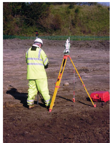
Freelance engineer setting out on virgin site
