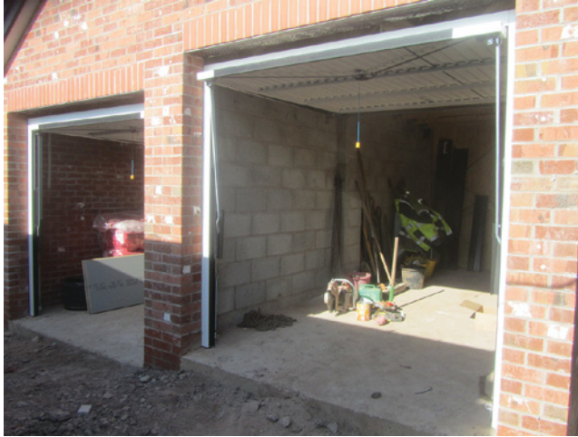
View of double garage facility
