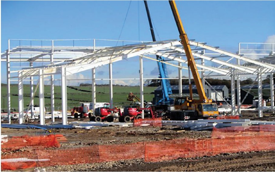
Erection of bay 2 in progress
