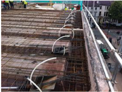
Post tensioning tendons shown in position at each troughed beam
