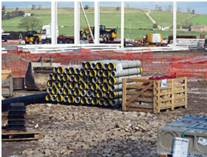
Site material storage
