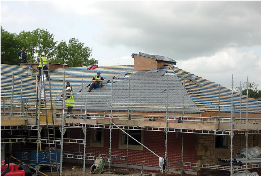
Slating to main roof in progress
