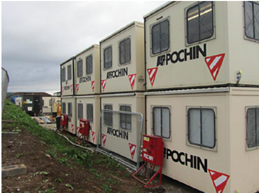
Eight tiered fully serviced mobile offices making up the main contractor's and design team accommodation
