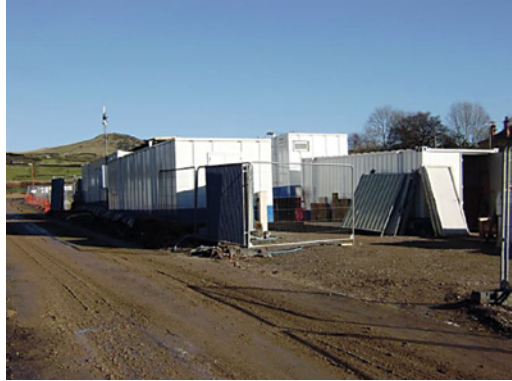
Site compound area
