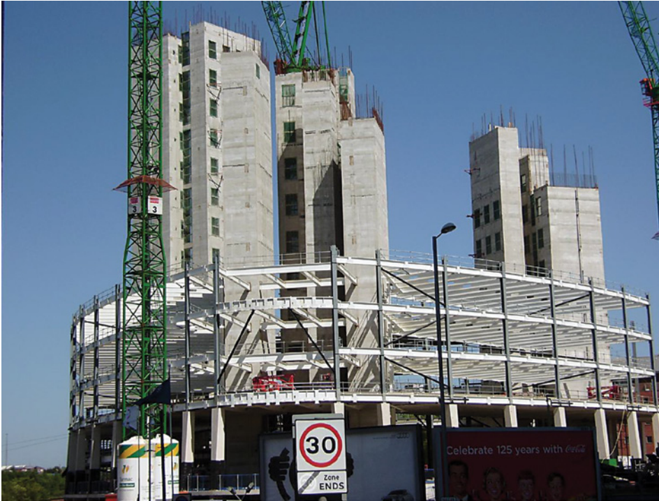
Image of building with steelwork at 5th floor level
