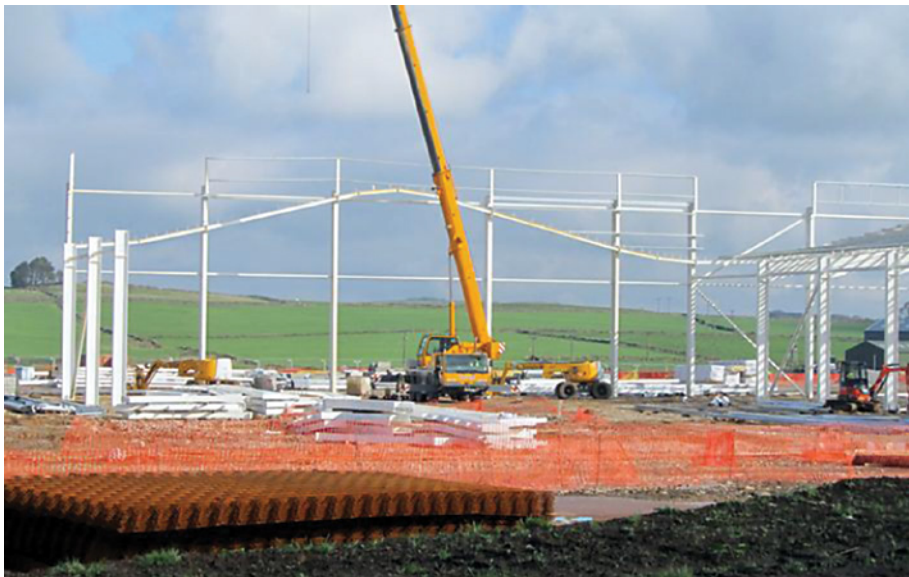
Commencement of bay 2: gable frame
