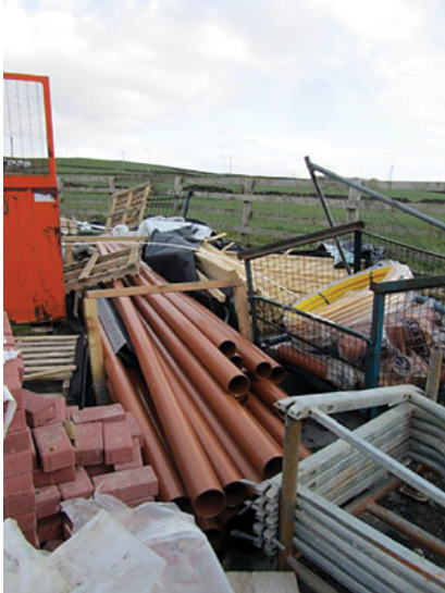
A disorganised storage compound – situations of this type occur towards the completion of a project, often resulting from the over-ordering of materials
