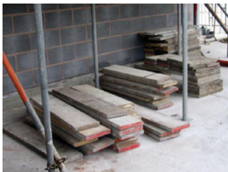
Scaffold boards stacked under a wall scaffold area
