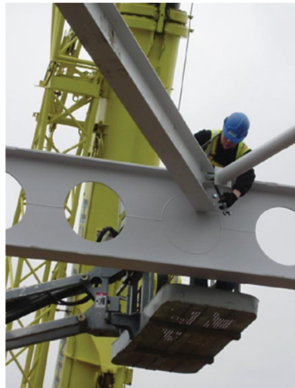
Fitting bolted connections from platform
