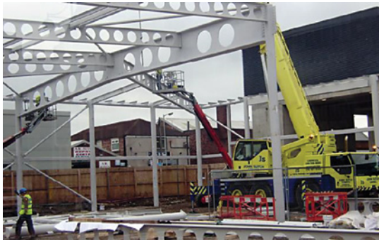
Single-storey frame erected with separate hydraulic mobile crane and lifters
