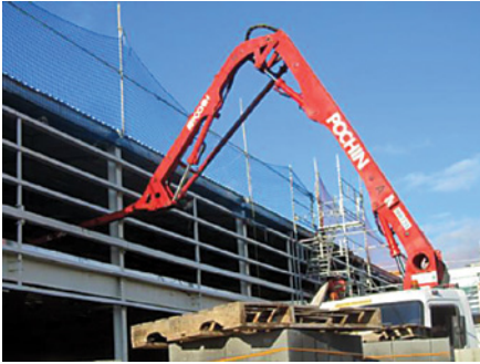
Mobile concrete pump located adjacent to bay pour. Pour commenced 8am – completed in 5/6 hour period
