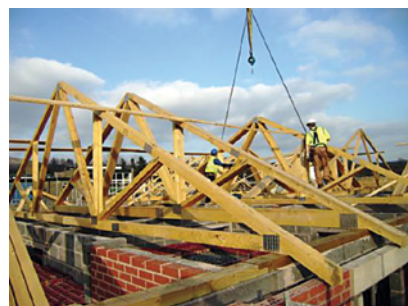
Trusses positioned in Area One
