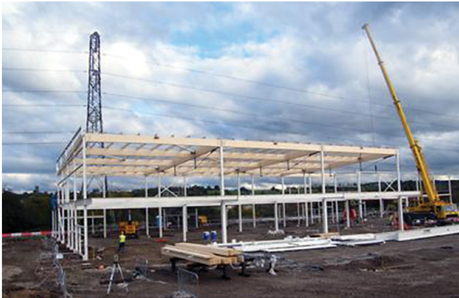
Bay 1 – frame erection day 5–7 on programme
