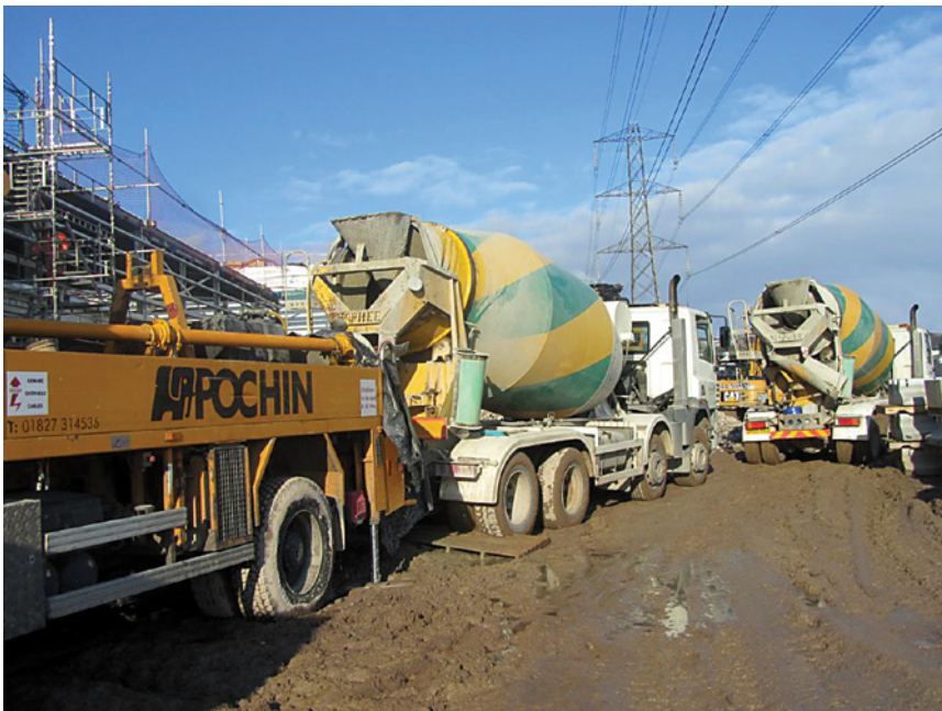
Ready mixed concrete supply vehicles feeding 120 cm floor pour
