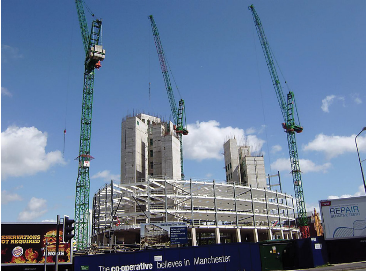
Tower cranes on site
