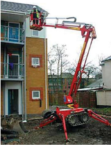
Track mounted lifter with stabilisers
