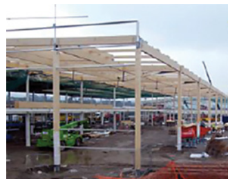
Bay 4 – frame erection day 14–15 on programme
