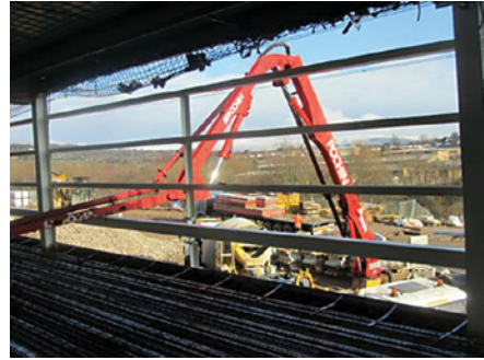
Mobile concrete pump located adjacent to bay pour. Pour commenced 8am – completed in 5/6 hour period
