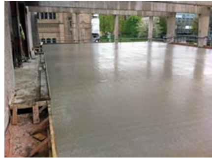
Floor slab poured in two 100 cm pours
