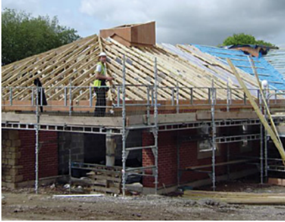
Completion of structural timber work and roof vents
