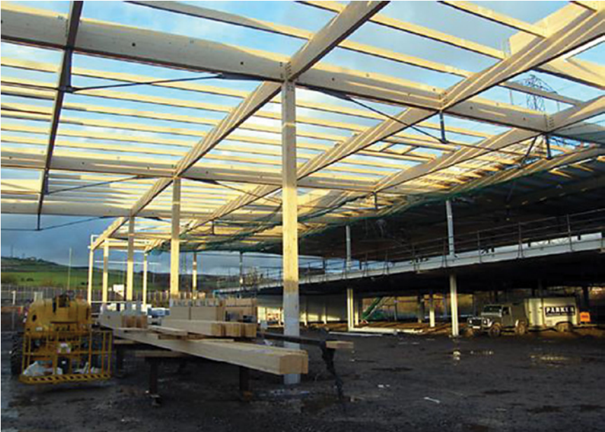
Internal view of roof structure on 6m x 18m long grid.
