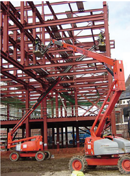
Erecting steelwork to a six-storey frame
