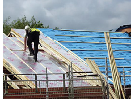
120 mm insulation to roof area prior to felting and battening
