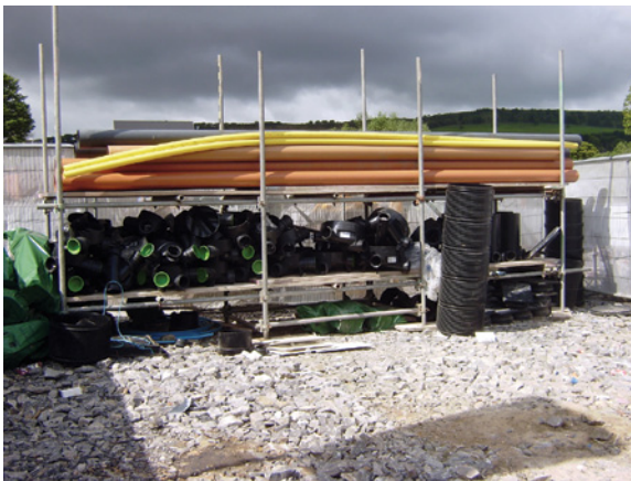
Taylor-Wimpey site showing good site materials control policy
