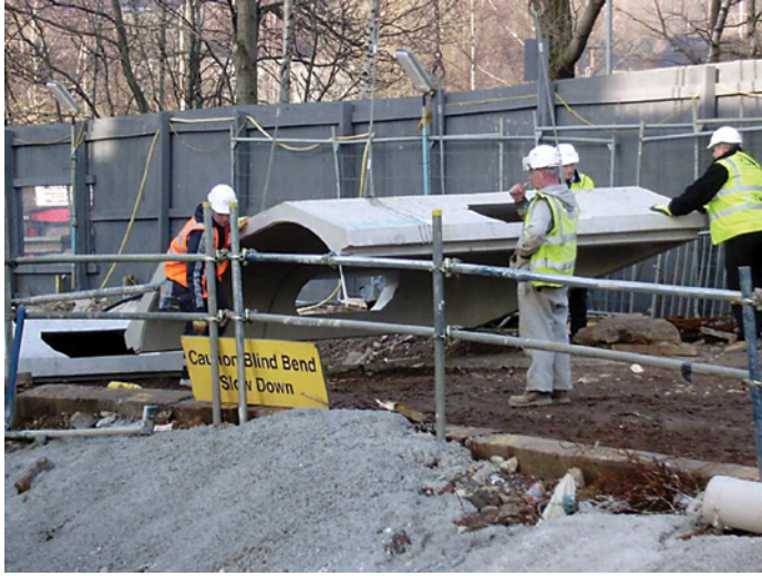
Handling pre-cast floor units
