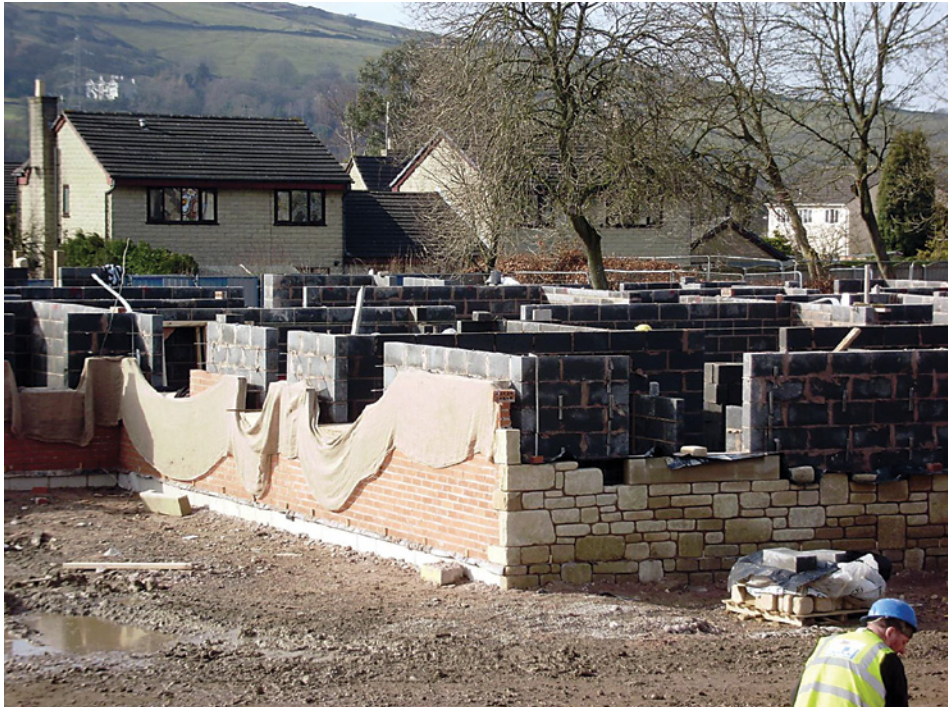
The residential block- blockwork and brickwork to first lift
