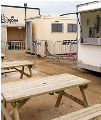
Site covered smoking area plus site canteen unit serving hot food
