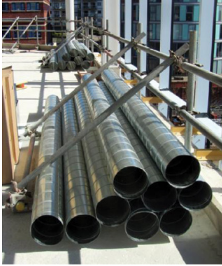
Ducting stored at each floor level strapped to adjacent handrail
