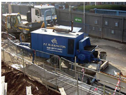
A: Position of static concrete pump unit on access road
