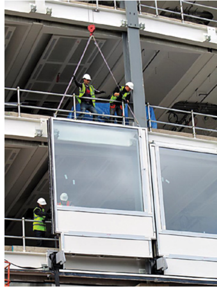
Panel moved into position and secured in fixing slots
