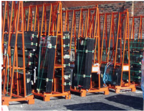
Glass storage racks for curtain walling material
