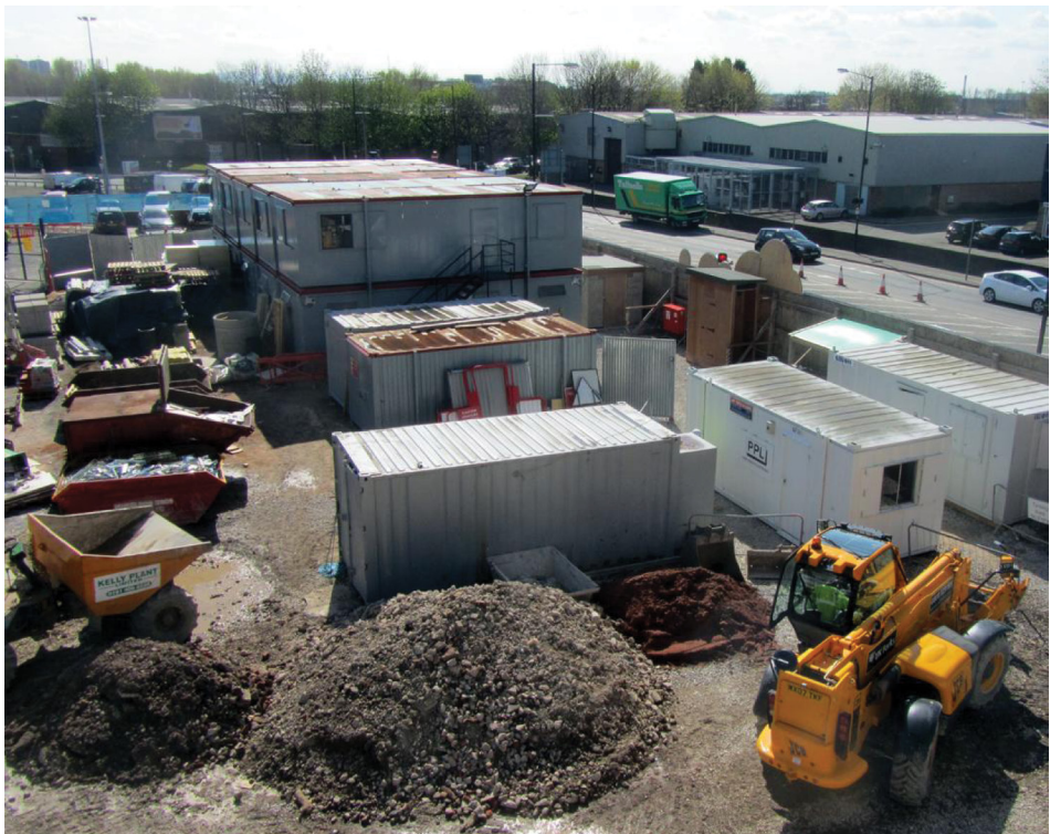
Contractor's main office set-up and subcontractors' storage areas
