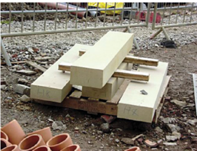
Stone lintels stored for ease of handling
