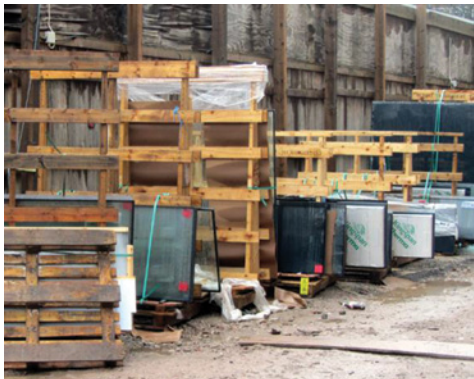
Storage racks for vertical storage of curtain wall storage panels.
