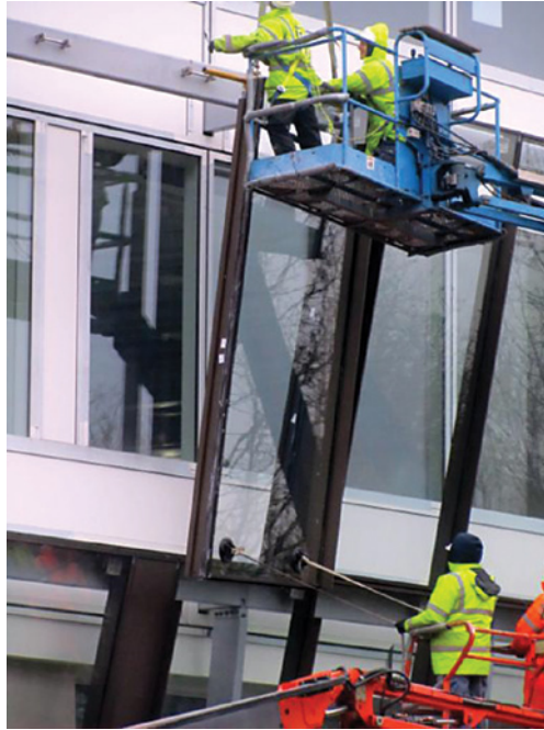
Positioning top and bottom of panels from cherry pickers
