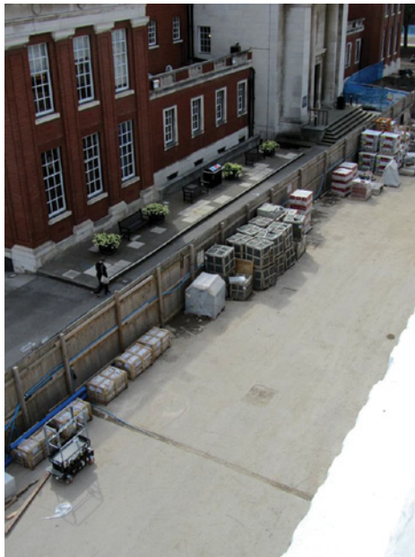
Storage adjacent to site access road
