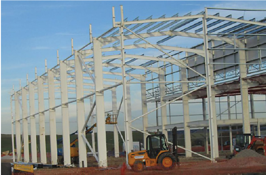
Completed high bay portal
