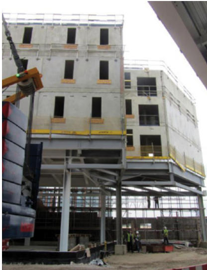
Crosswall construction at third floor level
