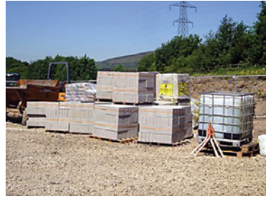
Well-planned storage areas prior to delivery – storage on pre-prepared areas – blocks and water stillage
