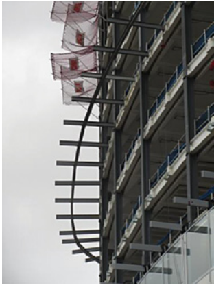
Fixing of mono-rail support
