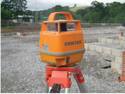
A Pentax laser level in use for foundation work
