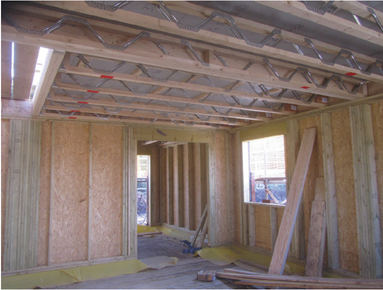
Internal timber frame and floors
