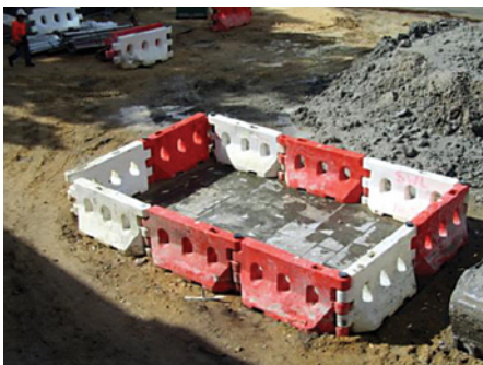
Road barriers set up to contain specific sub-contractors' materials and equipment.
