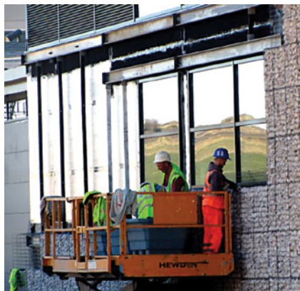
Vertical support rails for tying gabions back to wall
