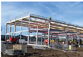
Bay 2/3 – frame erection day 8–10 on programme
