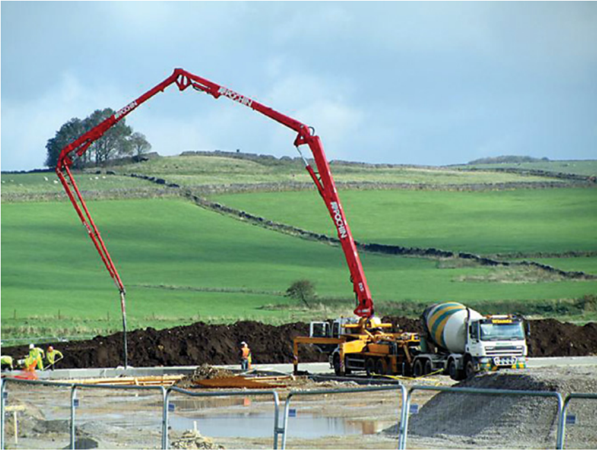
Commencement of concrete pumping to rear access road area
