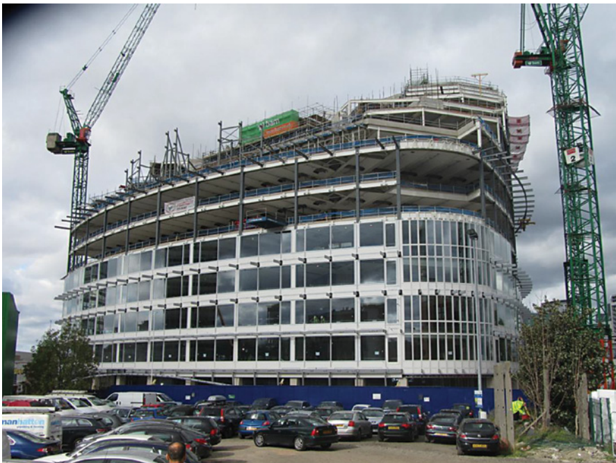
Wall panels completed to 6 th floor using handling method previously shown
