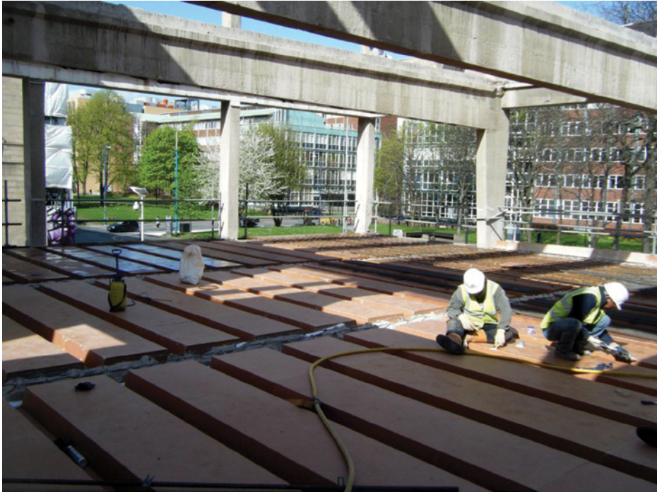
The utilisation of the formwork
