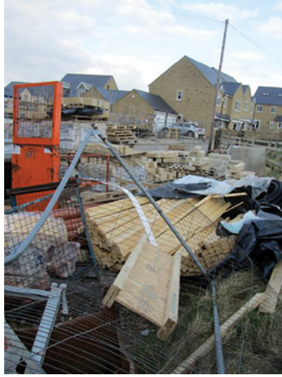
A disorganised storage compound – situations of this type occur towards the completion of a project, often resulting from the over-ordering of materials
