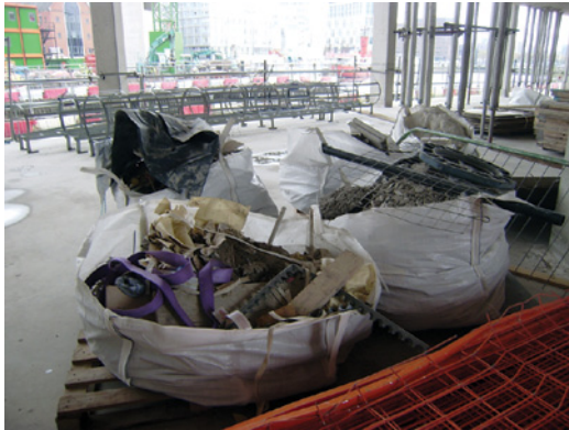
Large plastic storage bags used for collecting materials – to be handled by fork lift trucks
