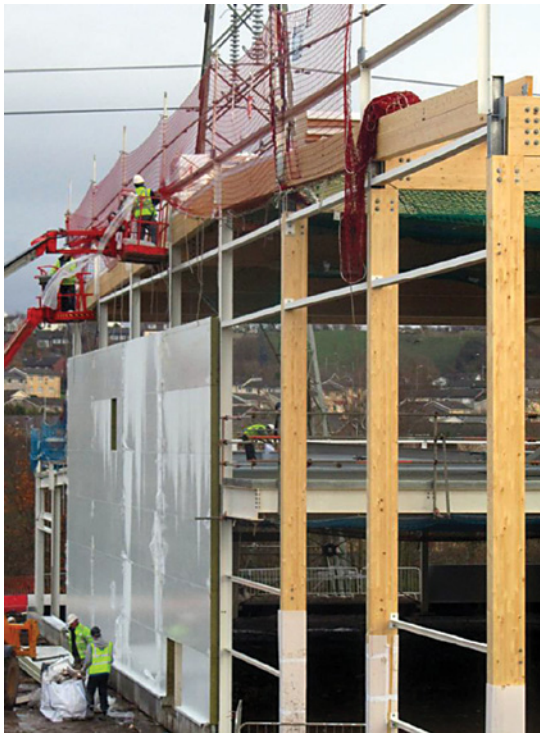
End gable frame showing insulated SIP timber cladding panels
