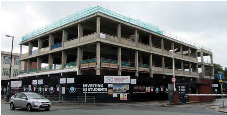
Building refurbishment and extension
