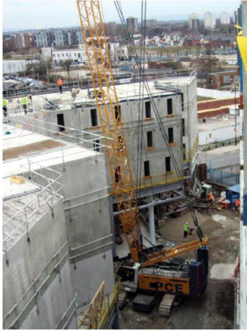
Crosswall construction at third floor level
