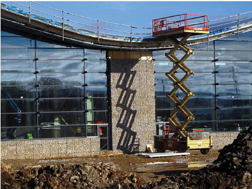
Feature gabion panels between portal bays, gabions filled with stone from scissor left platform
