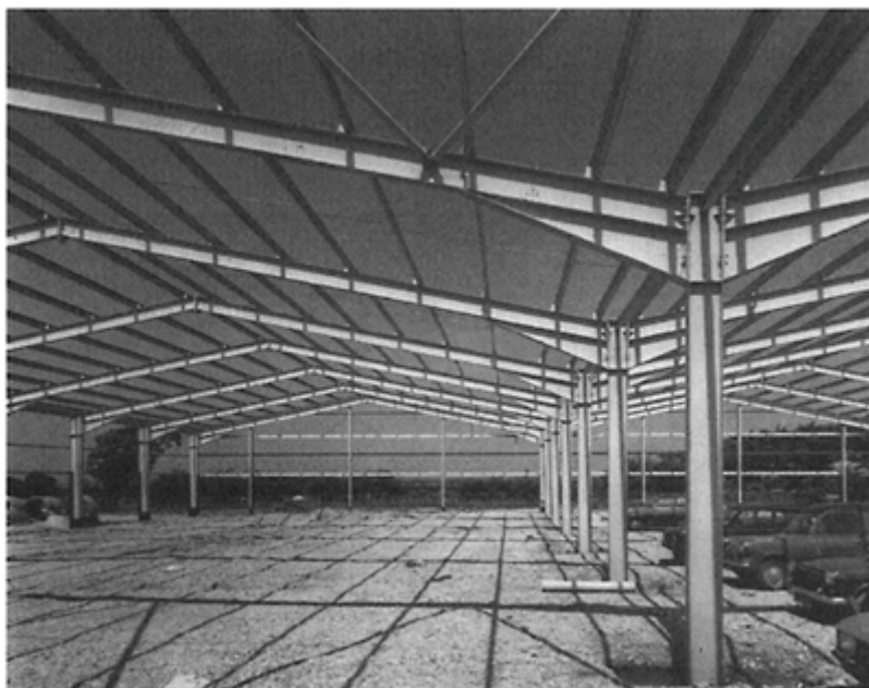
Figure 10.8 Typical portal frame structure during erection. (Courtesy of Condor Midlands, Burton-on-Trent)
