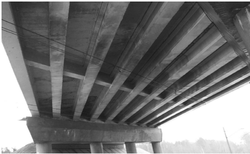
Figure 4. Bridge bottom view.
