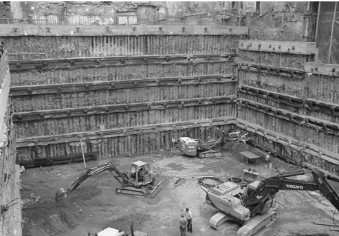
Figure 9. Erection of a temporary platform.
