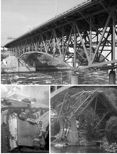
Figure 2. Collapse of the bridge over the Mississippi River in Minneapolis (August 1st, 2007).
