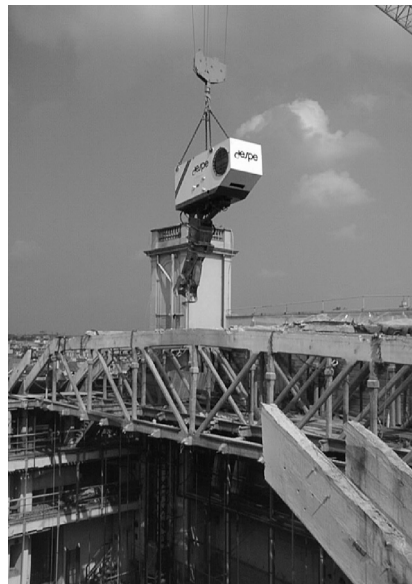
Figure 7. The cutting of the roof truss beams.
