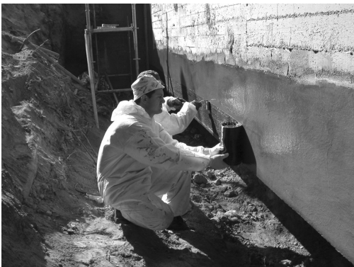
Figure 3. Application of CFRP sheets on the beam.
