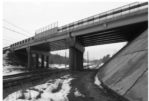
Figure 1. Bridge lateral view.
