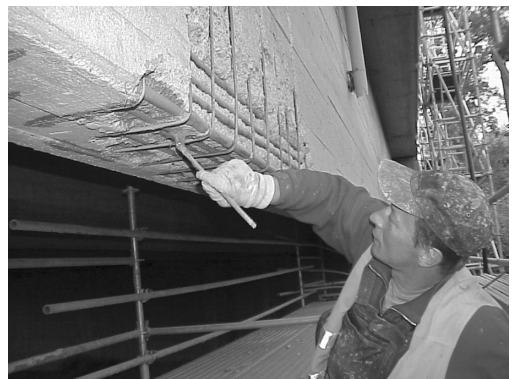
Figure 2. Rust-proofing of uncovered steel reinforcement during preliminary operations.
