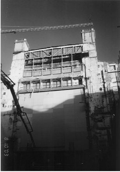
Figure 8. Internal view after demolition.
