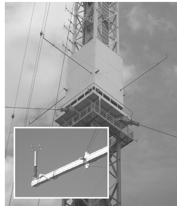
Figure 1. Covered part of the guyed mast Gartow II at 66 m.
