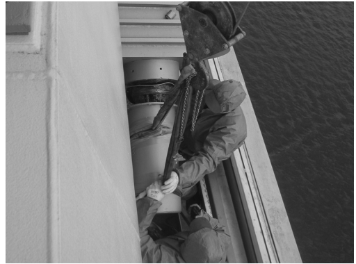
Figure 7. Preparation for lift-off test.
