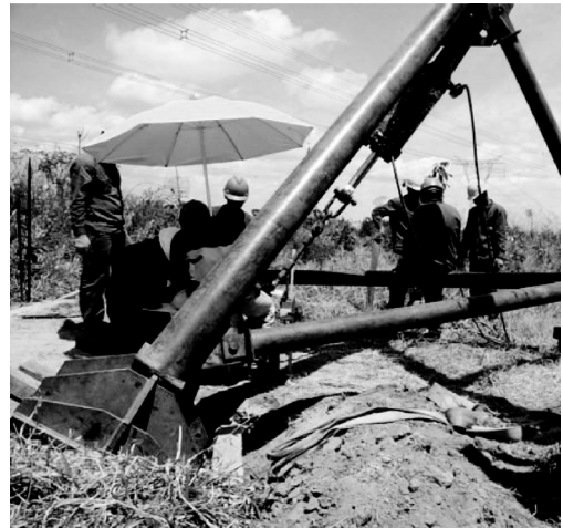
Figure 2. General view of the pull-out test (Azevedo 2006).
