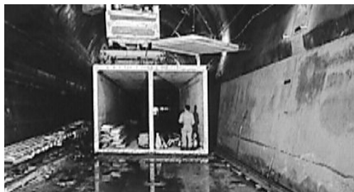
Figure 2. Archive photo: positioning of precast box segments and lateral haunches.
