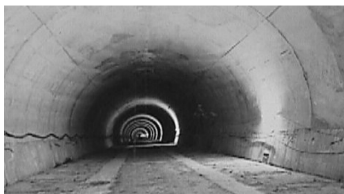
Figure 3. Archive photo: the internal structure finished.
