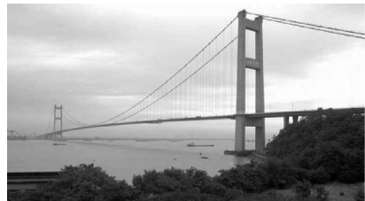
Figure 1. General view of Jiangyin suspension bridge.
