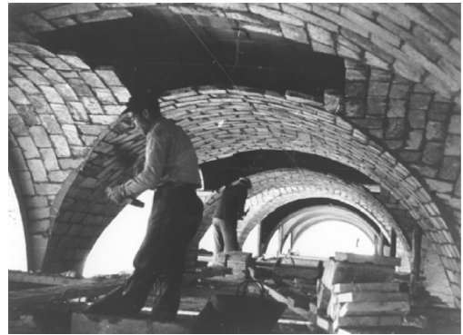
Figure 4. The brick vaults during the construction phase.
