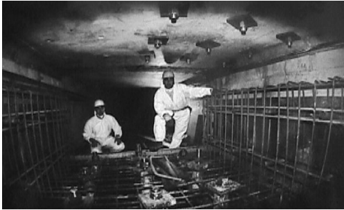
Figure 7. Provisional abutment—anchorage of the box.
