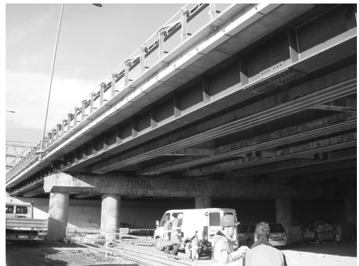
Figure 5. Battiferro-Navile Viaduct. General view during widening and strengthening operations.
