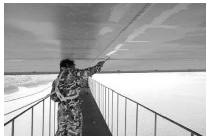
Figure 12. Rust cleaning of girder.
