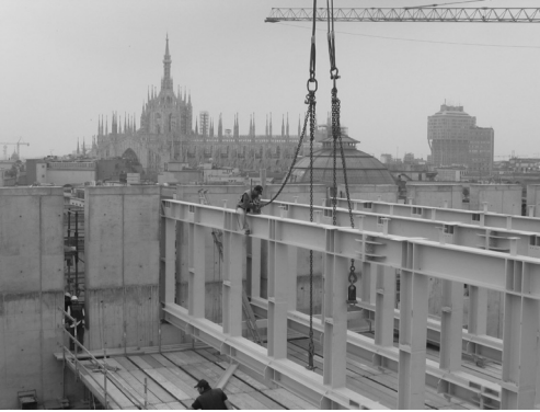
Figure 13. Steel Vierendeel beams of the roof.
