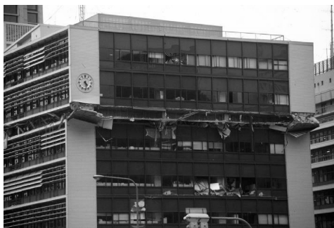
Figure 1. Mid-height collapse, Kobe, Japan, 1995.
