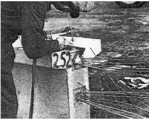
Figure 2. Finalising the post-tensioning procedure on a beam (Coombs 1957).
