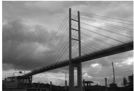
Figure 1. Cables of the bridge crossing the Strelasound.
