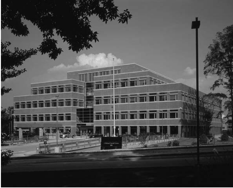
Figure 8.21 LEED Gold headquarters of PNC Global Investment Servicing.
