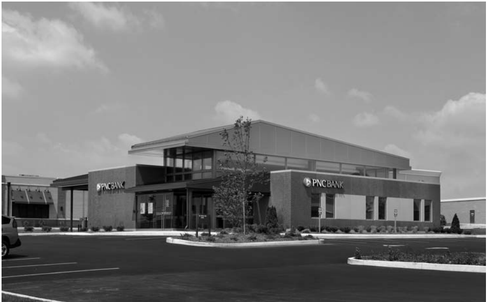
Figure 8.28 Green Branch® prototype constructed.
