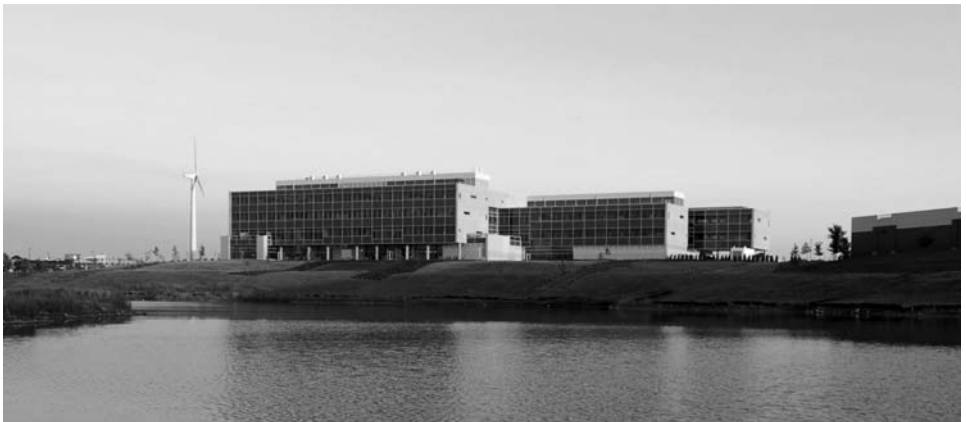
Figure 8.1 GRE headquarters—a 200-kW wind turbine provides renewable energy to the building.
