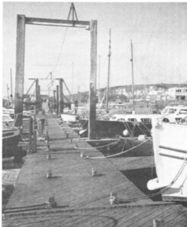
4 A large marina with full facilities for cruising boats and ample car parking. 5 shows a similar scene at eye level, with floating pontoons, locating piles, mooring bollards and overhead services. Installations on this scale need sensitive and strong handling if they are to be integrated with the landscape
