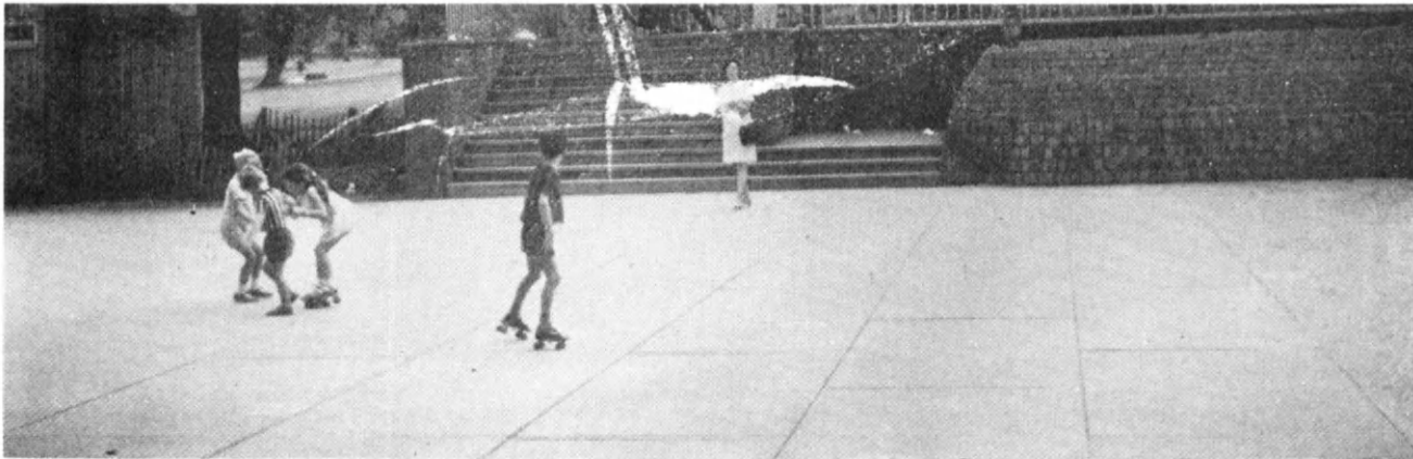
2 Butt jointed compressed asbestos cement sheeting as surfacing for a roller skating area
