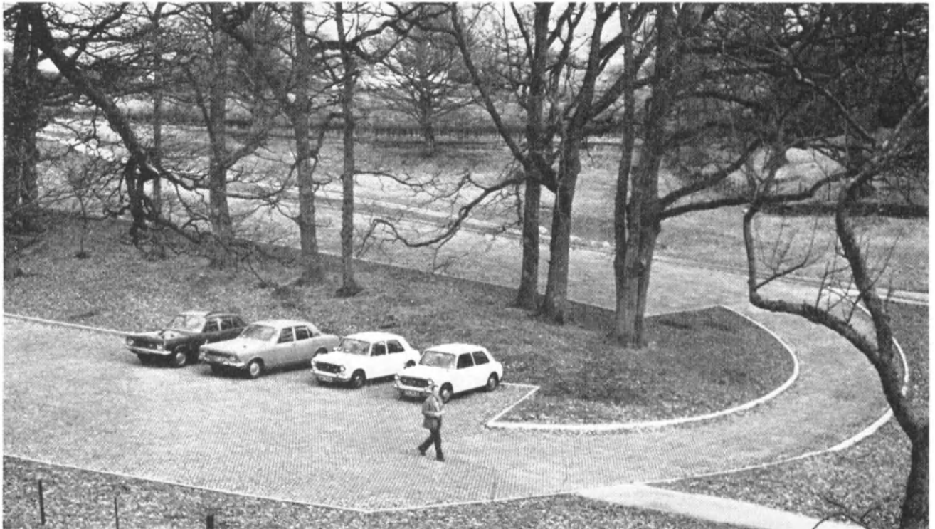
8 Firepath pots give fairly unobtrusive paved area. Grass can be grown in holes in pots. Suitable for light traffic
