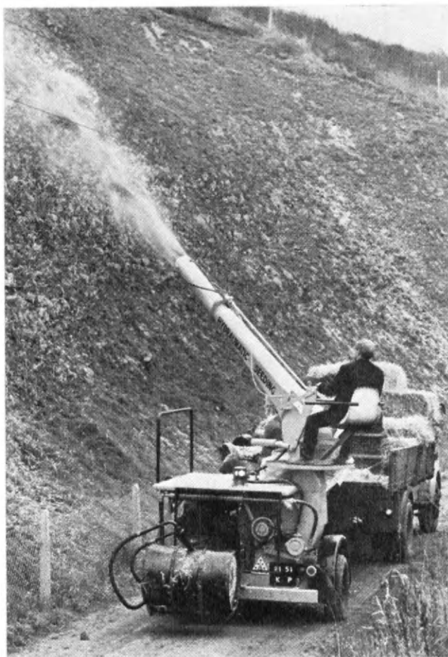
20 Hydra seeding bank too steep for conventional seeding techniques. In this illustration, seeded surface is being sprayed with a mulch of chopped straw
