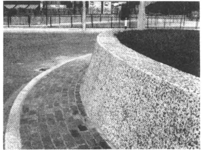
3 In situ retaining wall, Elephant and Castle, London
