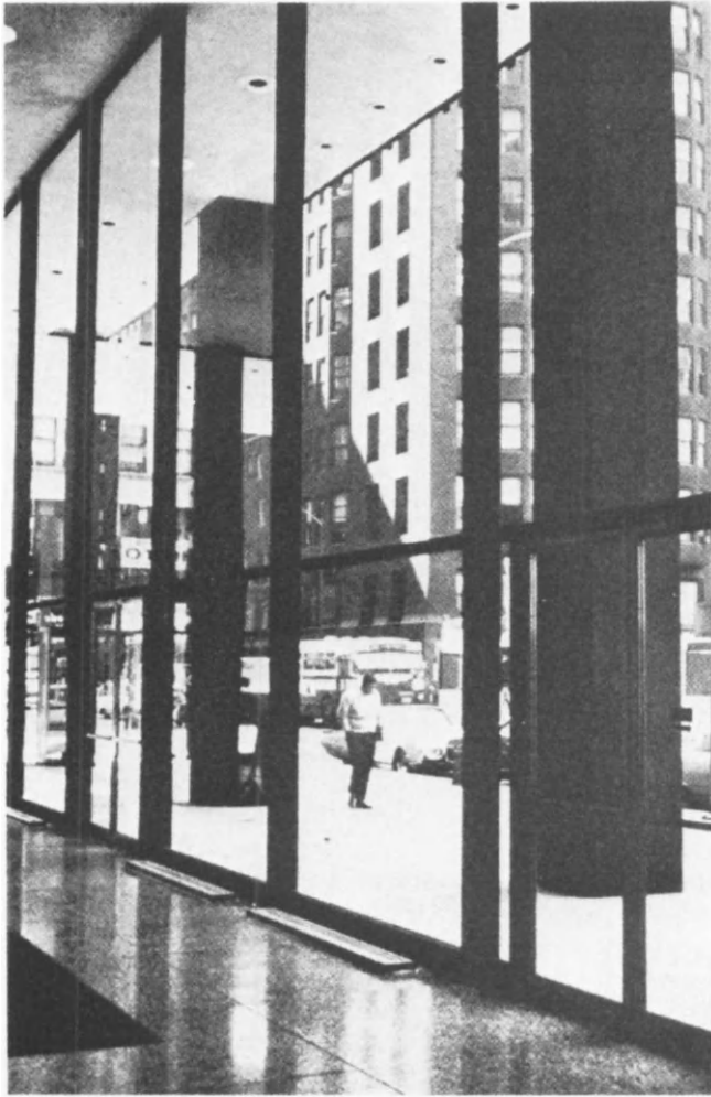
6 Monadnock building from Federal Centre, Chicago. Brick building radiates heat at night. Mies' glass façade, magnificent from within, is less effective climatically outside
