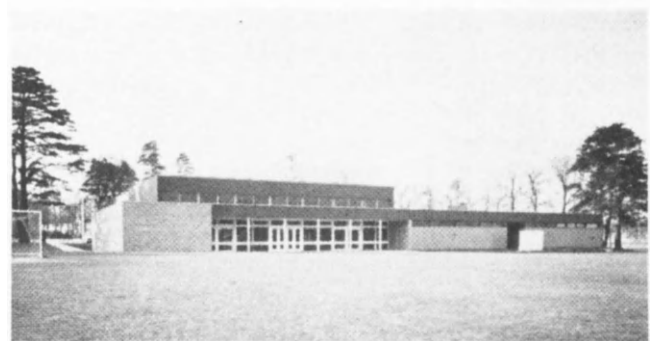
1 Part of Bracknell Sports Centre, Berks. Changing rooms on right serve outdoor pitches and running track
