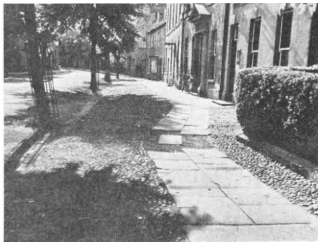
2 Small free path of stone flags set in a buffer zone of cobbles bordered by a small paved gutter
