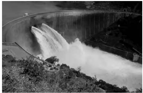
Figure 15.12 Wall of the Kariba Dam. Photograph reprinted with permission from Mike Main
