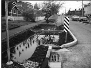
Figure B-Curb Extension Example
