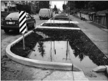
Figure C-Full Block Curb Shift Example
