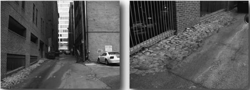
Picture 2: 12th Street Existing Conditions
