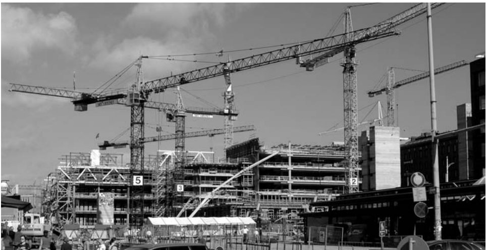
Figure 17.1 Construction of the Kamppi Centre building complex, Helsinki, Finland
