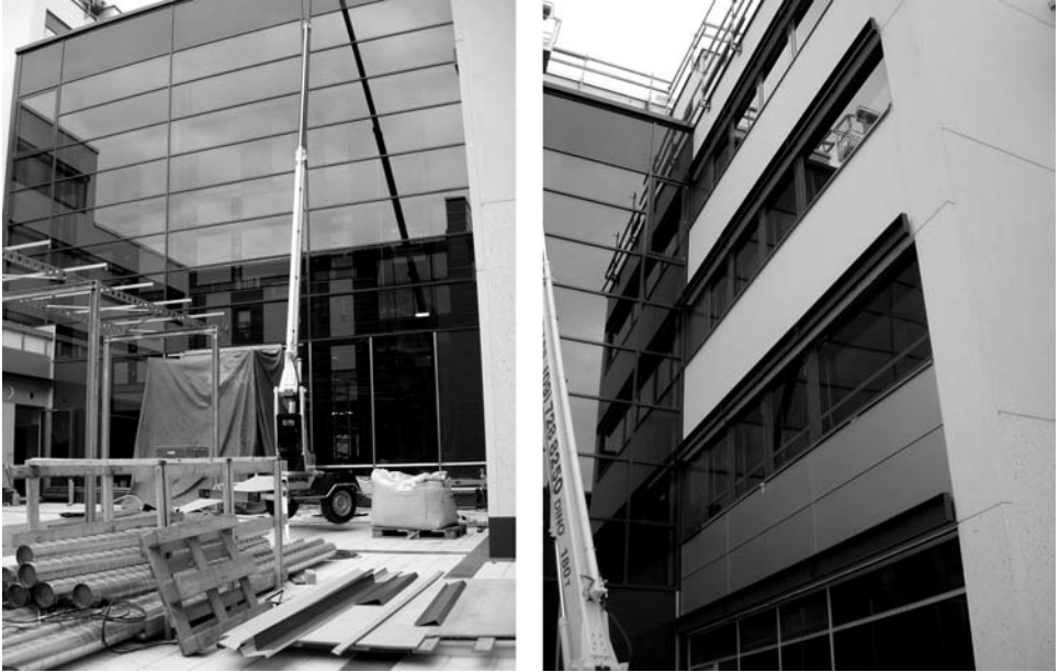
Figure 15.2 Opus 3: Opus Business Park—joining corridor façade
