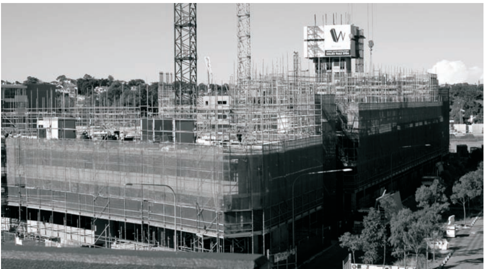
Figure 17.3 Victoria Park residential development—Form 302—in construction
