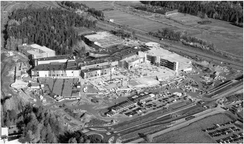
Figure 17.8 Skanssi retail centre—in construction
