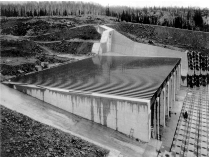
**Figure 18.40.** Debris-flow grill, Furano River, Japan.
