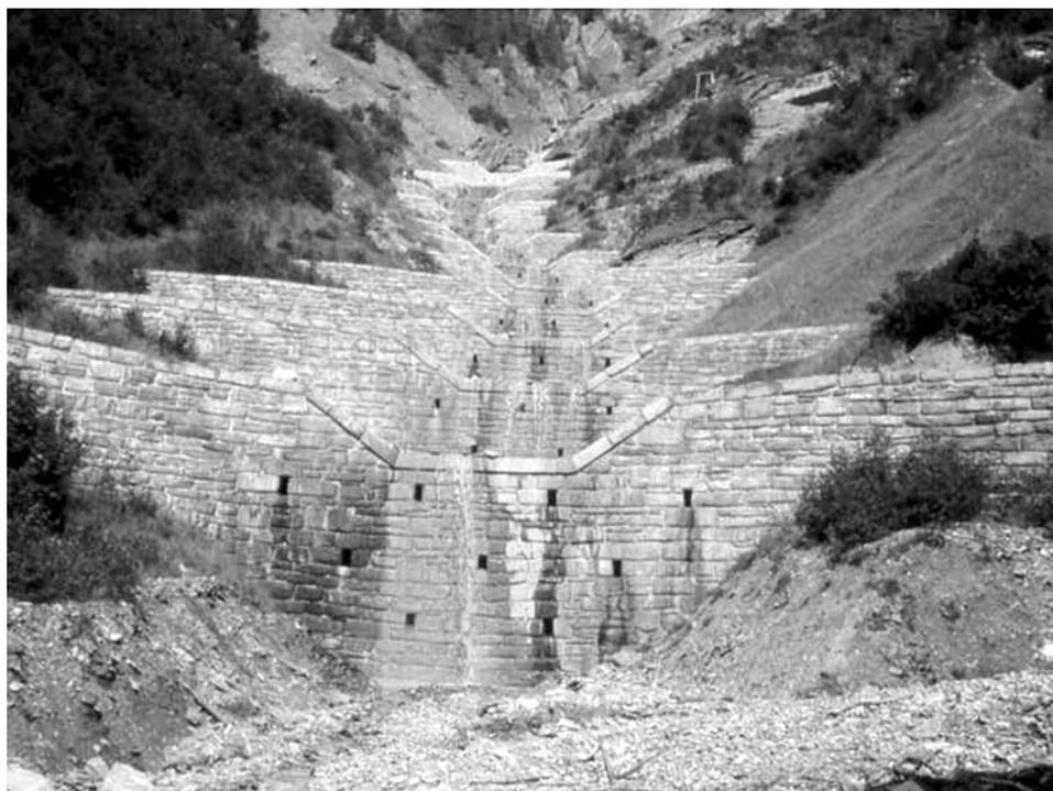
**Figure 18.6.** Transverse toe slope stabilization, Bretterwandbach, Tyrol, Austria.
