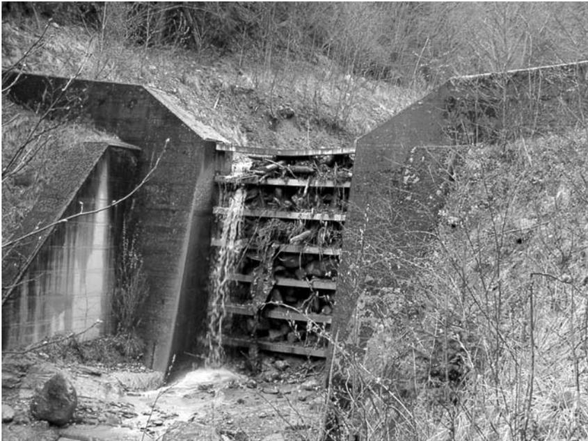
**Figure 18.28.** Beam barrier, Truebenbach, Carinthia, Austria.
