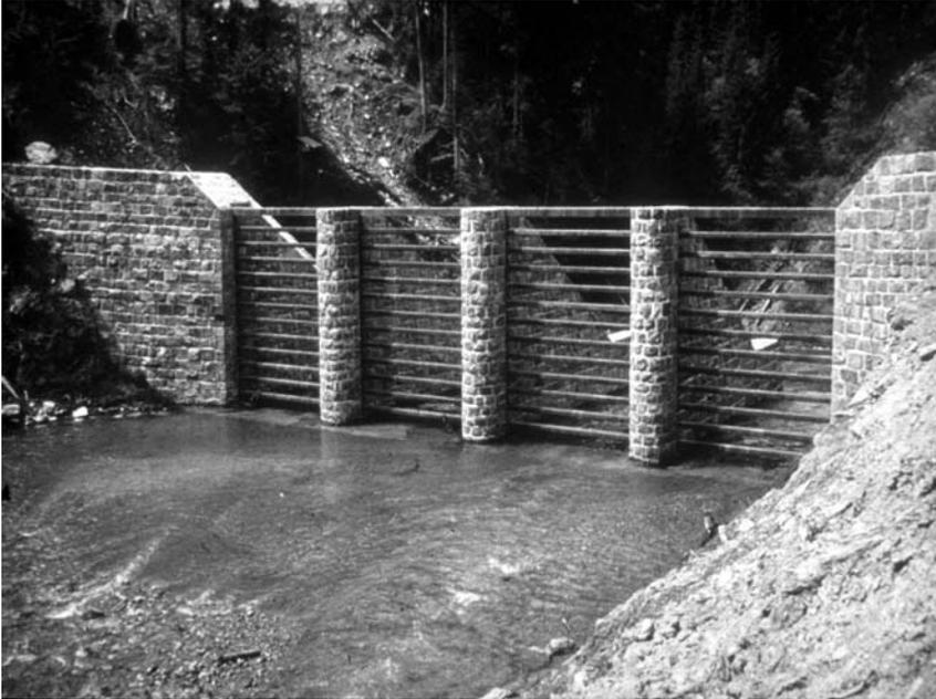
**Figure 18.25.** Sectional barrier with fins and beams, Maerzenbach, Tyrol, Austria.
