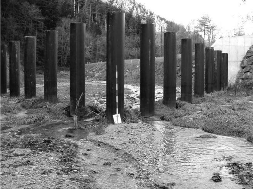
**Figure 18.27.** Sectional barrier with piles, Waldbach, Styria, Austria.
