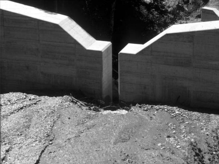
**Figure 18.23.** Slit barrier with vertical slits, Zinkenbach, Salzburg, Austria.
