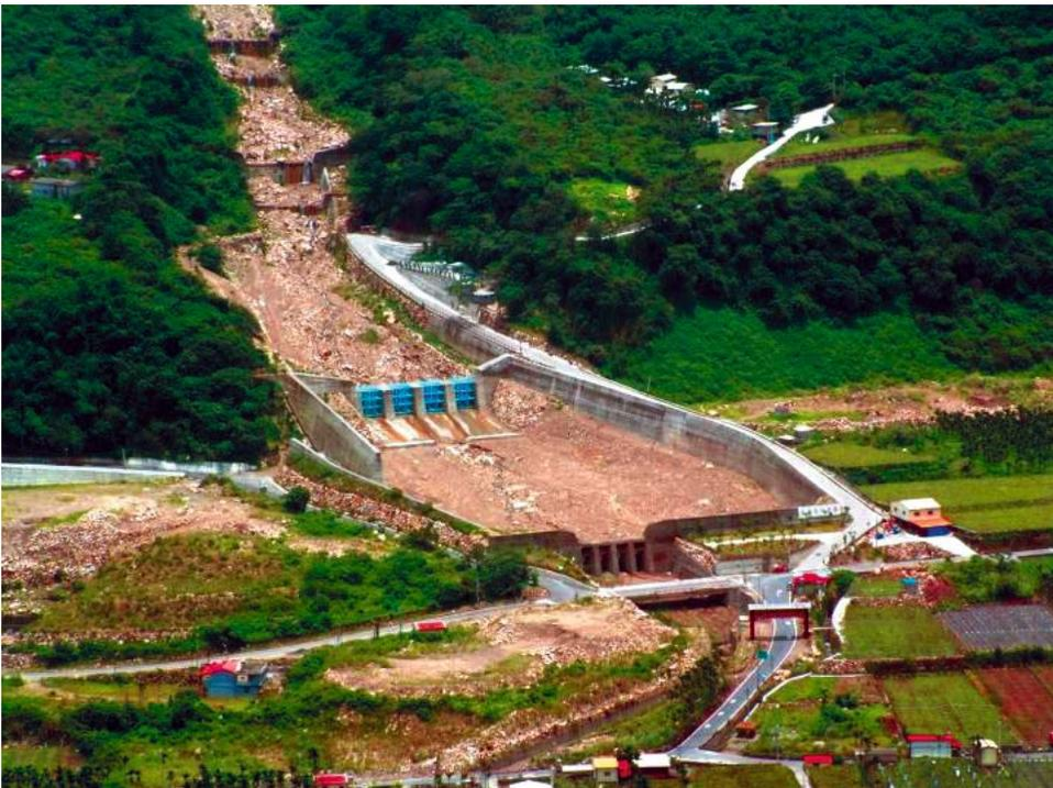
**Figure 21.17.** Debris-flow structural countermeasures, such as Sabo dams, debris barriers, and debris basins, at Fengqiu in the Chenyoulan stream watershed. The photo shows a relatively big debris basin having a designed capacity of 80,000 m<sup>3</sup>. It was built in 1999, and later divided by a grid-type slit dam (as shown in blue color) in 2000. Photo: Professor C.C. Wu).
