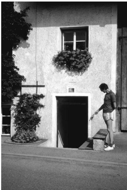
**Figure 3.4.** The side entrance to the library at Inzing is below ground, the level having been built up by earlier debris-flow depositions.
