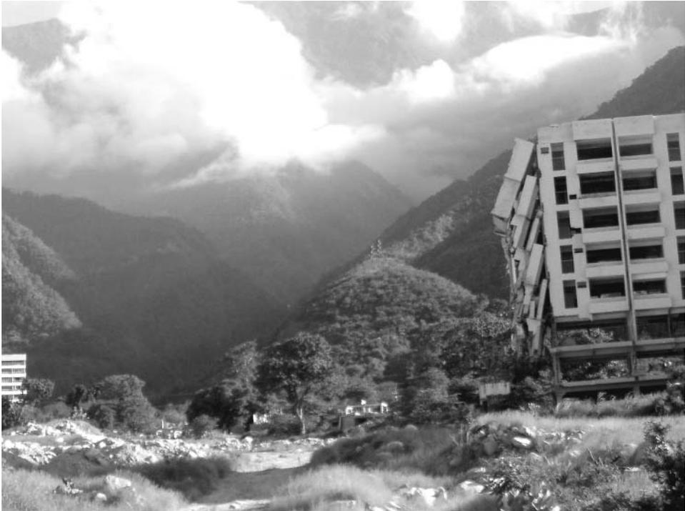
**Figure 1.1.** Damaged buildings on the Caraballeda Fan in the Vargas Province, Venezuela, caused by a series of debris flows descending the slopes of the El Avila range (background) in December, 1999.
