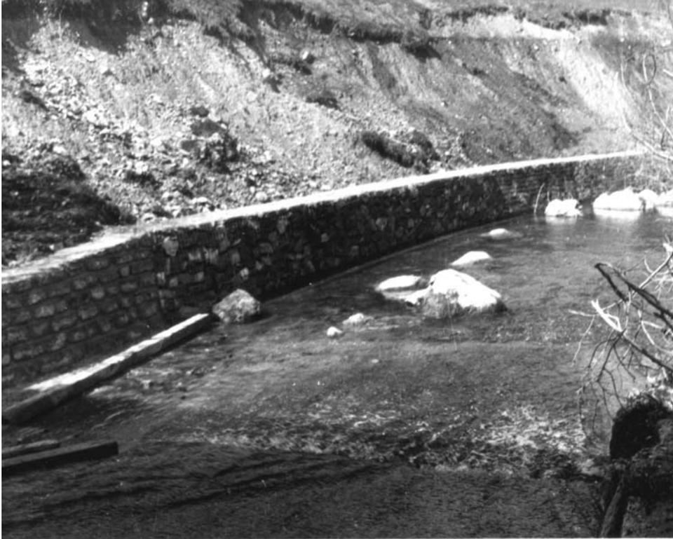
**Figure 18.7.** Longitudinal toe slope stabilization, Eugenchach, Austria.
