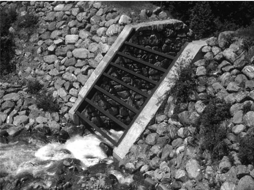
**Figure 18.30.** Beam barrier, Istalanzbach, Tyrol, Austria.
