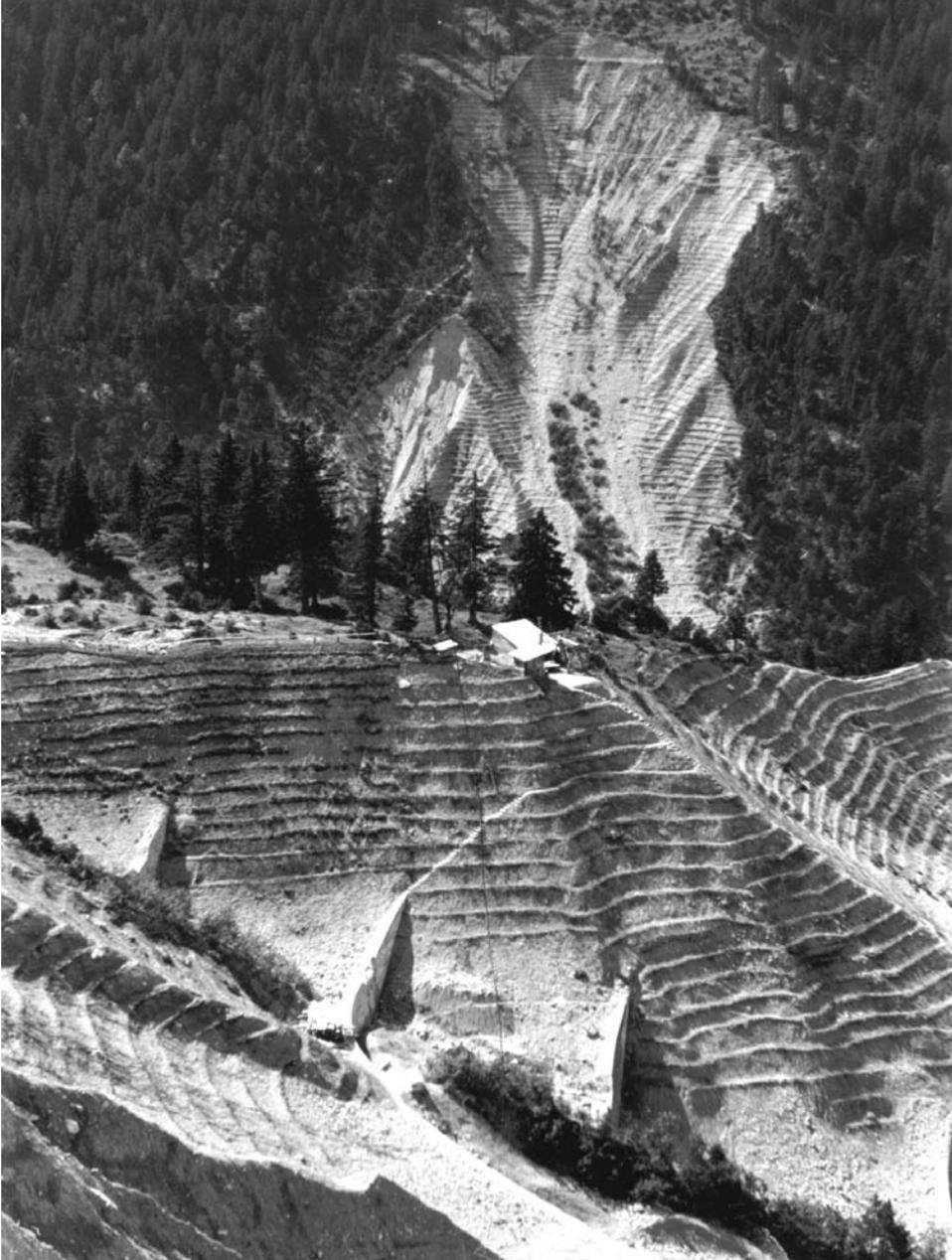
**Figure 18.5.** Slope stabilization at Filpittertobel in 1898, Vorarlberg, Austria.
