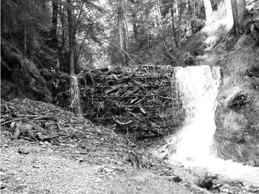
**Figure 18.35.** Net barrier, Gleiersbach, Tyrol, Austria.
