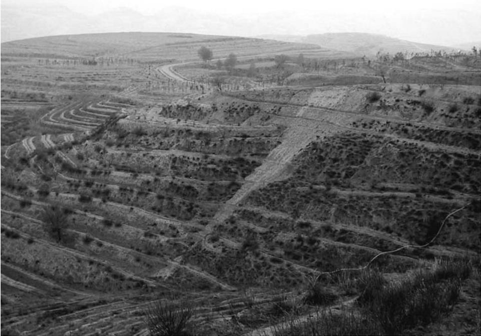
**Figure 16.7.** A landslide initiating on a constructed agricultural terrace in the Loess Plateau, Shanxi Province, China.
