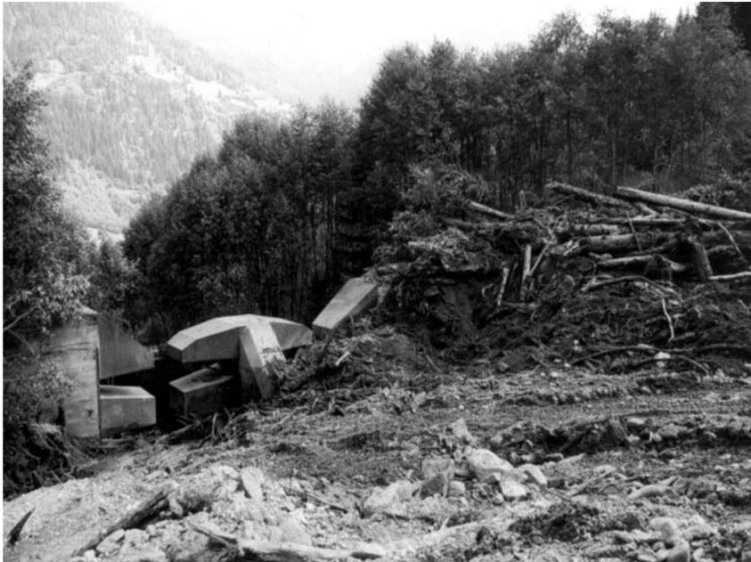
**Figure 18.32.** Cross-slit barrier in 2000 after a debris flow, Luggauerbach, Salzburg, Austria.
