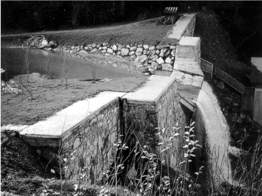
**Figure 18.11.** Downstream wing walls, Wagrain Ache, Salzburg, Austria.
