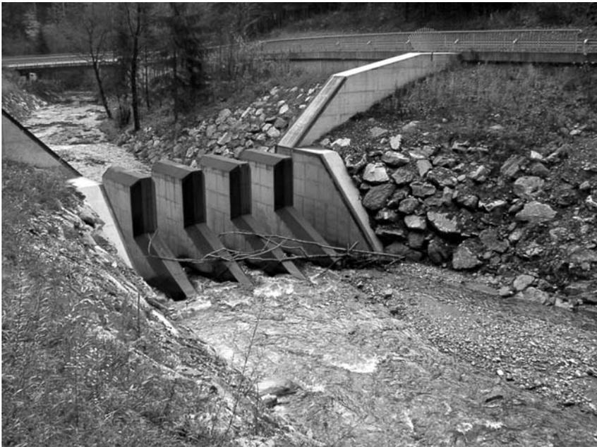
**Figure 18.26.** Sectional barrier with fins, Sallabach, Styria, Austria.
