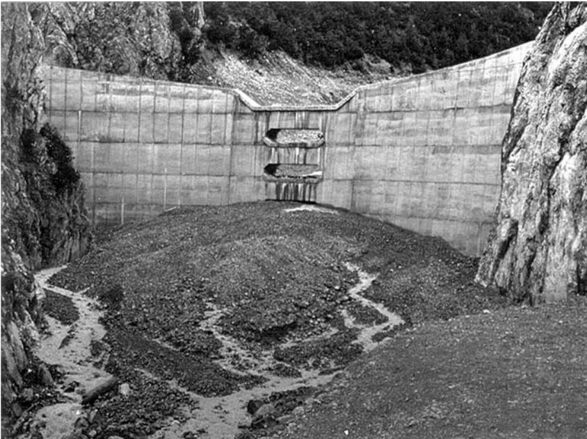
**Figure 18.24.** Slit barrier with horizontal slits, Schnannerbach, Tyrol, Austria.
