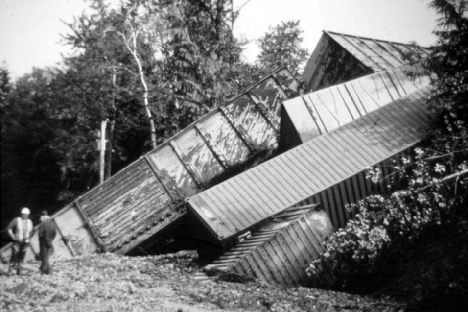
**Figure 1.2.** Freight train derailed by the direct impact of a small debris flow in high mountains. Although infrequent, such accidents cause property damage and could result in loss of life.
