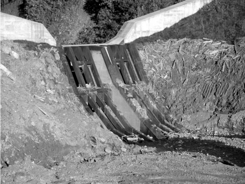
**Figure 18.29.** Sectional rake barrier, Loehnersbach, Salzburg, Austria.
