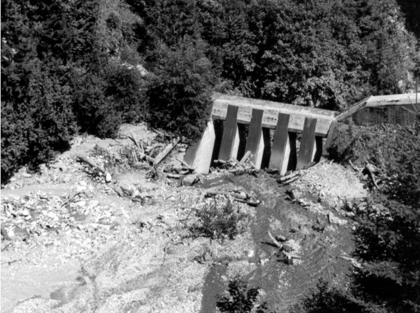
**Figure 18.37.** Sectional barrier with fins in 2000 after a debris-flow event, Luggauerbach, Salzburg, Austria.
