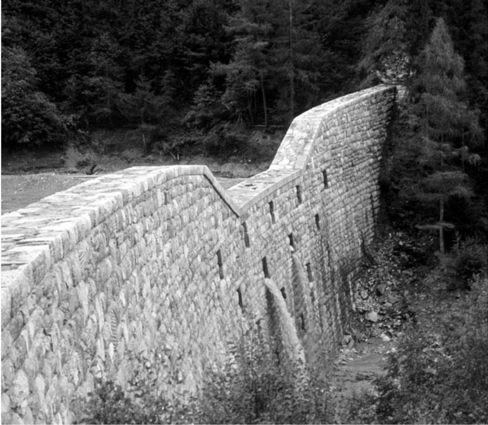
**Figure 18.19.** Small slot barrier, Koednitzbach, Tyrol, Austria.
