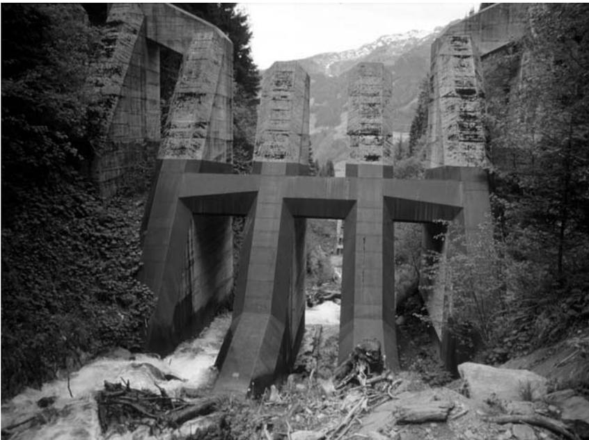
**Figure 18.38.** Sectional barrier with fins, Rastelzenbach, Salzburg, Austria.
