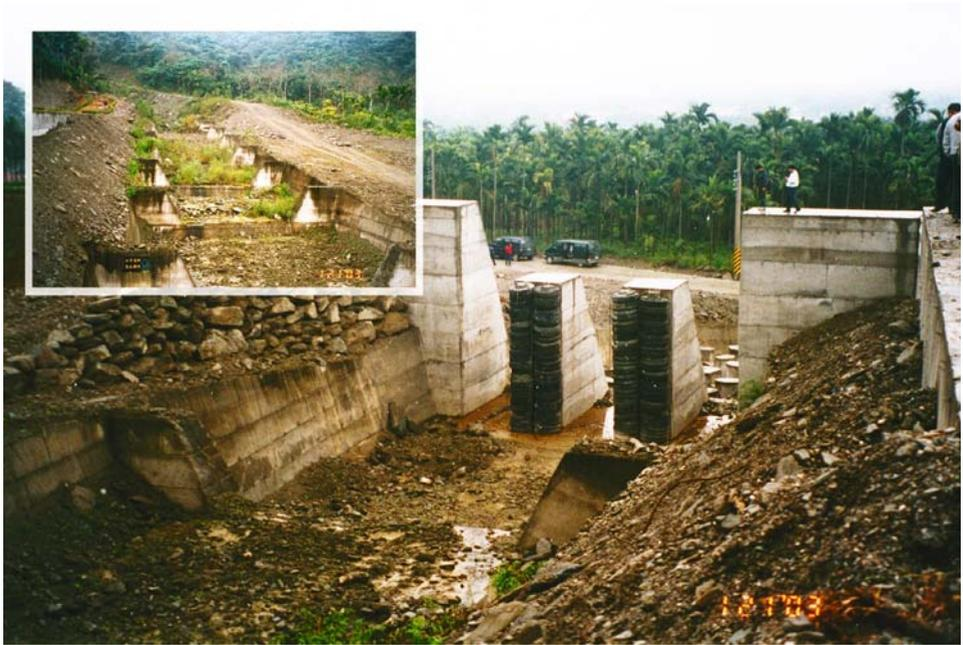
**Figure 21.18.** A slit dam built at the outlet of a debris-flow-prone stream at Jianqing in Hualien County. Note the use of tires on the upstream face of the slit dam to reduce the debris-flow impact. The photo inset shows a series of check dams constructed to stabilize the channel bed and banks along the stream channel upstream of the slit dam.
