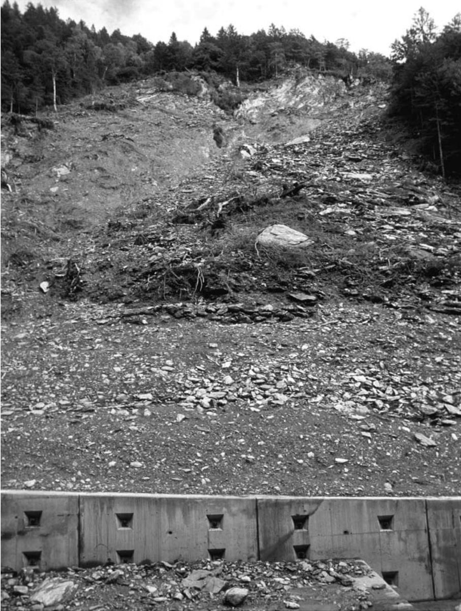
**Figure 18.14.** Anchored longitudinal structure, Kirchbachgraben, Carinthia, Austria.
