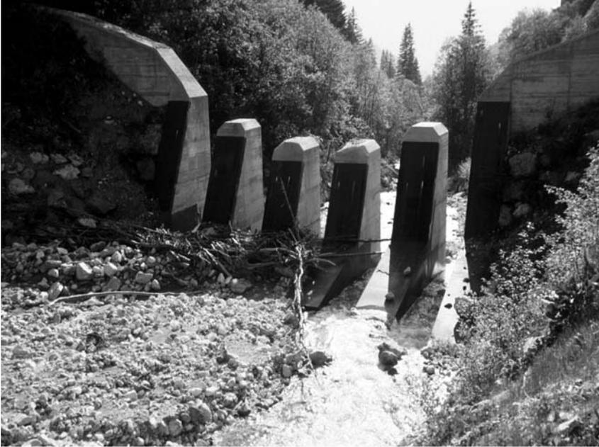
**Figure 18.39.** Sectional barrier with fins, Ellmaubach, Salzburg, Austria.
