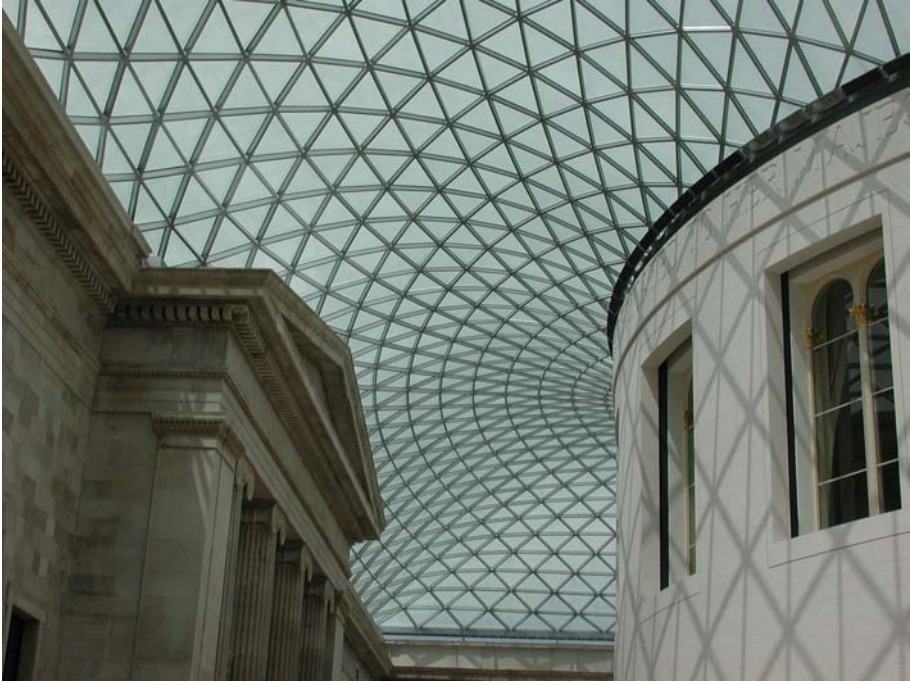
Figure 2 The roof of the British Museum courtyard, London, by Norman Foster. Non-repetitive construction is enabled by efficient numerically controlled fabrication, but design content remains fairly low, since the varied shapes of the roof panels, structural members, and joints are controlled by simple rules and a few parameter values.
