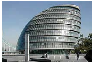
Figure 1 The GLA Building
