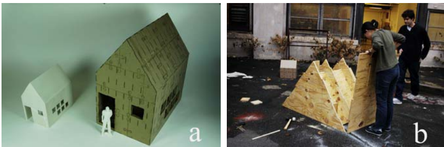
Figure 9 (a) 3D print and a model of cardboard sheets measuring 10" x 15" x 16", (b) student assembling a friction fit full scale plywood section at the roof
