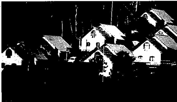
8. Multi-storey rented housing, Cavani, Mayotte.
