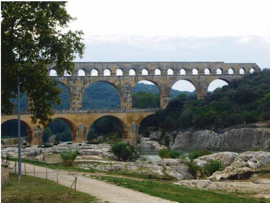
Fig. 8.1 Pont du Gard, a Roman aqueduct in the south of France built in 50 AD
