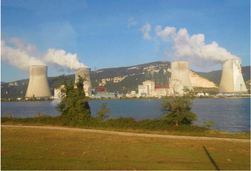
Fig. 6.3 The nuclear plant Cruas-Meysee (operating since 1983) on the bank of the river Rhône, France
