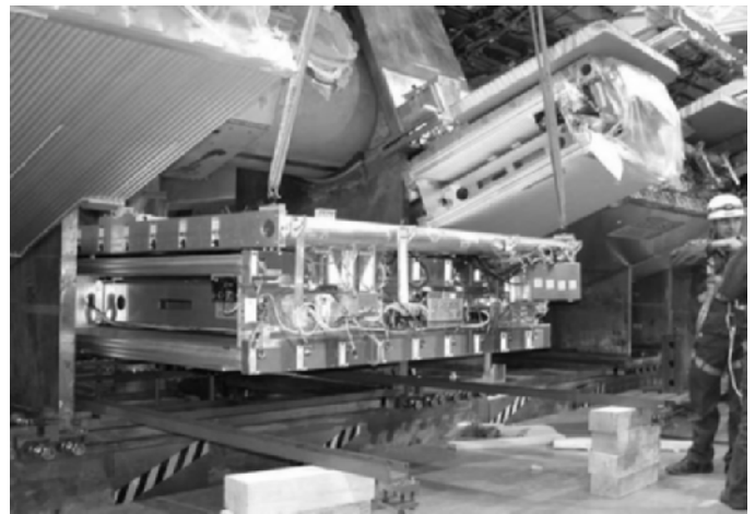
Fig. 9. Barrel muon chambers being installed.
