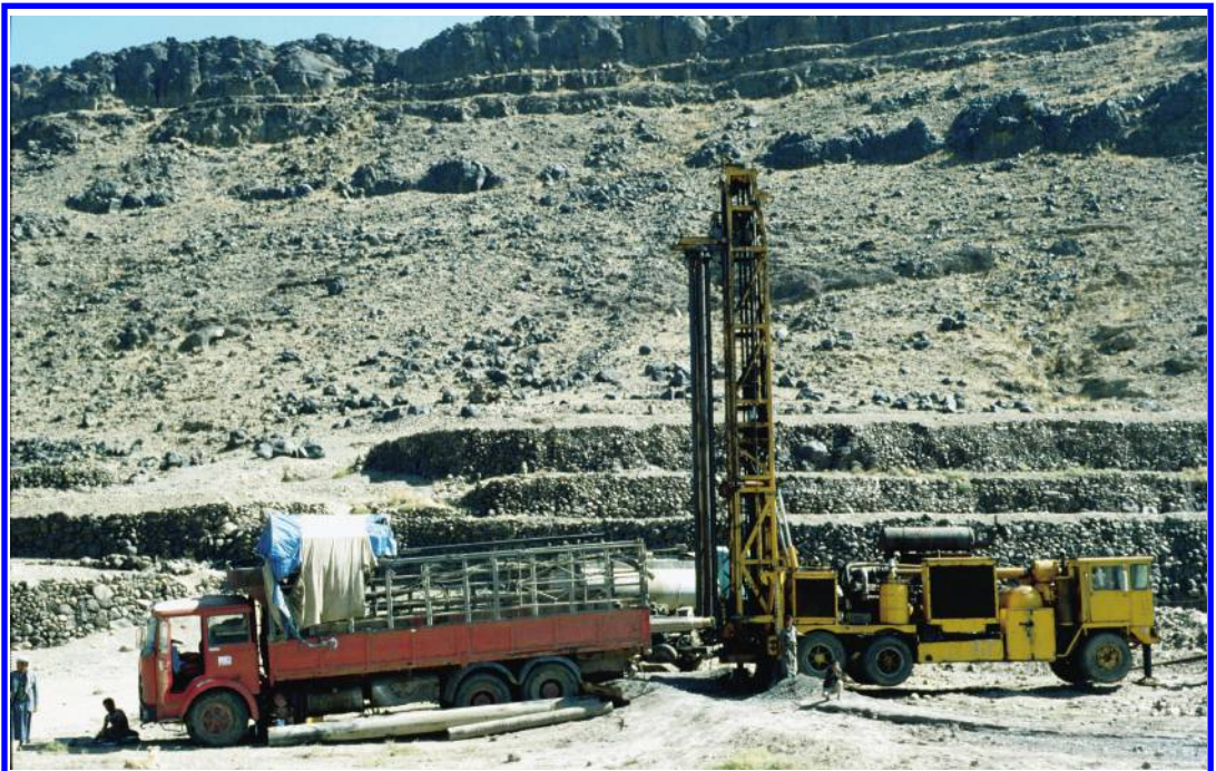
Figure 6.8. Direct (straight) circulation mud rotary drilling in the Sana'a Basin, Yemen.
