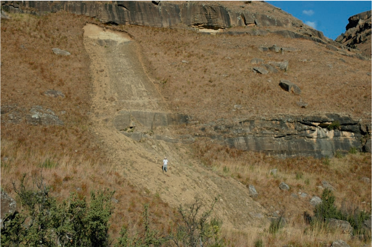
Fig. 14.7 Shallow landslides involving slope covers are common on the steep slopes below the main escarpment (Photo S. Grab)
