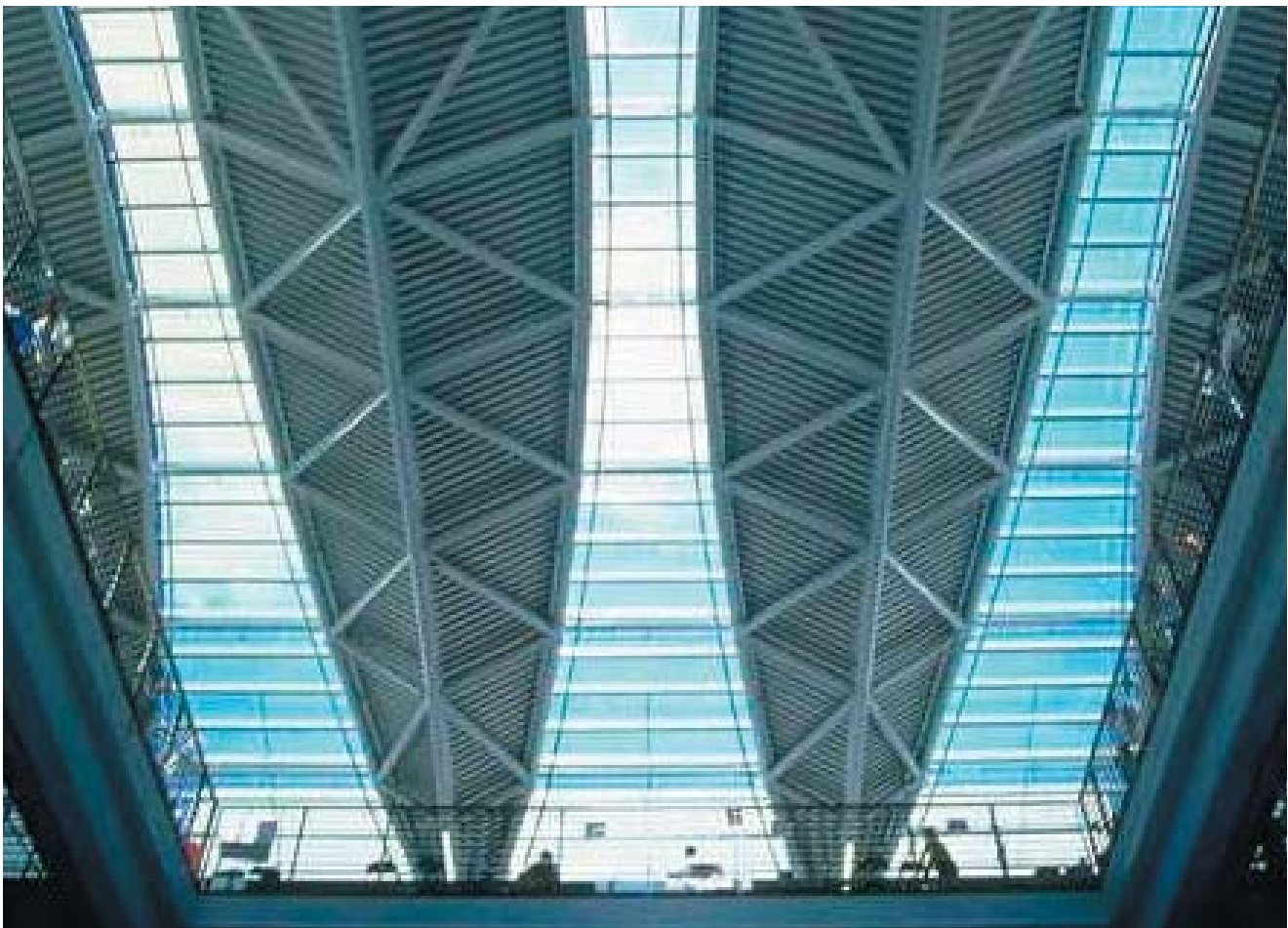
Fig 1.5 HACTL Terminal (Hong Kong Cargo Terminals Ltd) – On this project the automatic sprinkler system was incorporated into the tubular roof truss members in such a way that the sprinkler water served a dual purpose; that of controlling the fire size by normal sprinkler action and to remove heat from the structure. The combined effect was used to demonstrate that no passive fire resistance protection was required. © ARUP
