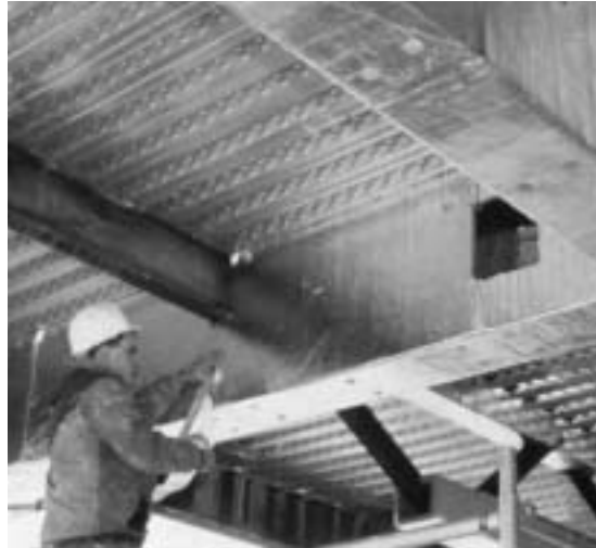
Fig A.3 Foil covered fibre board applied to beams © Rockwool Ltd
