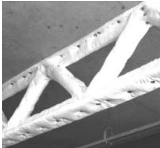
Fig A.4 Pin-fixed blanket applied to truss © Unifrax Corporation
