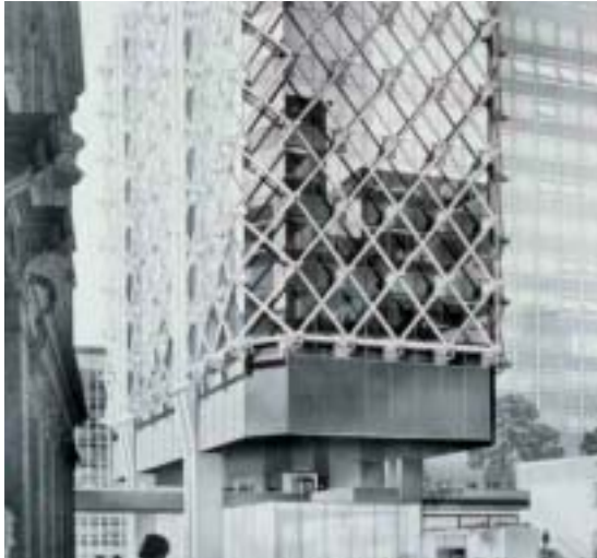
Fig 1.4 Bush Lane House – Water cooling of the external structure allowed the use of exposed steel without passive fire protection.
