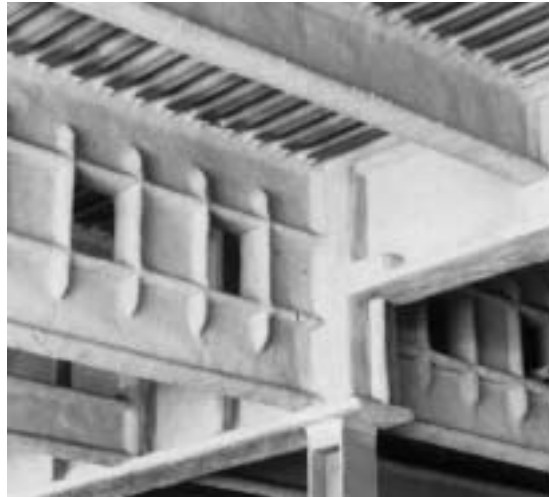
Fig A.1 Sprayed protection applied to complex beam detail © Cafco International
