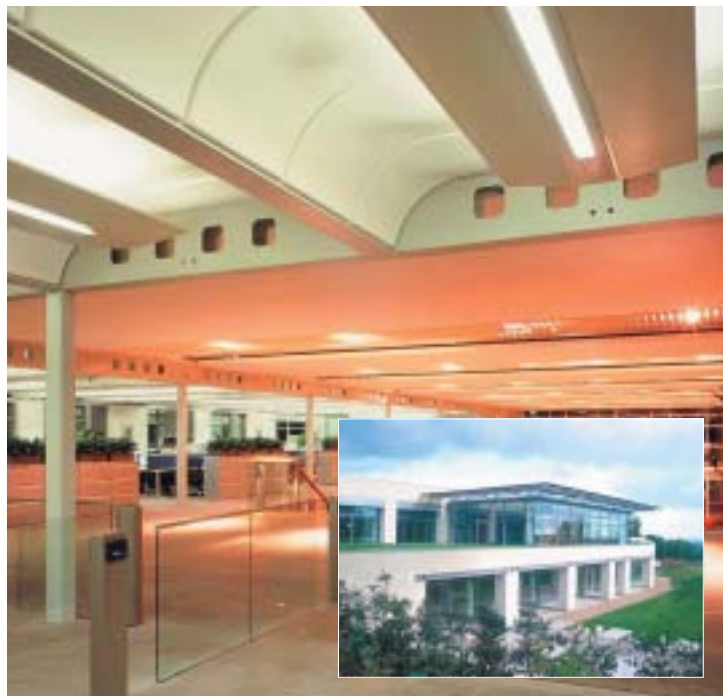
Fig 1.3 Wessex Water Headquarters – This project is an example of the integration of concrete and steel construction to support very low energy design solutions and the integration of services. Exposed structural steel was an integrated part of this solution. © Buro Happold/Mandy Reynolds
