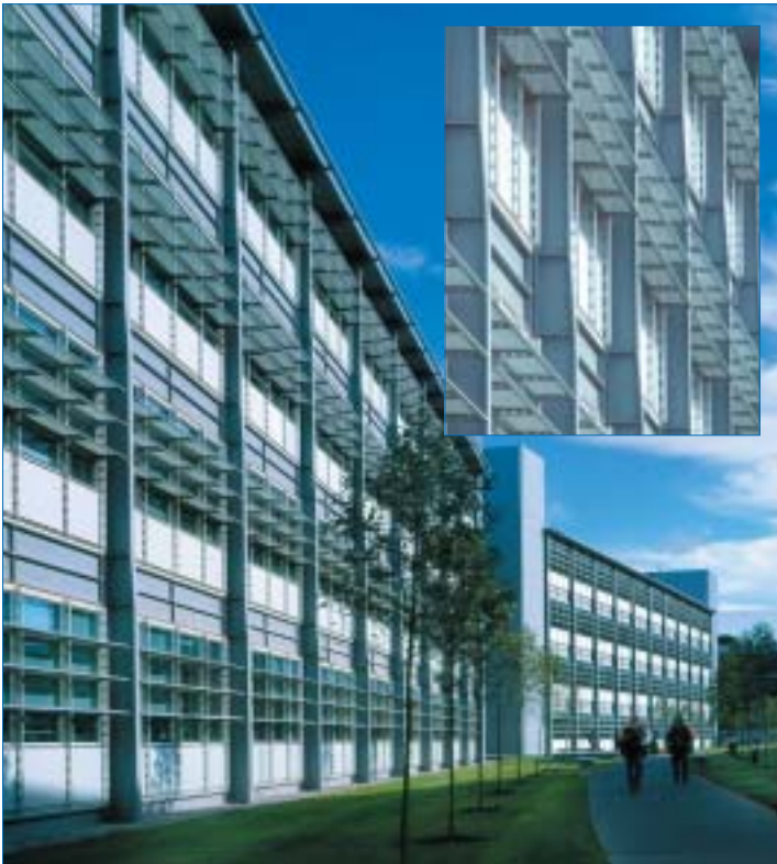
Fig 3.1 DSS Longbenton – external unprotected steelwork which is an integrated part of the architectural solution for the elevations
