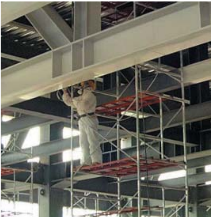
Fig A.6 Thin film intumescent coating being applied
