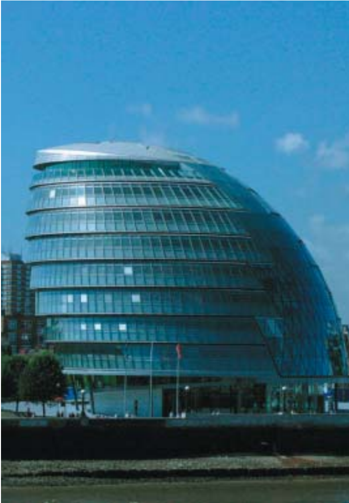
Fig 1.1 Greater London Assembly Building, London – This project used fire engineering principles to assess the fire resistance requirements for the structure as a whole, instead of relying entirely on the tabulated fire resistance values given in Approved Document B 1.4 © ARUP
