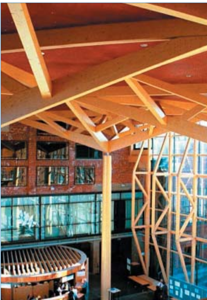
Fig 6.8 Sibelius Hall, Lahti Finland – view of atrium, ticketing and enquiries desks from gallery – note integrated restored brick building to rear and vertical wind girders supporting glazing to right – these incorporate embedded fire resistant flitched steelwork connections.
