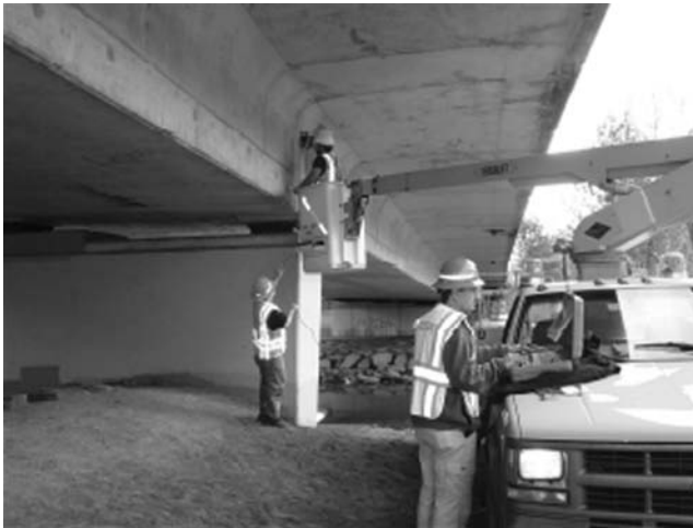
FIGURE 4.26 Impact-echo field experiment. (Courtesy of Olson Engineering, Inc.)
