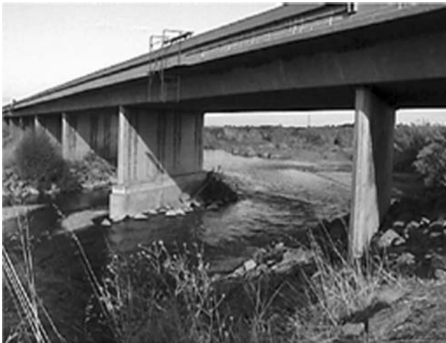
FIGURE 1.30 The Stony Creek Bridge, Glenn County, CA. (Courtesy of CRC Press.)
