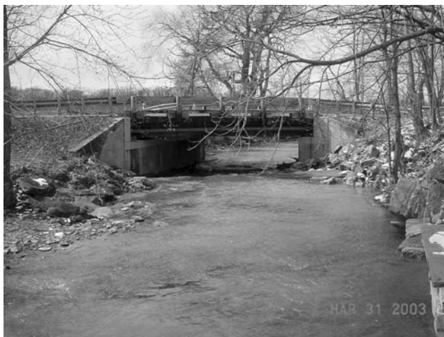
FIGURE 9.22 A conventional bridge. (Courtesy of New York State Department of Transportation.)
