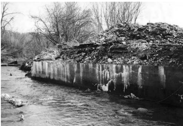
FIGURE 6.44 Removed old superstructure. (Courtesy of New York State Department of Transportation.)
