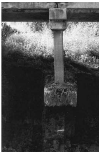
Excavating under foundation
