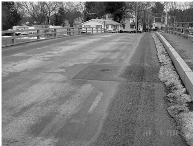
FIGURE 6.30 South Board Street Bridge—Wellsville, NY.
