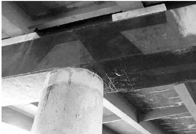
FIGURE 7.65 FRP retrofits. (Courtesy of New York State Department of Transportation.)
