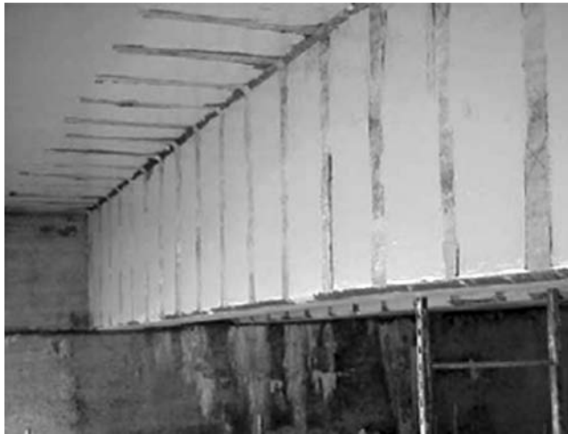
FIGURE 7.70 Retrofitting FRP laminates. (Courtesy of New York State Department of Transportation.)
