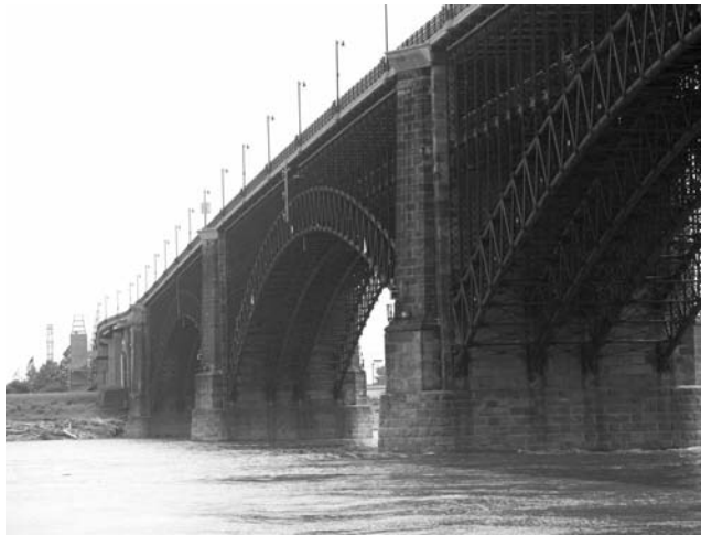
FIGURE 9.23 Complex bridge structural systems need special inspection procedures.
