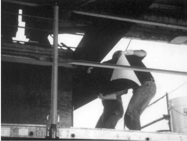
FIGURE 7.32 Laying FRP layers. (Courtesy of New York State Department of Transportation.)
