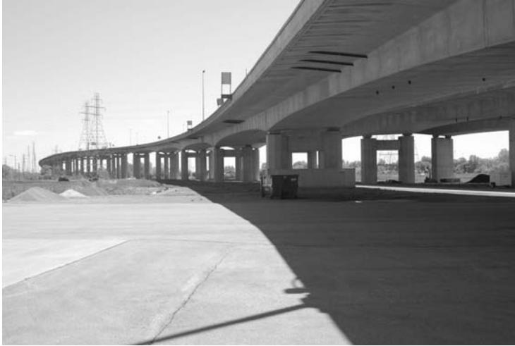
FIGURE 4.1 Zilwaukee Bridge: a box girder PSC system in Michigan.
