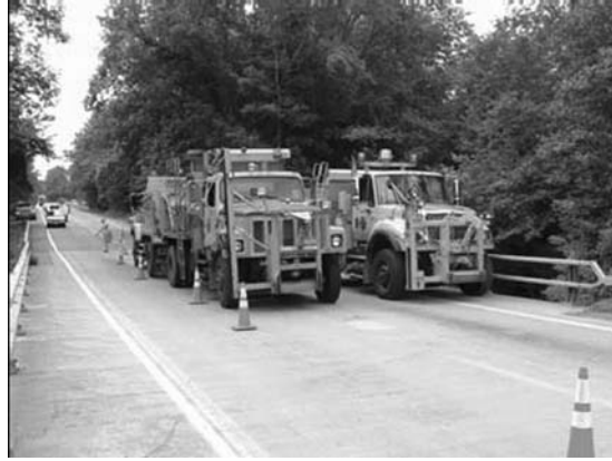
FIGURE 8.53 Typical load test. (Courtesy of New York State Department of Transportation.)
