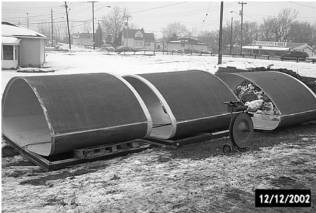
FIGURE 7.59 FRP culvert liners before installation. (Courtesy of Erie County DPW of New York State.)
