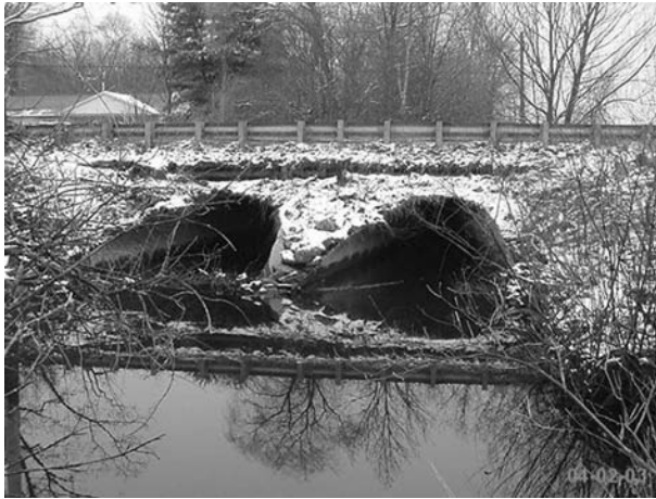
FIGURE 9.19 Nonbridge structure. (Courtesy of New York State Department of Transportation.)
