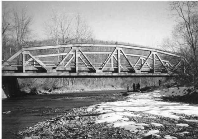
FIGURE 6.65 Effect of deck replacement on member total forces. (Courtesy of New York State Department of Transportation.)
