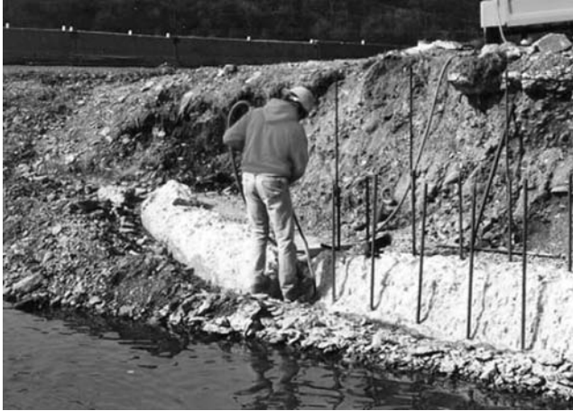
FIGURE 6.45 Construction of abutments. (Courtesy of New York State Department of Transportation.)
