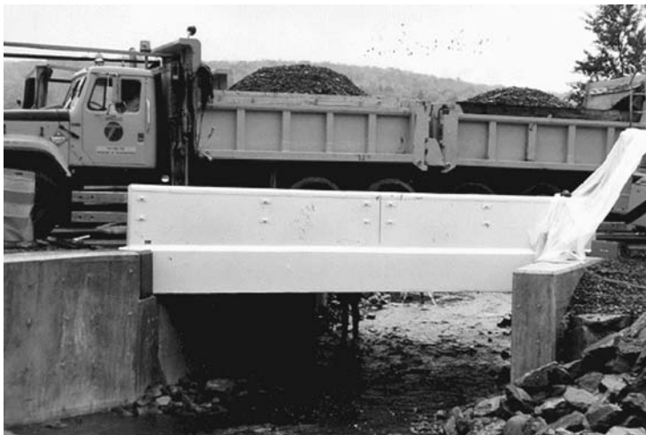
FIGURE 8.9 Truck loading process. (Courtesy of New York State Department of Transportation.)
