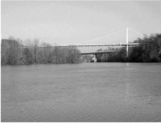
FIGURE 5.24 Photo showing suspension bridge cables.
