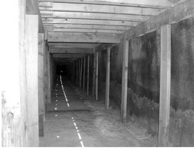
FIGURE 4.31 Interior view of the girder area. (Reprinted from ASNT Publication.)
