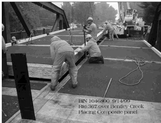
FIGURE 6.57 Placing FRP deck. (Courtesy of New York State Department of Transportation.)
