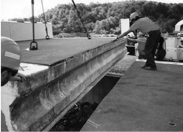
FIGURE 6.50 Final construction steps. (Courtesy of New York State Department of Transportation.)
