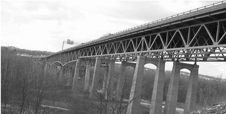
FIGURE 5.34 Patroon Island Bridge. (Courtesy of New York State Department of Transportation.)
