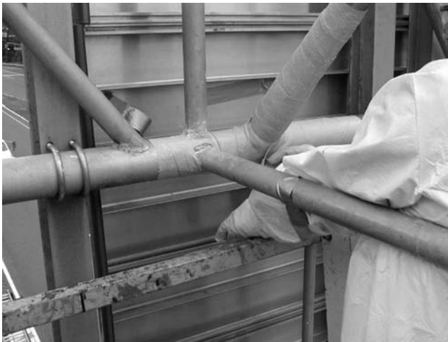
FIGURE 7.57 Finished FRP retrofit. (Courtesy of New York State Department of Transportation.)
