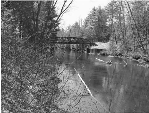
FIGURE 1.19 Sheetpiling. (Courtesy of New York State Department of Transportation.)
