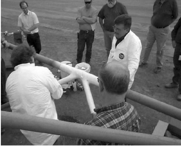
FIGURE 7.56 Applying FRP retrofit. (Courtesy of New York State Department of Transportation.)
