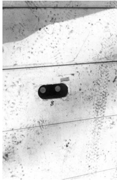
FIGURE 6.27 FRP deck during construction to show the connection with the girders.
