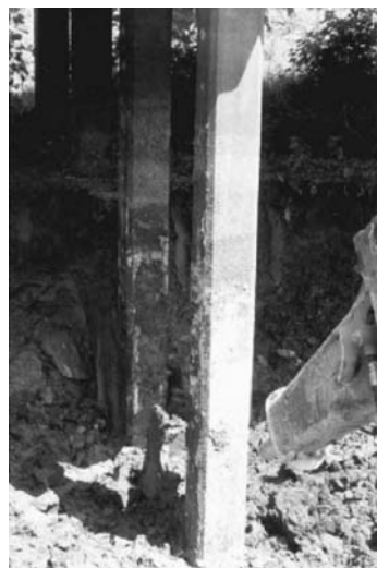
Excavating around piles
