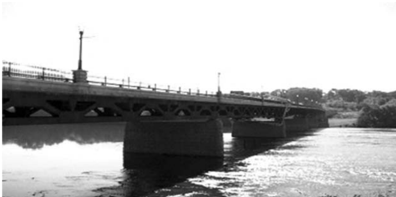
FIGURE 8.41 Court Street Bridge. (Courtesy of New York State Department of Transportation.)
