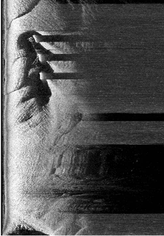
FIGURE 1.54 Scour of river bottom as shown by dual sonar monitoring. (From Stock, T., Use of a hummingbird model 997 side scan sonar as a bridge inspection tool, Report to Wisconsin Division of FHWA, 2008.)
