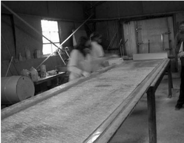
FIGURE 6.18 FRP bridge deck manufacturing: open mold—I. (Courtesy of Jerome O'Connor.)
