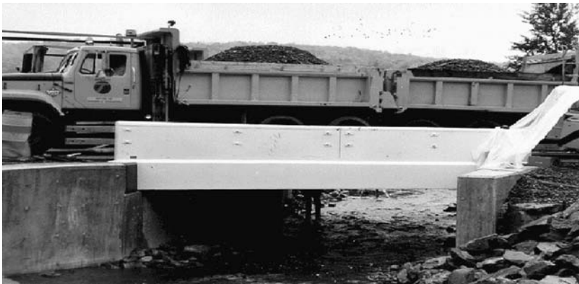
FIGURE 6.53 Subsequent load tests. (Courtesy of New York State Department of Transportation.)
