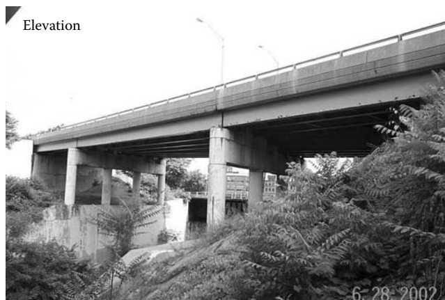
FIGURE 9.21 A conventional bridge. (Courtesy of New York State Department of Transportation.)
