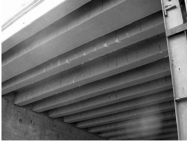
FIGURE 7.71 Retrofitted beams. (Courtesy of New York State Department of Transportation.)
