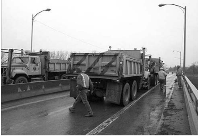
FIGURE 7.67 Load test of FRP retrofits. (Courtesy of New York State Department of Transportation.)
