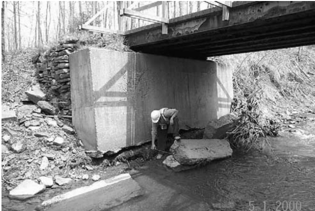
FIGURE 8.34 Potential brittle behavior during a load test: foundation problem. (Courtesy of New York State Department of Transportation.)
