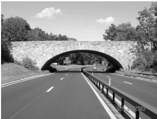
FIGURE 9.20 Highway bridge. (Courtesy of New York State Department of Transportation.)
