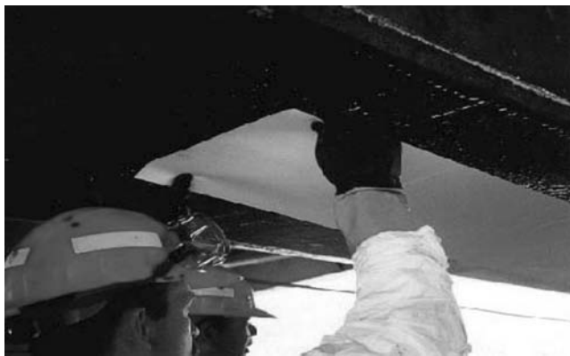
FIGURE 7.66 Installation of laminates. (Courtesy of New York State Department of Transportation.)
