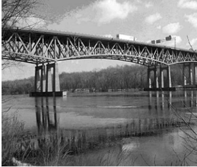
FIGURE 5.10 Patroon Island Bridge. (Courtesy of New York State Department of Transportation.)
