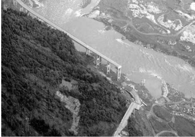
FIGURE 2.4 Seismic failure of curved bridge. (Courtesy of MCEER, University of Buffalo.)
