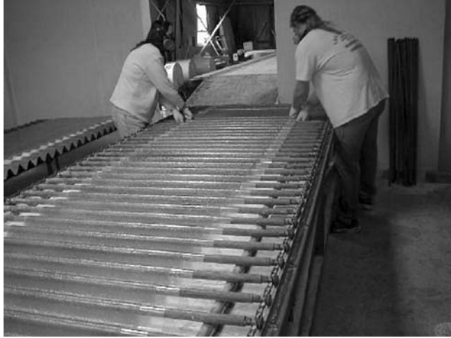
FIGURE 6.19 FRP bridge deck manufacturing: open mold—2. (Courtesy of Jerome O'Connor.)
