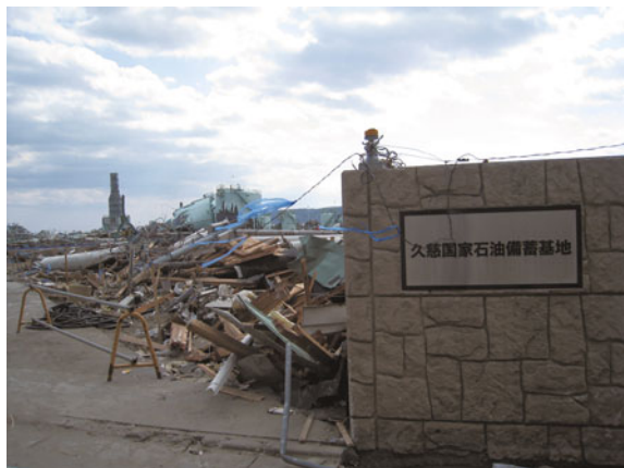
Fig. 4 National oil storage station in Kuji City, Iwate Prefecture
