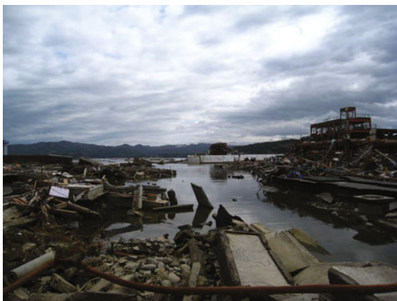
Fig. 9 Damaged port in the port area of Minami-sanriku
