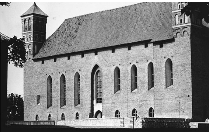
The pointed arches of the doors and windows of the bishop's palace at Lidzbark are typical of the early Polish brick gothic style of architecture. Copernicus lived in this palace from 1503 to 1510 while assisting his uncle, Bishop Lucas Watzenrode.
