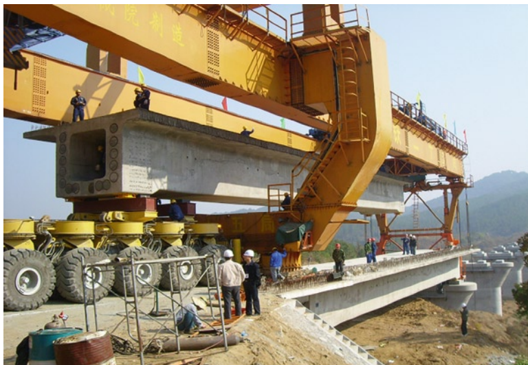
Fig. 12.4 Modern bridge construction equipment
