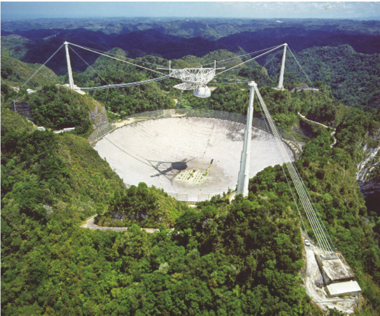
Fig. 1.19. With a diameter of 305 m, the Arecibo telescope in Puerto Rico is the largest single-dish telescope in the world; it may also be known from the James Bond movie “Goldeneye”. The disadvantage of its construction is its lack of steerability. Tracking of sources is only possible within narrow limits by moving the secondary mirror
