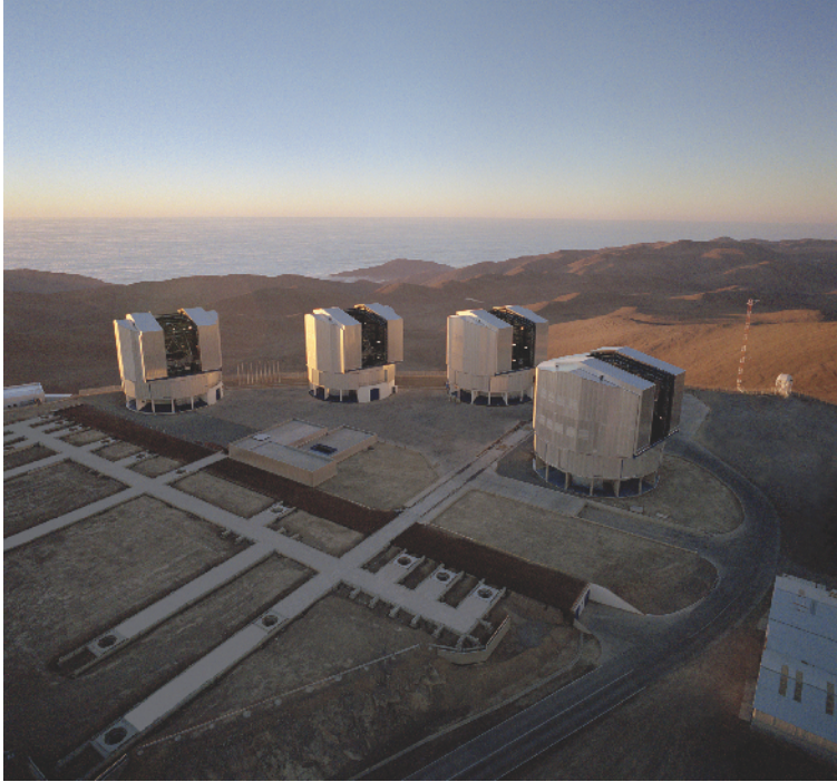
Fig. 1.31. The Paranal Observatory after completion of the domes for the four VLT unit telescopes. The tracks seen in the foreground were installed for additional smaller telescopes that are now jointly used with the VLT unit telescopes for interferometric observations in the NIR
