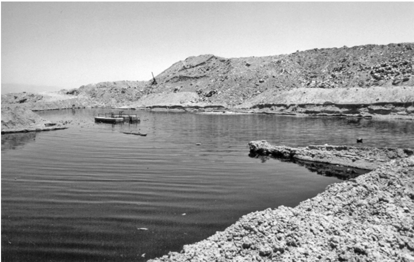
Fig. 11-1 Highly contaminated leachate pond (1.5 hectare, 180 000 m 3 ) in front of the Tehran Central Landfill, Iran (Körtel et al., 2003)
