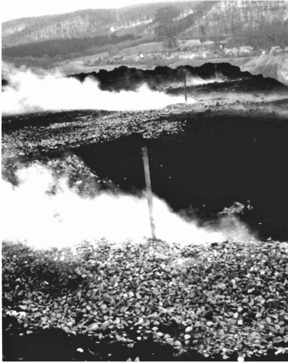
Fig. 11-24 Large bored piles filled with crushed stone to prevent heat accumulation by controlled heat dissipation. The flickering air and the plumes of steam indicate heat removal. Bright spots in the area of the steam plume are sulphur precipitations
