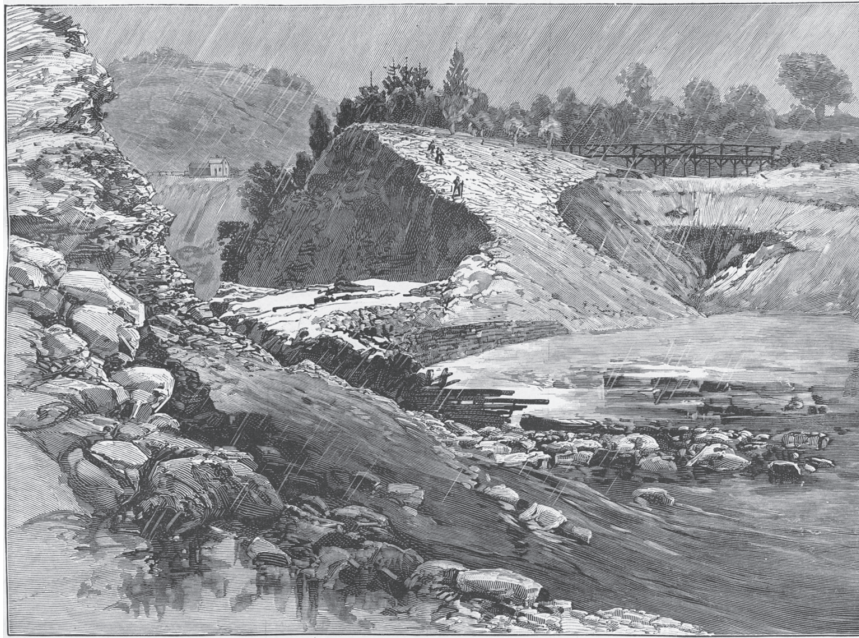
Fig. 7.3 The broken South Fork dam, as seen from inside the empty reservoir. The opening was about 130 m wide near the top; the spillway can be seen on the right just below the bridge. It took the flood surge roughly 53 min to reach Johnstown. Drawing by Schell and Hogan. (From Harper's Weekly , 1889.)
