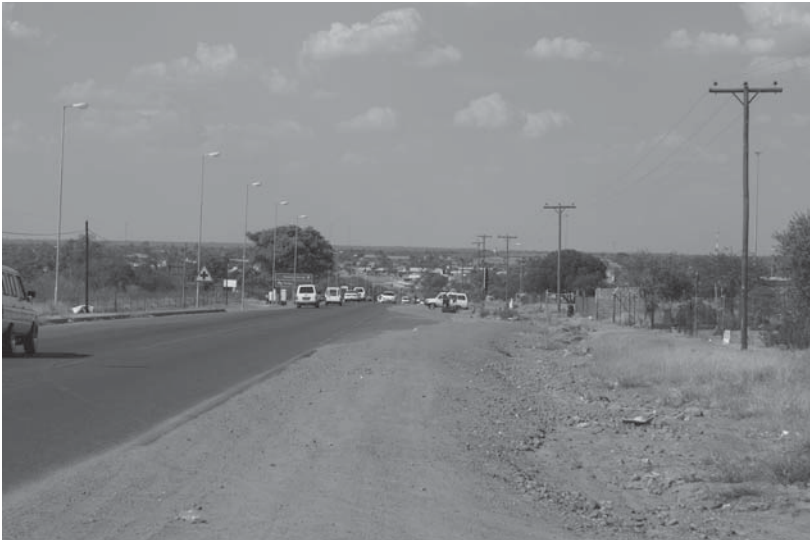
Figure 3.1 Hammanskraal to Soshanguve Road
