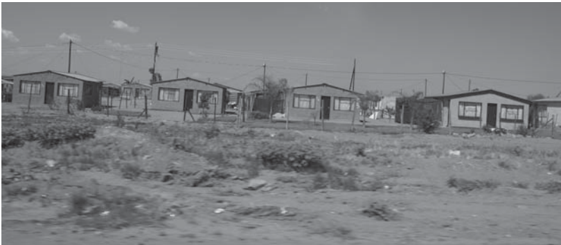
Figure 3.4 Parts of Kanana after RDP house building
