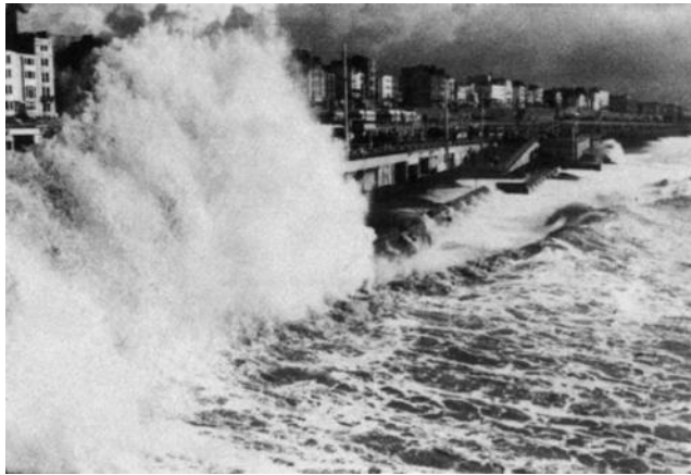
FIGURE 8.13 Wave impact and reflection during a storm.
