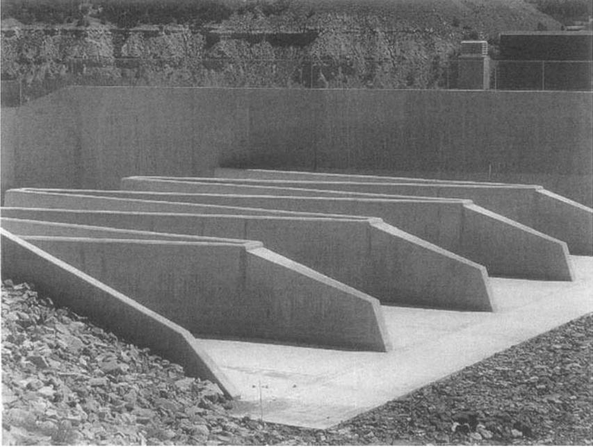
Figure 7. Ice Breaking Piers - Tongue River Dam, USA
