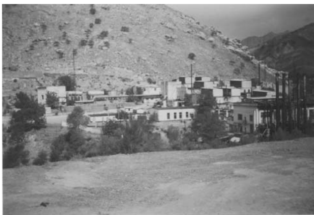
Photo 1. Former uranium plant near Mailuu-Suu River
