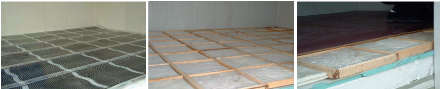
Fig. 9.55. Layered structure of an electric floor heating system. From left to right: electric heaters, wooden frame with plates of shape-stabilized PCM, and wooden floor cover (pictures: Tsinghua University, PR China)
