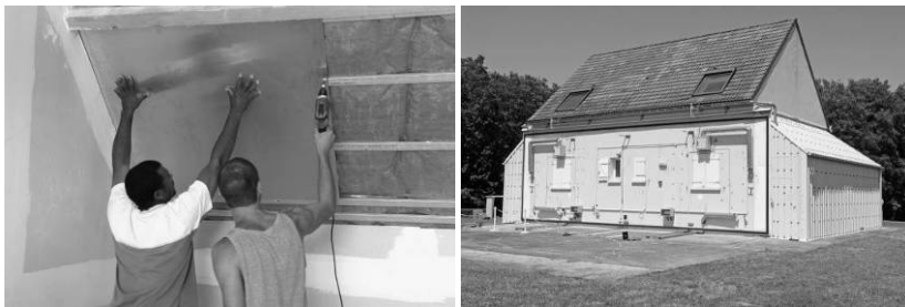
Fig. 9.16. Left: installation of a DuPont™ Energain® panel. Right: test site for experimental tests in a real building (pictures: DuPont).
