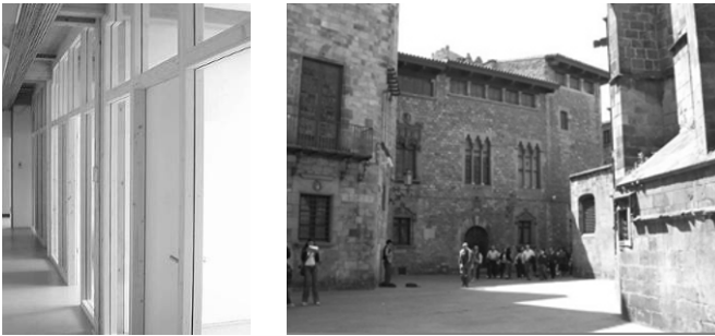
Fig. 9.3. Left: typical lightweight construction with wooden frame and glass windows. Right: typical heavy weight construction with massive stonewalls.
