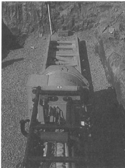
FIGURE 1. Machine Setup in the Pit.
