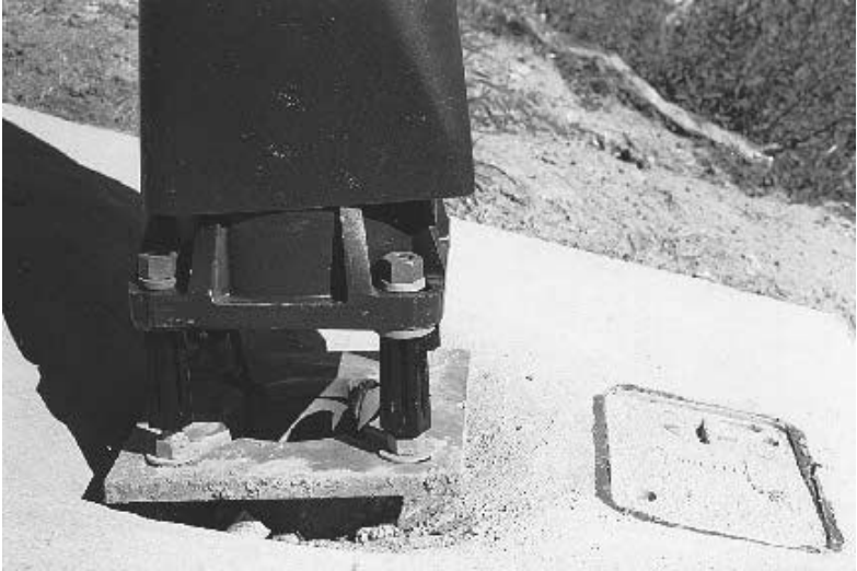
FIGURE 7.90 Frangible-coupling luminaire support.
