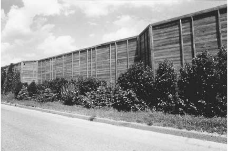
FIGURE 9.4 Timber noise wall with buttress-type alignment.
