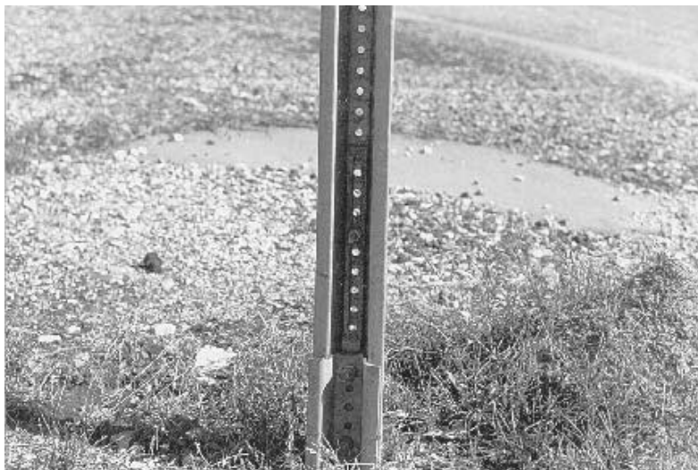
FIGURE 7.7 Example of breakaway single sign support.
