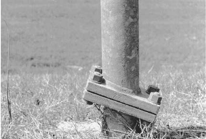
FIGURE 7.27 Installation of unidirectional slip base.
