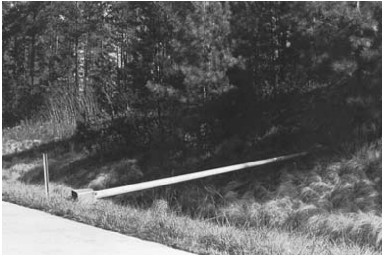
FIGURE 7.95 Failure of luminaire support without impact.
