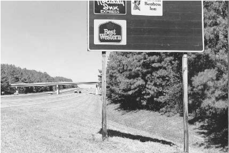
FIGURE 7.61 Multiple-mount frangible wood post design.
