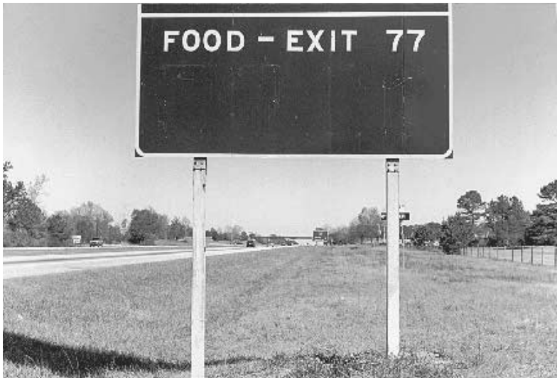
FIGURE 7.31 Multiple-mount sign support.
