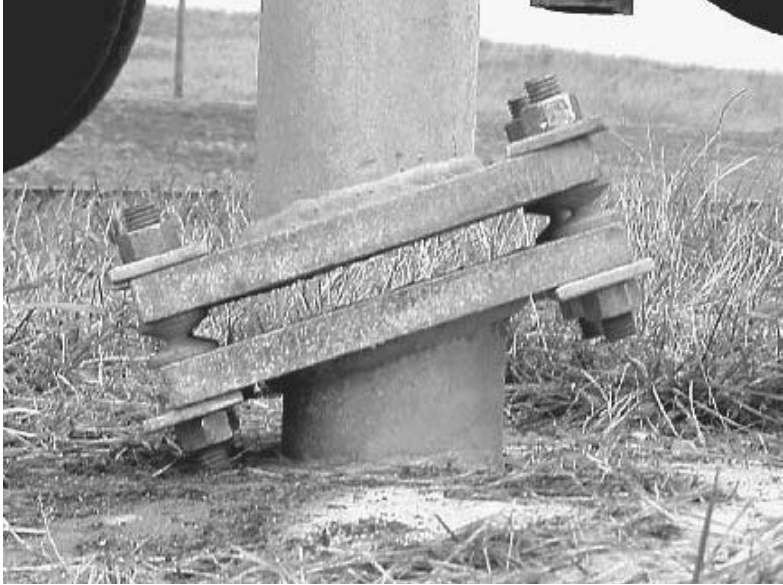
FIGURE 7.30 Frangible-coupling sign support.
