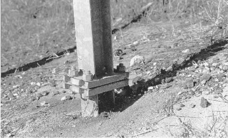
FIGURE 7.8 Example of mechanical release support type.
