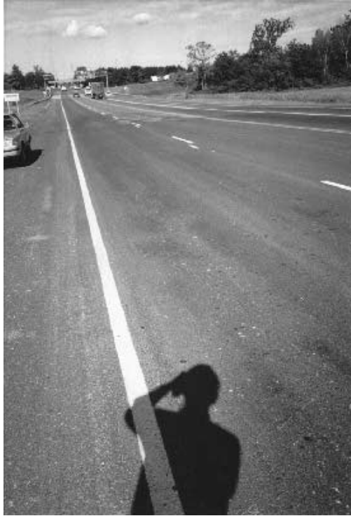
FIGURE 3.32 Example of bleeding in flexible pavement.
