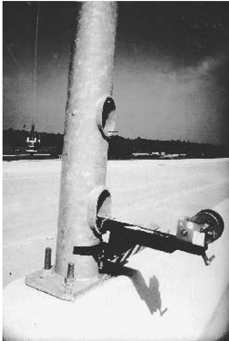
FIGURE 7.76 Lowering device manufactured by ITS Products Inc.
