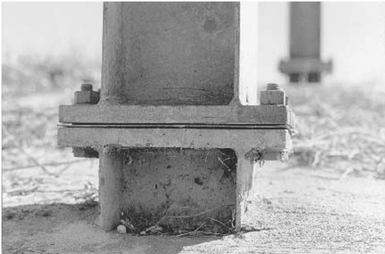
FIGURE 7.34 Installation of horizontal slip base.
