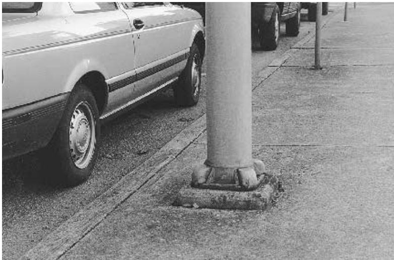
FIGURE 7.89 Flange-type steel base.
