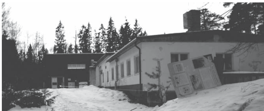
Fig. 4 The explosives approved zone used with the maximum safe distance, 55 m
