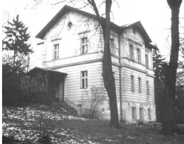
Figure 10. Historical building of the Astronomical Institute of Charles University, Švédská Street No. 8, Prague 5. (Photo of 1985 from author's archive.)
