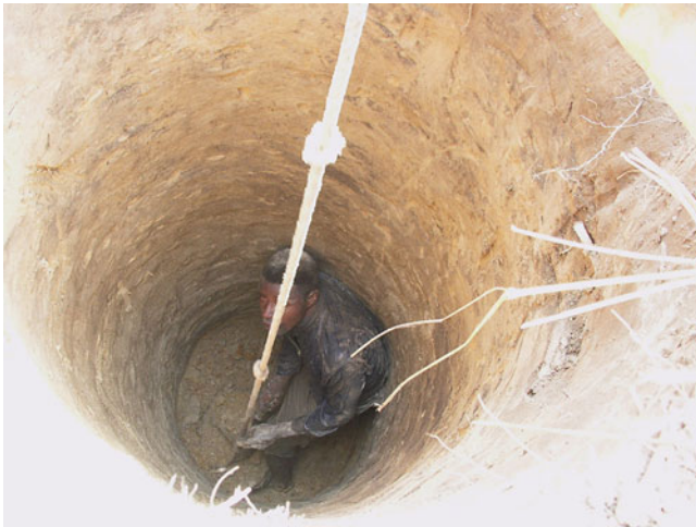
Fig. 16.13 Looking down a Majimba hole dug by hand in order to penetrate terrace deposits
