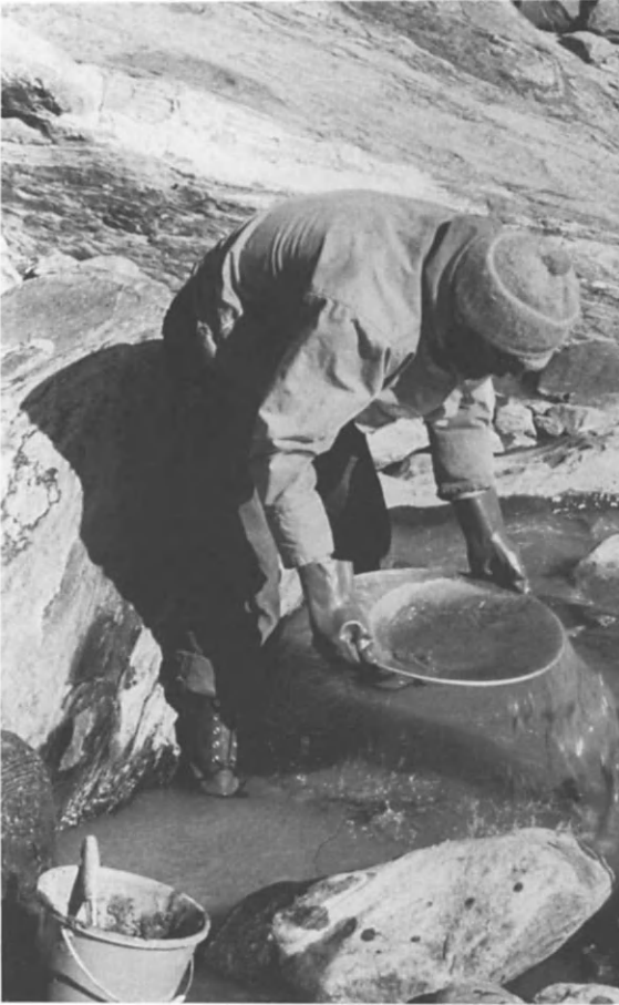
Fig. 6-8. (b) Panning techniques using a batêa. Photo by H. Stendal.
