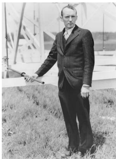
Bell Telephone Laboratories engineer Karl Jansky built this movable radio antenna in a field near Holmdel, New Jersey, in 1930 and called it his "merry-go-round." With it, he detected a mysterious radio hiss that proved to come from outside the solar system. (National Radio Astronomy Observatory/AUI/NSF)
