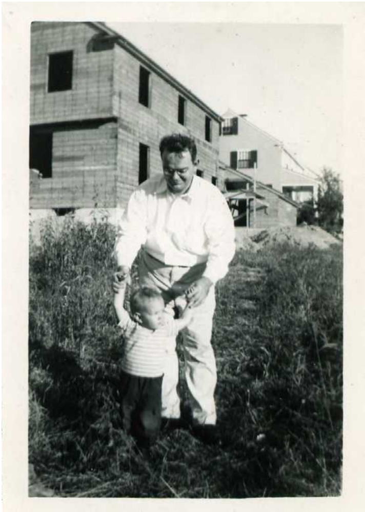
Fig. 1.1. Fred at the Belmont house construction site with his son, Bill, in 1948.
