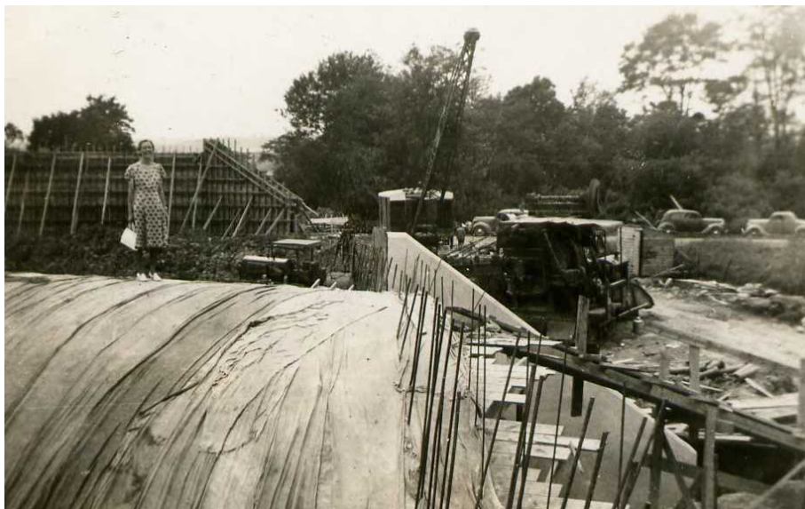
Fig. 10.1. Virginia at a road job in the late 1930s.
