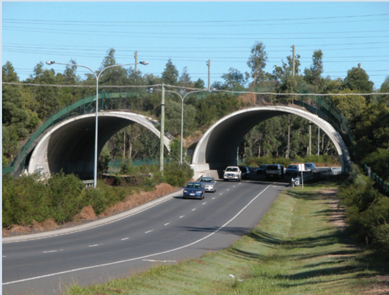
Figure 48.1 Wildlife overpass at Compton Road, in the suburbs of Brisbane, Australia. Due to successful negotiations between local government, community groups, ecologists and engineers, this site has a wide variety of mitigation measures to allow wildlife to cross the road. Source: Photograph by Darryl Jones.
