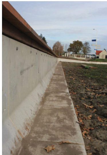
Figure 32.4 Barrier fence for reptiles with (A) grass that needs mowing to prevent animals from climbing over and (B) a well-maintained and durable fence with wide base, smooth wall and overhanging lip. Source: Photographs by R. P. J. H. Struijk.
