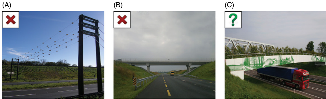
Figure 34.6 Over-the-road-crossing structures: gantries (A) and conventional overpasses (B) are not effective. Wildlife overpasses (C) have potential but need more research. Source: (A) Photograph by Anna Berthinussen, (B) Photograph by Isobel Abbott; and (C) Photograph © Herman Limpens/Zoogdierveniging. Reproduced with permission.
