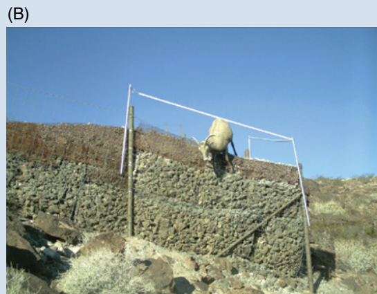
Figure 20.10 Desert bighorn sheep entering the roadway via a jump-out without modification (A) and a sheep successfully exiting the roadway via a jump-out with plastic pipe to provide a visible obstruction to deter access from outside the roadway while continuing to allow proper use (B). Eventually, the plastic pipe was replaced with metal bars at a height of 0.4 m. Source: Photographs by J.W. Gagnon.
