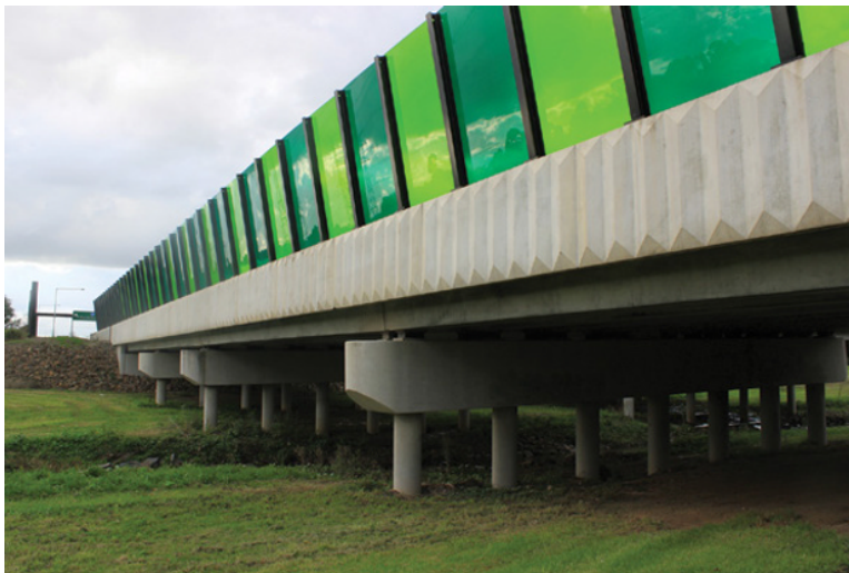
Figure 33.4 Fencing and walls on bridges can force birds to fly below the bridge or above the walls, hopefully avoiding traffic. In this example, in Australia, the coloured glass panels also act as sound and light walls. Walls of clear glass should be avoided to reduce the risk of bird-wall collision. Source: Photograph by Rodney van der Ree.
