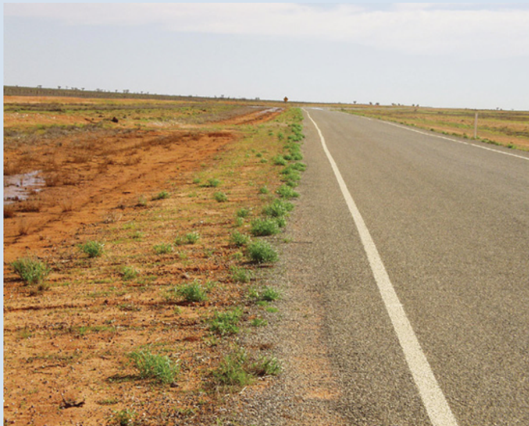
Figure 47.1 Increased cover, quality and productivity of plants along an arid-zone road in inland Australia. This arid-zone road is a typical low-formation, single-lane, sealed arid-zone road less than 10 m wide, lacking features such as bridges, median strips and crash barriers. Source: Photograph by E. Lee.
