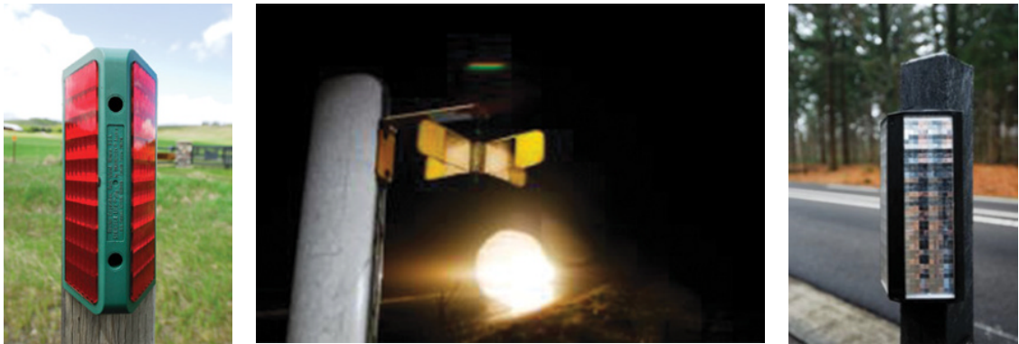
Figure 25.1 Three different types of roadside reflectors. Source: Photographs by Marcel Huijser.
