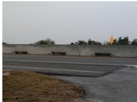
Figure 20.7 Jersey median barriers with drainage holes can trap animals, such as this river otter, and/or force them back into traffic (A), and while not ideal, animals that encounter such barriers in the centre median with larger holes (B) at least have a chance to make it across the road. Source: Photographs by D.J. Smith.
