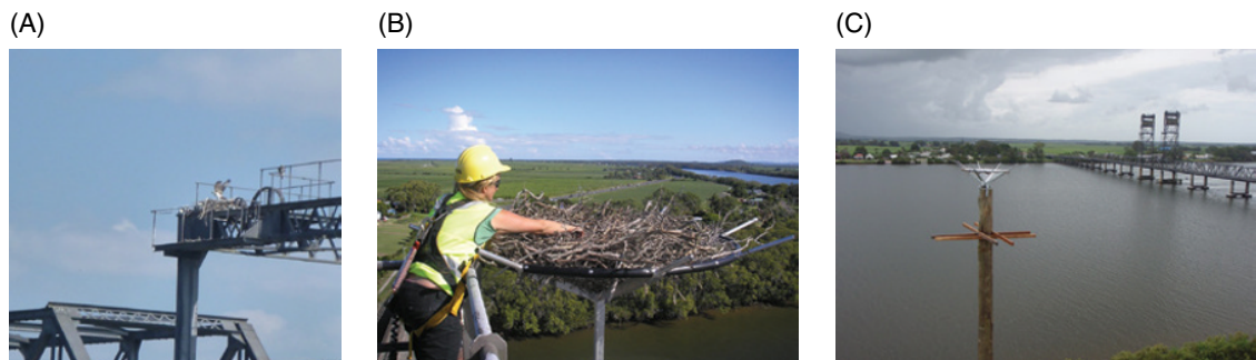
Figure 33.5 Ospreys frequently nest on bridge structures across rivers in northern coastal New South Wales, Australia (A), posing a traffic hazard and mortality risk to the birds. To alleviate this, artificial nesting platforms were erected at the highest point of bridges but suspended above the river (B). It soon became apparent that nesting by a threatened bird species could prevent maintenance during the breeding season, and nesting platforms are now erected on poles away from the bridge (C). Ospreys have successfully nested on many of these platforms and fledged young, allowing routine bridge maintenance to occur year-round. Source: Photographs by Kate Dallimore, Roads and Maritime Services, New South Wales.
