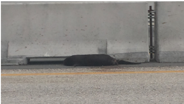
Figure 20.7 Jersey median barriers with drainage holes can trap animals, such as this river otter, and/or force them back into traffic (A), and while not ideal, animals that encounter such barriers in the centre median with larger holes (B) at least have a chance to make it across the road. Source: Photographs by D.J. Smith.
