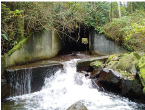
Figure 44.5 These culverts have constricted the flow of water, which increases velocity and leads to erosion at the outfall. When originally installed, these culverts were at the same elevation as the streambed but over time, erosion has led to a significant outfall drop, creating a vertical barrier to the upstream movement of fish and other aquatic organisms. As this process continues, the integrity of the culvert and the road fill is at risk. Source: Photography by Paul J. Wagner - Washington State Department of Transportation.
