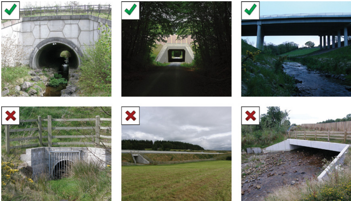
Figure 34.4 Bat-friendly underpasses (top row of images) are spacious and connected with flight paths along streams, woodland lanes or hedgerows. Underpasses that are too small, blocked with vegetation or grilles, situated in open ground, wide but too low, flood prone or disturbed by lighting (e.g. bottom row of images) are much less beneficial to bats. Source: (top left, top right, bottom left, bottom middle, bottom right) Photographs by Isobel Abbott; and (top middle) Photograph by Markus Melber.
