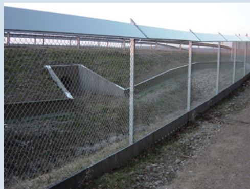
Figure 35.10 (A) The European wildcat is identified by the circular black rings on its tail. (B) Fences for wildcats in Germany are 2 m high with mesh size of 5 cm 2 , a 50 cm-wide overhanging metal sheet and plastic board buried 30 cm deep. Source: (A) Photograph by and reproduced with permission of Heiko Müller-Stieß; and (B) Photograph by N. Klar.
