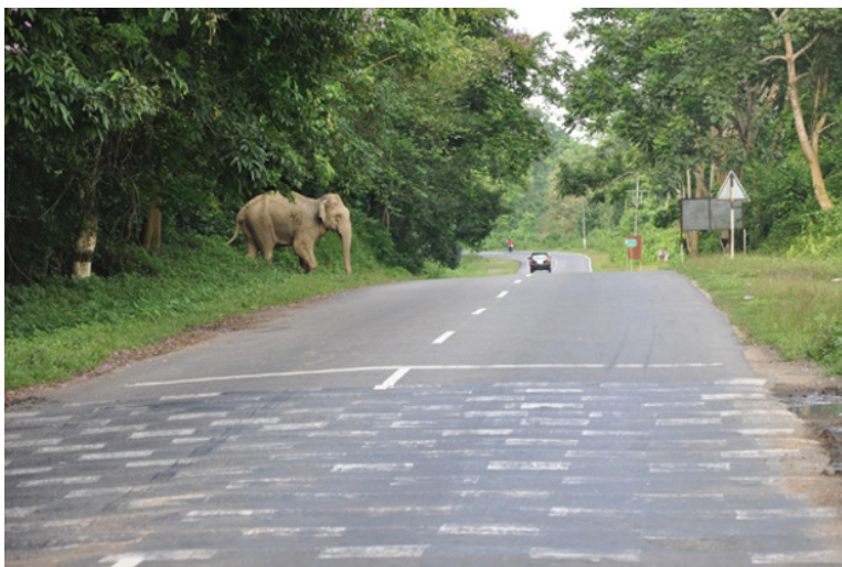
Figure 53.4 Elephant from the Kaziranga National Park in India approaches NH-37. In situations like this, a cleared verge provides wildlife and drivers with time and space to see each other and potentially avoid WVC. Source: Photograph by A. Pragasheesh © WII 2013. Reproduced with permission from Wildlife Institute of India.
