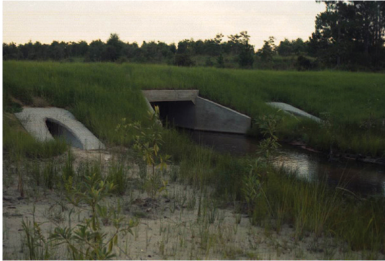
Figure 21.4 The two pipe culverts are elevated above the box culvert used for stream flow, providing dry passage for wildlife. Source: Photograph by D.J. Smith.
