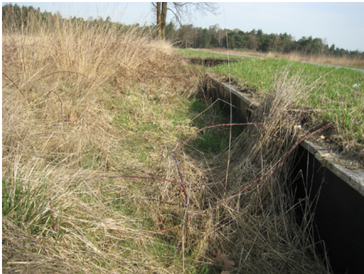
Figure 32.4 Barrier fence for reptiles with (A) grass that needs mowing to prevent animals from climbing over and (B) a well-maintained and durable fence with wide base, smooth wall and overhanging lip. Source: Photographs by R. P. J. H. Struijk.
