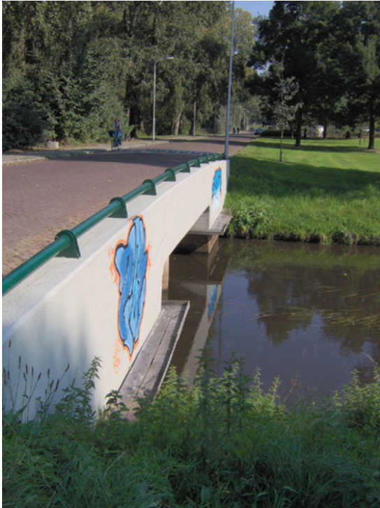
Figure 39.3 Shelves for small mammals on both walls of a culvert near Eindhoven, the Netherlands. Source: Photograph by R. van der Ree.
