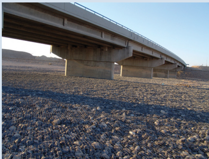
Figure 47.3 Netting the surface below a bridge into gabions may affect the natural flow of water, soil and organic material and may also affect animal movement. Source: Photograph by and reproduced with permission of Dr. Ron Frumkin.
