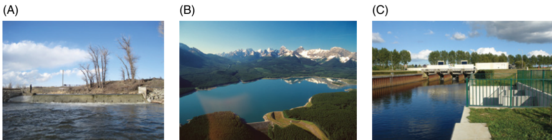
Figure 45.3 Other examples of structures that are barriers to fish movement include (A) this low-head dam in Montana USA, (B) this large dam for hydropower in Canada and (C) this sluice to control water levels in North Brabant, the Netherlands. Source: (A and B) Photographs by Matt Blank; and (C) Photograph by Fabrice Ottburg.
