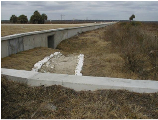
Figure 20.6 Solid wall at Paynes Prairie, Florida, immediately after construction (A) and a few years later (B). Wall height is 1.1 m, culvert is 1.8 m × 1.8 m, and the overhanging lip protrudes by about 15 cm. Source: Photographs by D.J. Smith.
