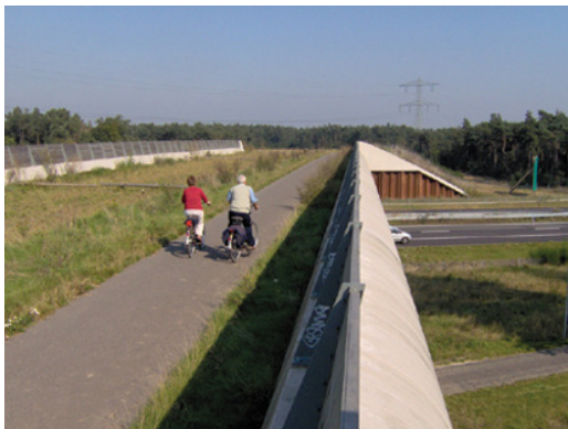
Figure 22.1 (A) Recreational use by cyclists of the land bridge at Slabroek, The Netherlands. (B) This wildlife overpass in Brisbane, Australia, has boulders separating the recreational and wildlife zones. Both structures are just 15 m wide, and neither represents best practice in co-use design (Lesson 22.3). Source: Photograph (A) by Rodney van der Ree and (B) by Edgar van der Grift.
