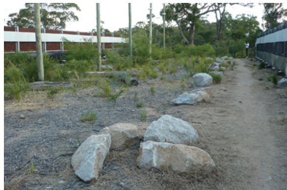
Figure 22.1 (A) Recreational use by cyclists of the land bridge at Slabroek, The Netherlands. (B) This wildlife overpass in Brisbane, Australia, has boulders separating the recreational and wildlife zones. Both structures are just 15 m wide, and neither represents best practice in co-use design (Lesson 22.3). Source: Photograph (A) by Rodney van der Ree and (B) by Edgar van der Grift.
