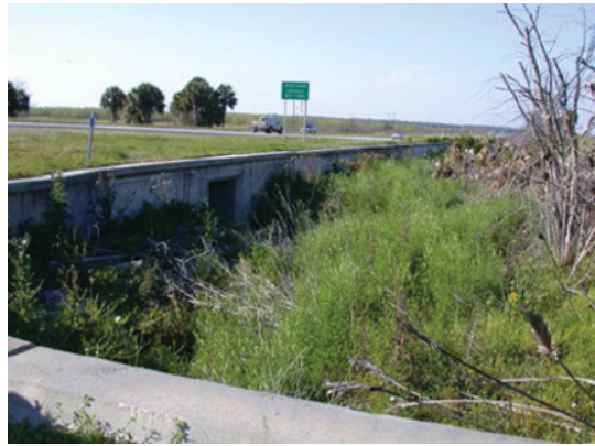
Figure 20.6 Solid wall at Paynes Prairie, Florida, immediately after construction (A) and a few years later (B). Wall height is 1.1 m, culvert is 1.8 m × 1.8 m, and the overhanging lip protrudes by about 15 cm. Source: Photographs by D.J. Smith.
