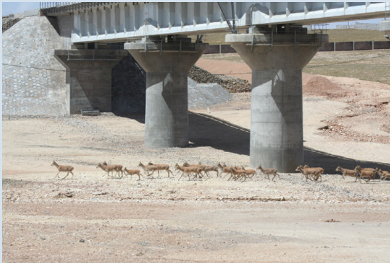
Figure 57.3 Tibetan antelopes using the Hoh Xil wildlife crossing structure in August 2006, shortly after the railway was opened. Source: Reproduced with permission of Hongfeng Zhang, Northwest Institute of Endangered Zoological Species.
