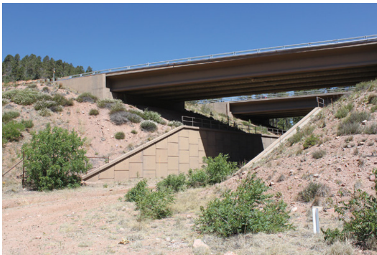
Figure 23.4 Avoid abutments or ledges in underpasses such as those shown here on State Route 260, Arizona, United States, where ambush predators may hunt from. Source: Photograph by R. van der Ree.
