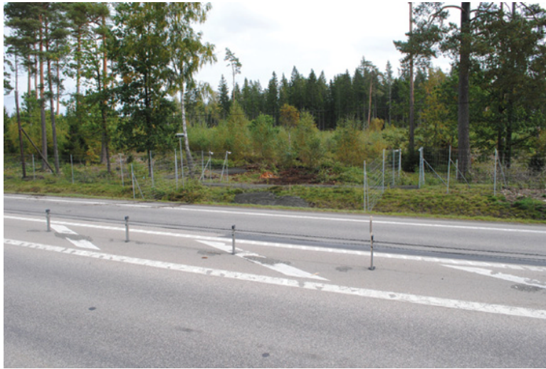
Figure 24.10 Moose detection system at a gap in a wildlife fence, southern Sweden. Source: Photograph by Mattias Olsson.
