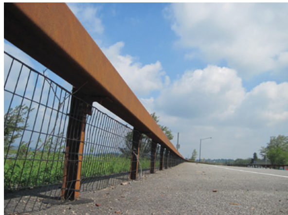
Figure 20.2 (A) This cost-effective temporary retrofit of a 1.2 m-high livestock fence to a height of 2.4 m along Interstate 17 in Arizona reduced the rate of elk-vehicle collision by 100%. Note the coloured tape on the top strand to warn birds of the new fence. (B) Simple wire mesh added to existing guard rail to reduce WVC with snapping turtle, New York. In all mitigation and especially retrofits, it is essential to ensure that a cheap option is also ecologically effective. Source: (A) Photograph by J.W. Gagnon and (B) Photograph by and reproduced with permission from Tom Langen.
