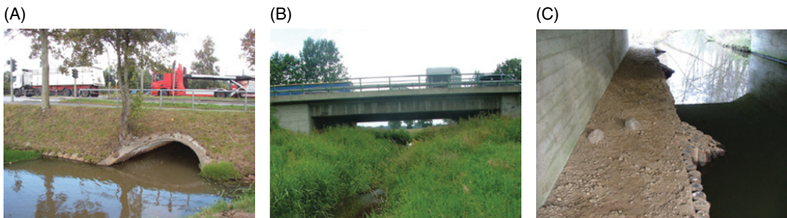
Figure 35.6 Examples of river otter crossings: (A) unsuitable culvert design with high risk of submersion from flooding, (B) superior design with riparian strips and (C) retrofitted culvert with dry ledge including aquatic entry points for otters. Source: Photographs by N. Klar.
