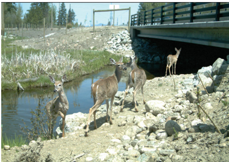
Figure 42.2 White-tailed deer move through an underpass in Montana, United States, with a pathway cleared through large rocks Source: Photograph by P. Cramer and Montana DOT.
