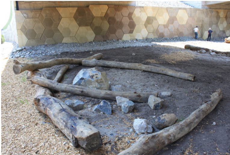
Figure 39.1 Logs and rocks in this underpass offer cover and protection to small animals. Ideally, the logs and rocks would provide continuous cover through the underpass. Source: Photograph by R. van der Ree.
