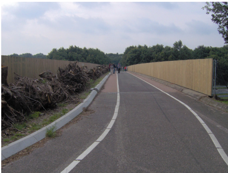
Figure 39.2 A line of tree stumps as shelter for small mammals, reptiles, amphibians and invertebrates on a small multi-use bridge overpass in the Netherlands. Source: Photograph by R. van der Ree.
