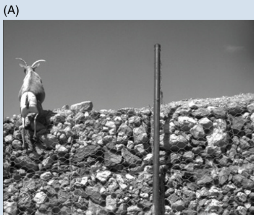
Figure 20.10 Desert bighorn sheep entering the roadway via a jump-out without modification (A) and a sheep successfully exiting the roadway via a jump-out with plastic pipe to provide a visible obstruction to deter access from outside the roadway while continuing to allow proper use (B). Eventually, the plastic pipe was replaced with metal bars at a height of 0.4 m. Source: Photographs by J.W. Gagnon.
