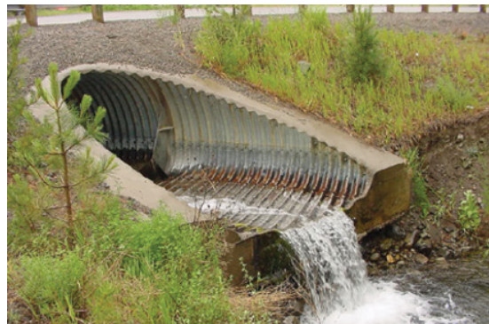
Figure 44.5 These culverts have constricted the flow of water, which increases velocity and leads to erosion at the outfall. When originally installed, these culverts were at the same elevation as the streambed but over time, erosion has led to a significant outfall drop, creating a vertical barrier to the upstream movement of fish and other aquatic organisms. As this process continues, the integrity of the culvert and the road fill is at risk. Source: Photography by Paul J. Wagner - Washington State Department of Transportation.
