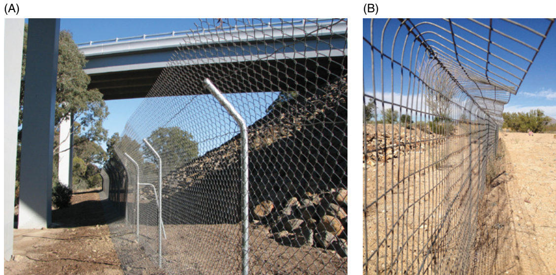
Figure 20.4 (A) Floppy top fence for koalas and (B) curved fence for desert tortoise in Arizona. Source: (A) Photograph by R. van der Ree and (B) Photograph by and reproduced with permission from Scott Sprague.
