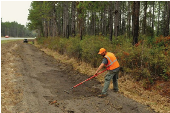
Figure 11.2 (A) Preparation of a track bed parallel to the road using naturally occurring soil. The track bed should be wide enough to ensure the target species will leave several footprints when crossing. (B) Red wolf imprint. Source: Photographs by D.J. Smith.
