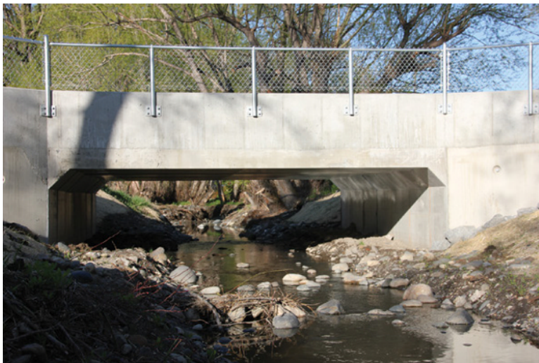
Figure 45.5 This recently constructed crossing of Fleshman Creek, Montana, was designed using the stream-simulation approach. The culvert maintains the stream channel and bank lines through the entire structure, thus ensuring fish passage for most flows. The structure is designed to provide flood conveyance up to the 100 year event. Source: Photograph by Matt Blank.
