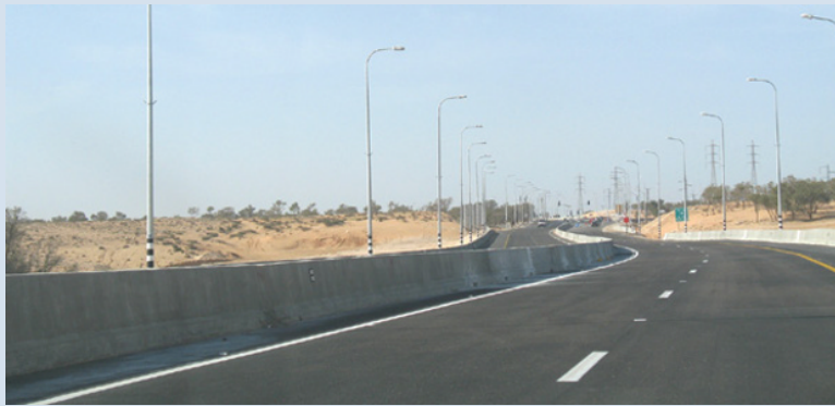
Figure 47.2 A large, multi-lane and engineered arid-zone road may fragment habitat. Source: Photograph by T. Achiron-Frumkin.
