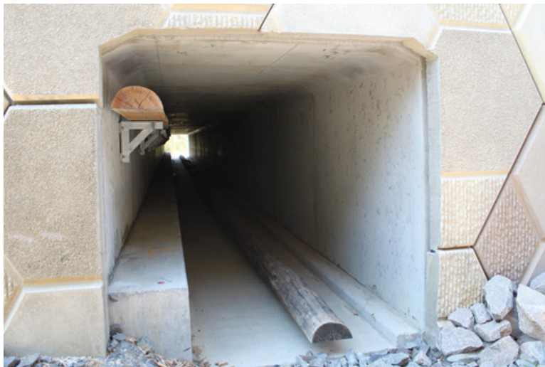
Figure 9.1 The concrete shelf and elevated poles designed to facilitate crossings by small to medium-sized and arboreal mammals in this wildlife underpass are less effective (and possibly ineffective) because they have not been connected to the surrounding habitat. Source: Photograph by R. van der Ree.
