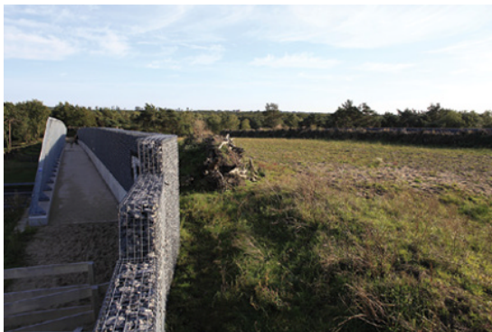
Figure 22.2 Examples of internal screening on land bridges in The Netherlands. (A) Rock gabion walls on Wolfheze land bridge and (B) earth berm with shrubs on the Zanderij Crailoo land bridge. Source: Photographs by Edgar van der Grift.
