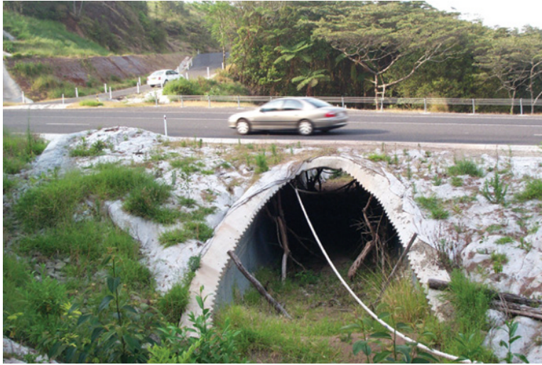
Figure 40.5 Logs and ropes provide refuge for tree kangaroos from terrestrial predators in this underpass on the Atherton Tablelands, Australia. Source: Photograph by R. van der Ree.
