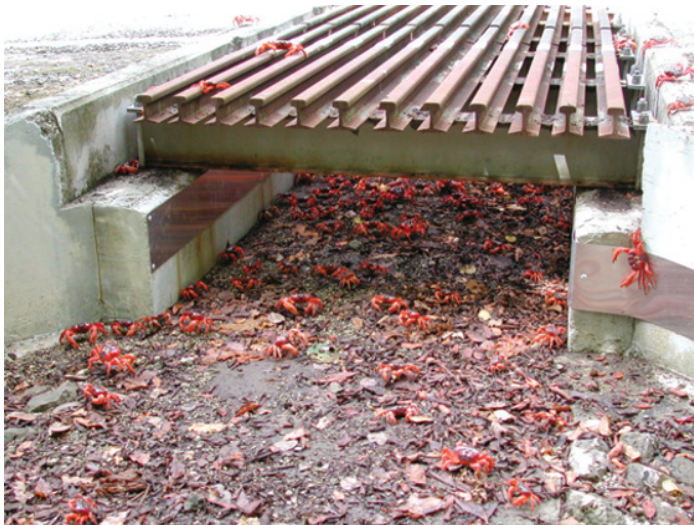
Figure 30.2 Small, open-topped underpasses (A) with funnel fencing (B) are the key mitigation measures to reducing mortality and maintaining crab movements. Source: Photographs reproduced with permission of Parks Australia.
