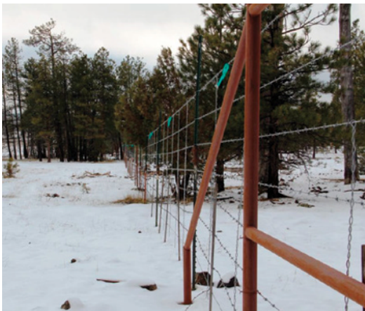
Figure 20.2 (A) This cost-effective temporary retrofit of a 1.2 m-high livestock fence to a height of 2.4 m along Interstate 17 in Arizona reduced the rate of elk-vehicle collision by 100%. Note the coloured tape on the top strand to warn birds of the new fence. (B) Simple wire mesh added to existing guard rail to reduce WVC with snapping turtle, New York. In all mitigation and especially retrofits, it is essential to ensure that a cheap option is also ecologically effective. Source: (A) Photograph by J.W. Gagnon and (B) Photograph by and reproduced with permission from Tom Langen.
