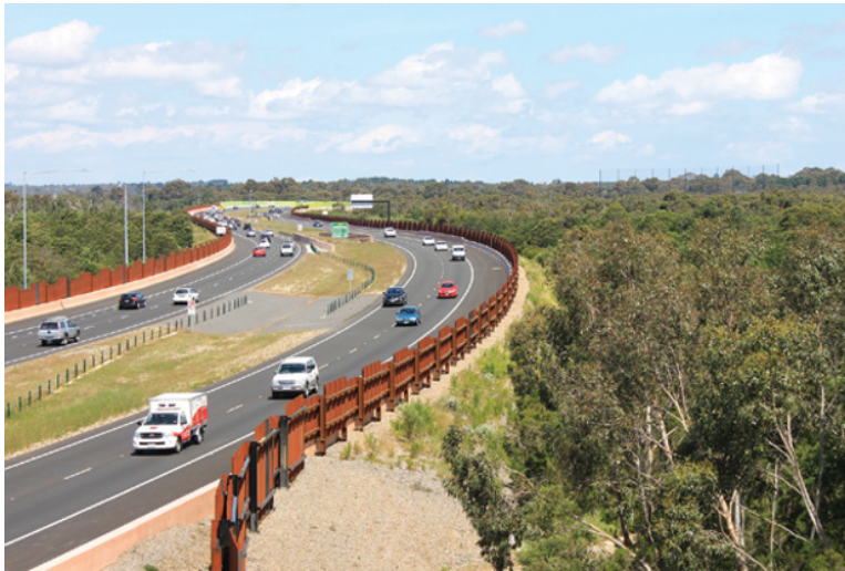
Figure 33.3 The elevated road plus 3–4 m tall solid walls along Peninsula Link in Victoria, Australia, may force some birds to fly up and over the traffic, avoiding WVC. However, the efficacy of this approach has not been evaluated, and this road and walls may be a barrier to movement for some species. Source: Photograph by Rodney van der Ree.
