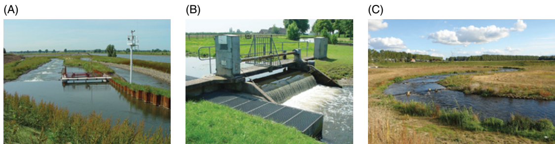
Figure 45.7 A series of step-pools or pool weirs (A), De Wit fish ladder inside the rectangular steel box (B) and semi-natural bypass (C) are used on rivers in the Netherlands to bypass barriers to fish movement. The water velocity through fish ladders, culverts and other structures must not exceed the swimming speed of any life stage or species living within the waterway. In lowland streams common to flat landscapes, water velocities < 1.0 m/s are typical, and most adult fish species are capable of moving through passages with such conditions. For subadults or juvenile fish, water velocities should be < 0.8 m/s or even < 0.4 m/s for some species (Jens 1982; Lieffering et al. 2005; Gough et al. 2012). Source: Photographs by Fabrice Ottburg.
