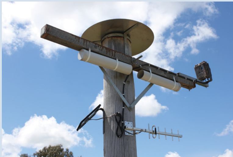
Figure 40.4 PVC tubes on glider poles provide protection for arboreal animals, in this case squirrel gliders, from aerial predators. Camera for monitoring and antenna to transmit images are also shown. Source: Photograph by R. van der Ree.
