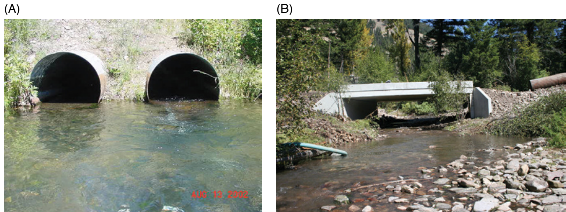
Figure 45.6 Pipe culverts (A) on the Clearwater River, Montana, were replaced with a bridge (B) to provide natural channel function and improve passage for all fish species and life stages. Source: Photographs by and reproduced with permission of Shane Hendrickson.
