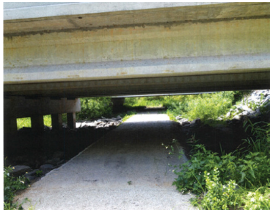
Figure 21.5 Example of (A) before and (B) after removal of riprap and creation of dry ledge adjacent to stream to facilitate use by white-tailed deer. Source: Photographs by D.J. Smith.
