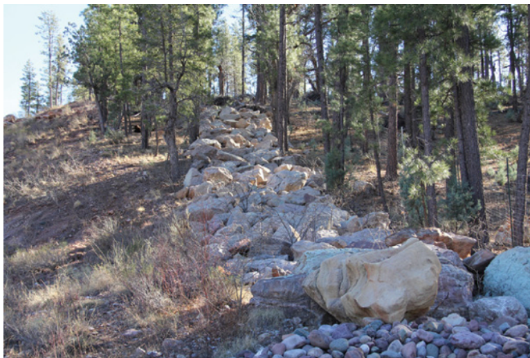
Figure 20.8 This riprap was installed to funnel deer and elk towards crossing structures. While initially successful, deer and elk managed to negotiate their way through and fencing had to be retrofitted. Source: Photograph by J.W. Gagnon.
