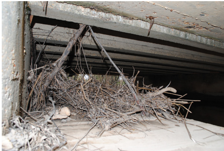
Figure 35.5 Logs and brush were included inside this underpass to provide cover for carnivores and small mammals. Source: Photograph by C. Grilo.
