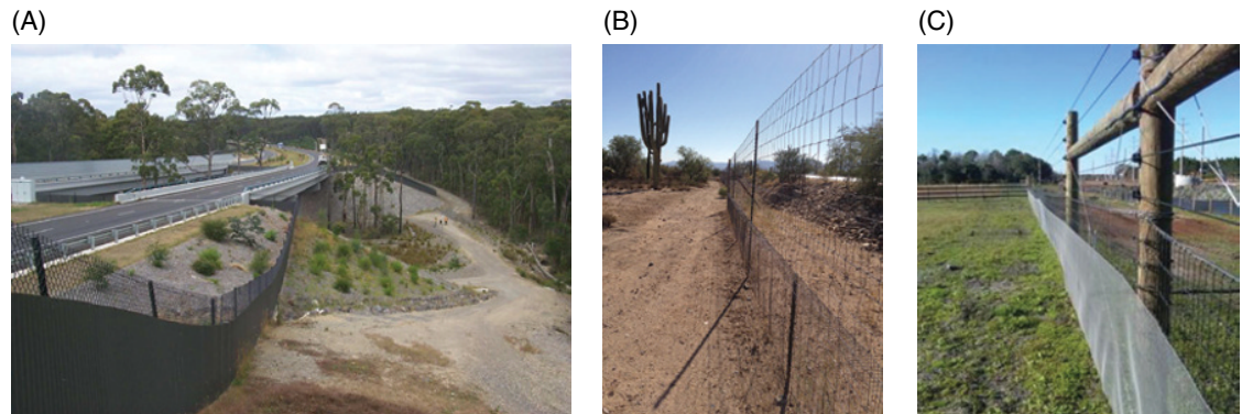
Figure 20.5 Examples of combination fencing for multiple species. (A) A 2.4 m-high wire mesh fence with sheet metal below to prevent arboreal species and kangaroos from climbing or jumping over, Victoria, Australia; (B) fencing for deer and tortoise in Arizona; (C) a 0.635 cm 2 mesh fence for reptiles and amphibians with 1.2 m aboveground and 30 cm belowground, with a stock fence to 1.5 m and ElectroBraid to 2.4 m, Florida. Source: (A) Photograph by R. van der Ree, (B) Photograph by J.W. Gagnon and (C) Photograph by D.J. Smith.
