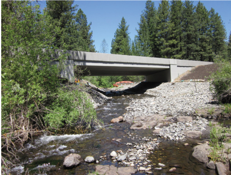
Figure 44.6 Example of a stream crossing designed using the stream simulation concept. This bridge spans the channel even at high flows and under normal flows has a significant area which is available for passage by terrestrial species. This photo was taken when construction was just finishing up at Butler Creek in Washington State, USA, and deer had already begun to use it to cross under this rural highway. Source: Photograph by Paul J. Wagner.
