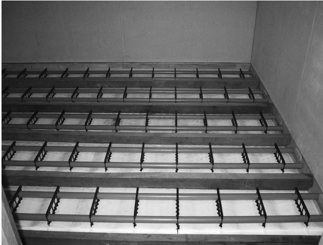
Figure 28. EPS Composite Panels for Floor Insulation.
