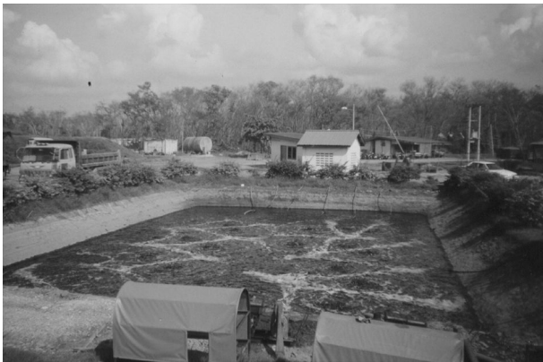
Figure 3. Leachate Collection Pond (End Line of Main Leachate Pipeline). 7
