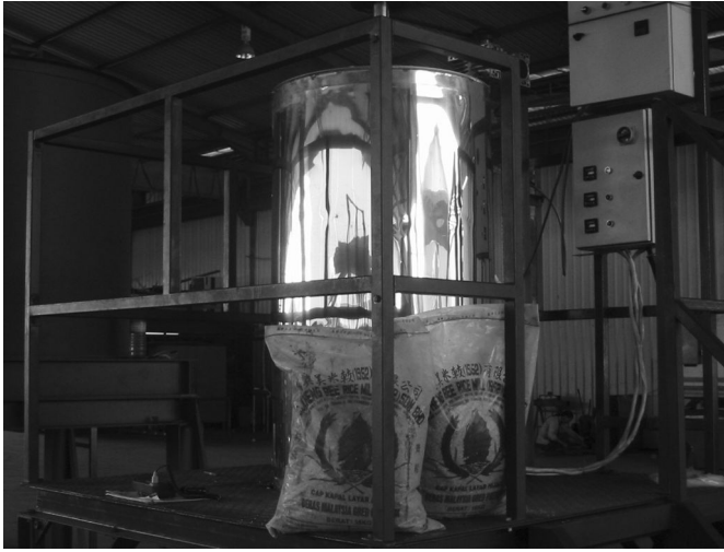
Figure 33. Rotary Furnace for Controlled Incineration of Rice Husk.
