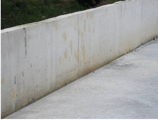
Figure 31. Cast in situ Engineered Shear Wall.
