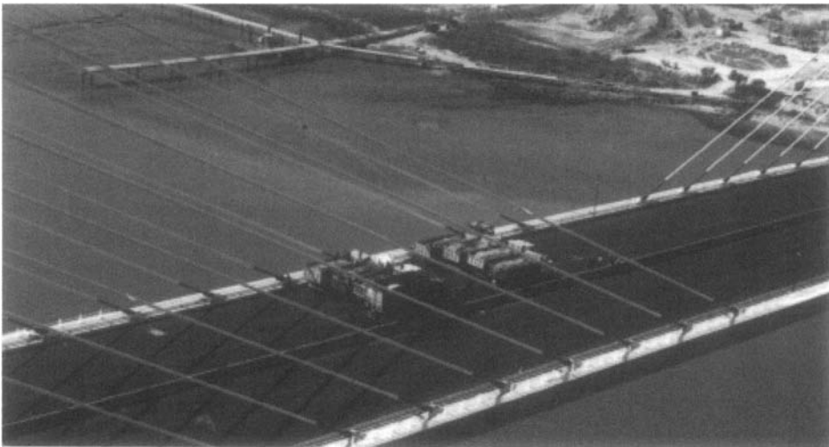
Figure 10-10. Bridge load test made with several lorries filled with sand
