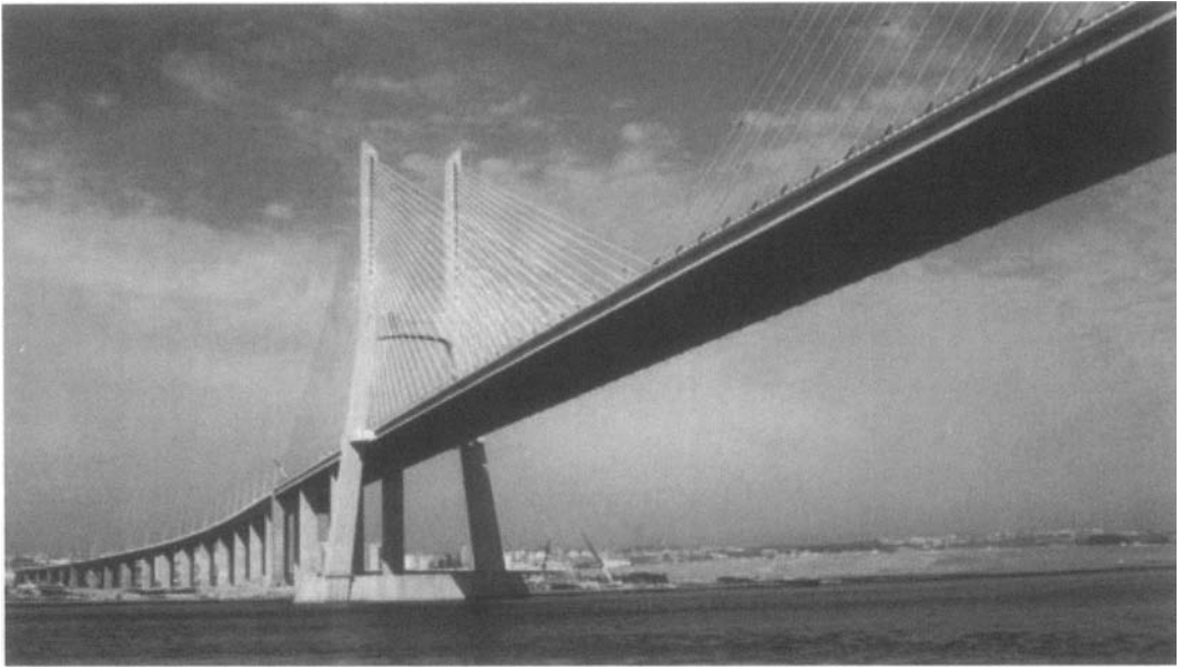
Figure 1-7. Vasco da Gama Bridge, in Lisbon, Portugal, was designed for a 120-year service life
