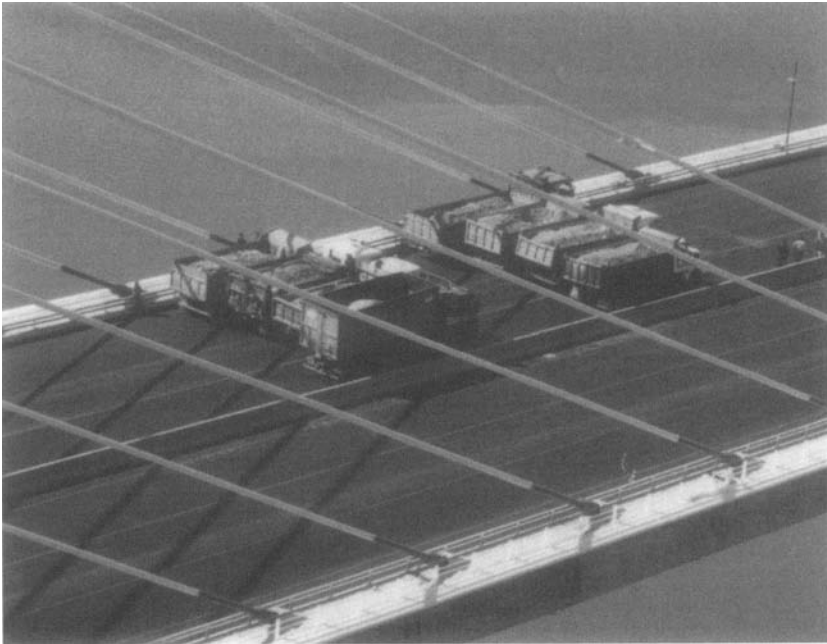
Figure 3-1. Bridge load testing
