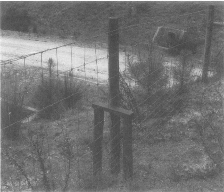
Figure 10-3. Simple device to clear fences
