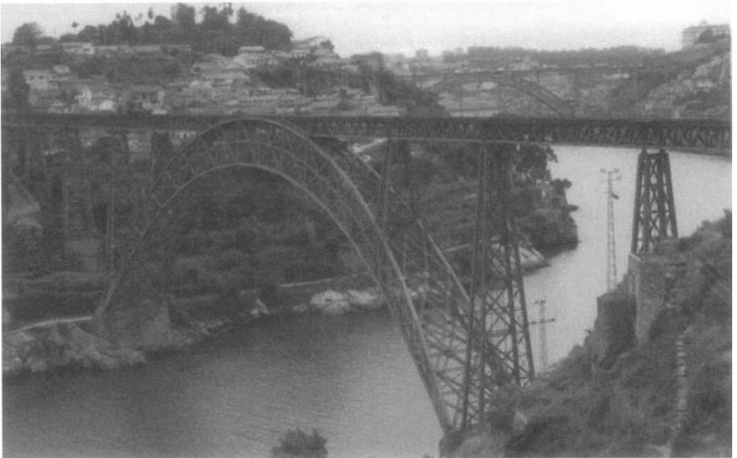
Figure 1-4. Maria Pia Railway Bridge (1877) in Porto, Portugal, built by Gustave Eiffel in wrought iron
