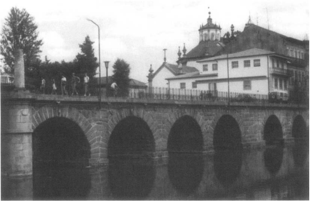
Figure 1-1. 2,000-year-old Roman bridge, still in service, in Chaves, Portugal
