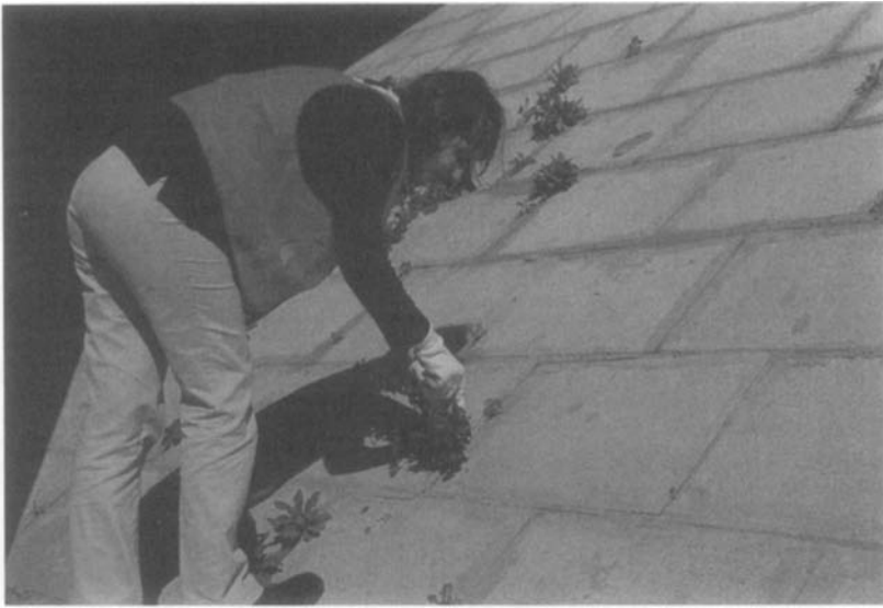
Figure 10-5. Routine maintenance during an inspection: vegetation removal
