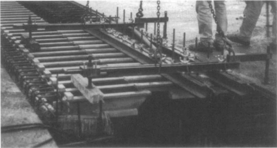
Figure 5-20. Placement of a bridge joint
