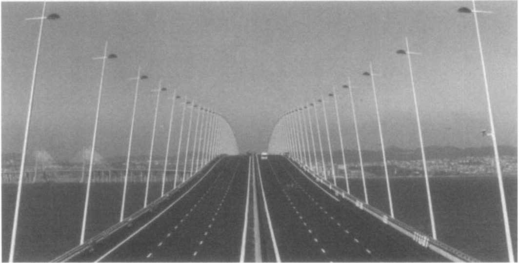
Figure 2-3. Vasco da Gama Bridge in Lisbon, Portugal, with 2 × 3 lanes, able to support 2 × 4 lanes
