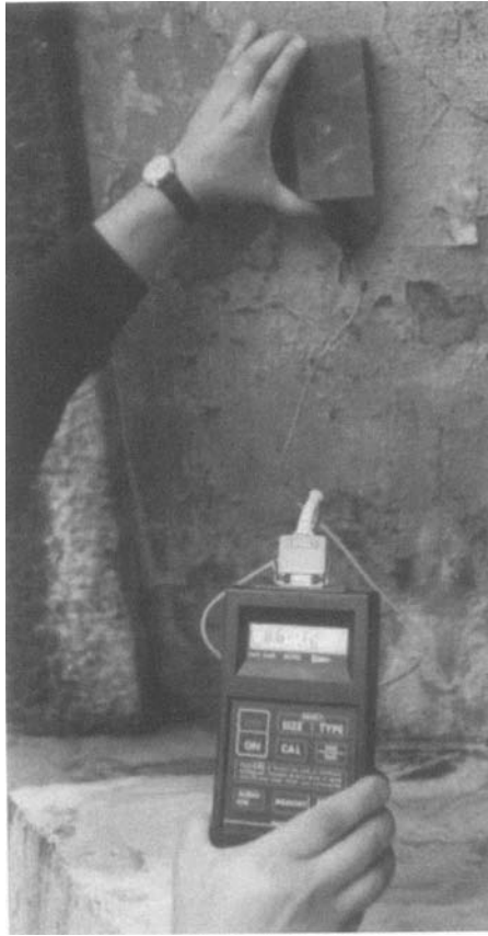
Figure 3-16. Use of covermeter
