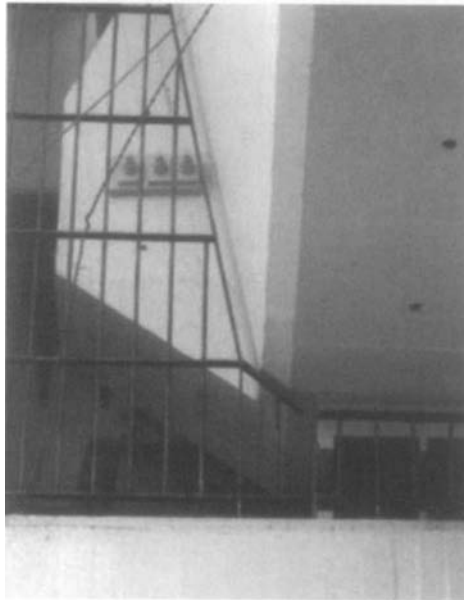
Figure 4-14. Protected access to an abutment
