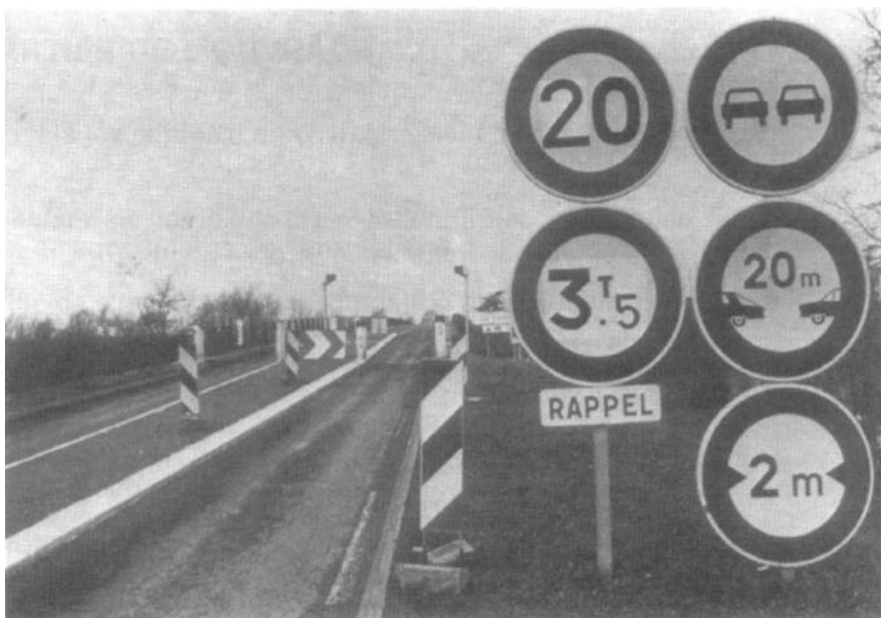
Figure 7-9. French bridge in which traffic is seriously restricted
