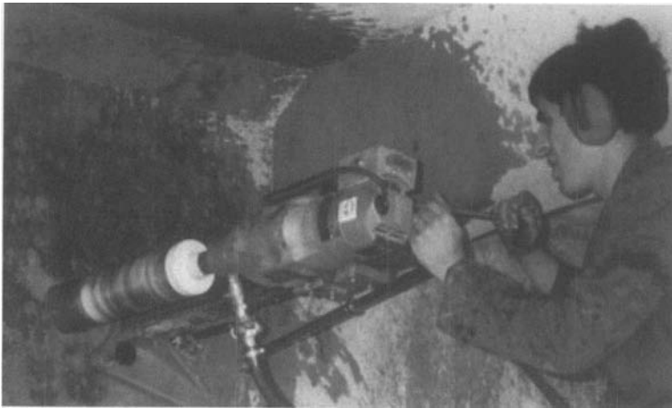
Figure 3-10. Drilling a core
