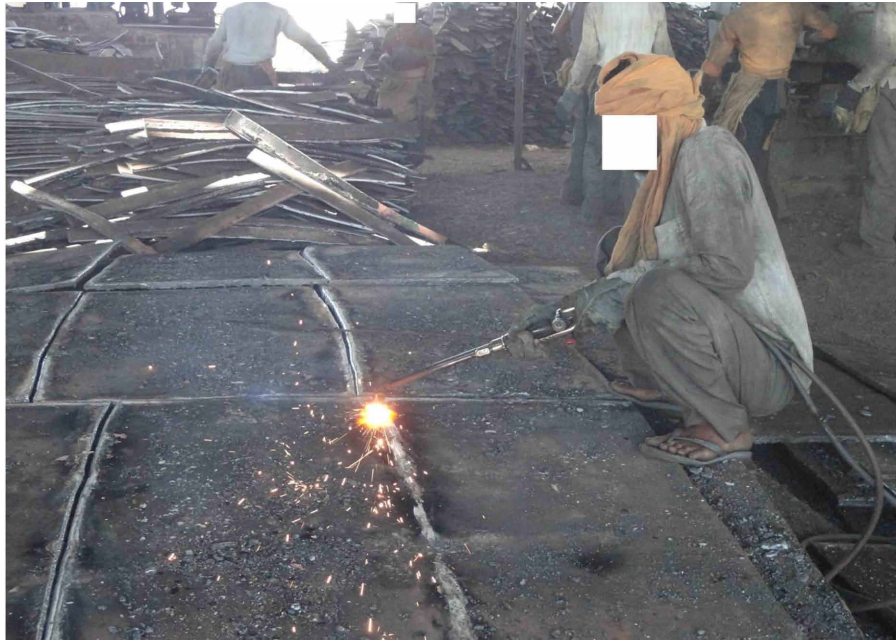
Figure 3. Worker carrying out welding activity in semi-shaded workplace
