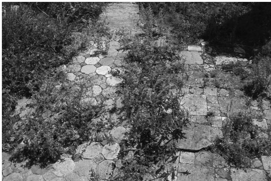
Figure 14.2 Neglected remains of the fifth-century church of St Barnabas near Salamis: Opus sectile floor being destroyed by vegetation (Susan Balderstone).
