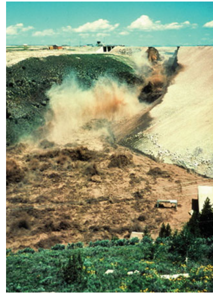
The Teton Dam in southeastern Idaho collapsed on first filling on June 5, 1976, causing the deaths of 11 people and $2 billion in damages.
