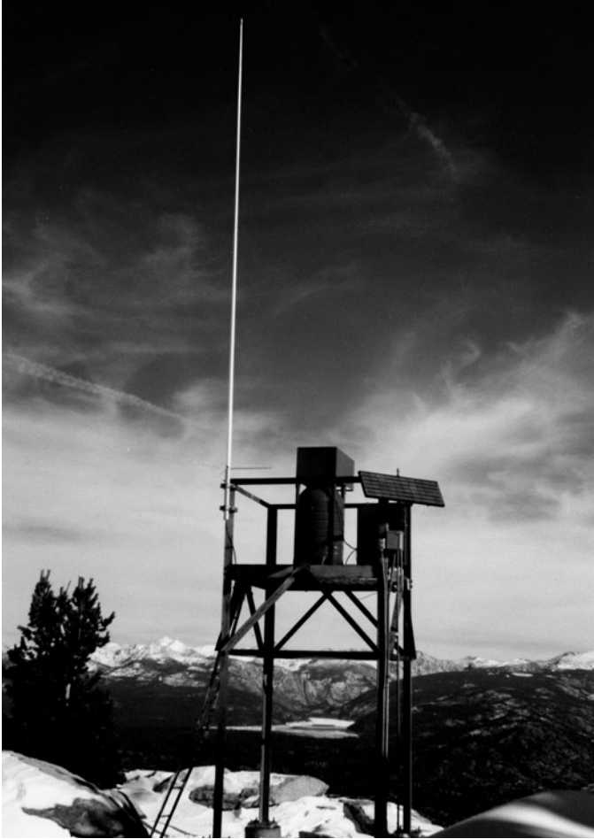
FIGURE 5-7. Remotely Controlled, Ground-Based Silver Iodide Generator (Griffith et al., 1995).
