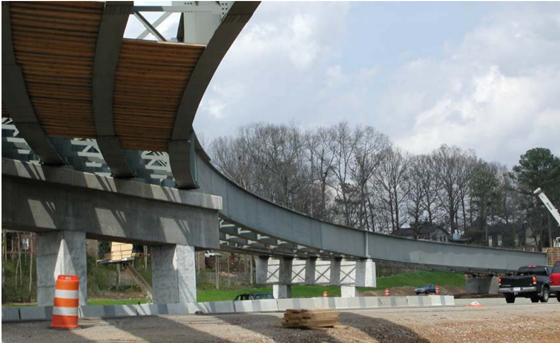
Figure 4.42. EICCS1, I-459 / US31 Interchange Flyover A, Jefferson Co. AL (Osborne, 2002).
