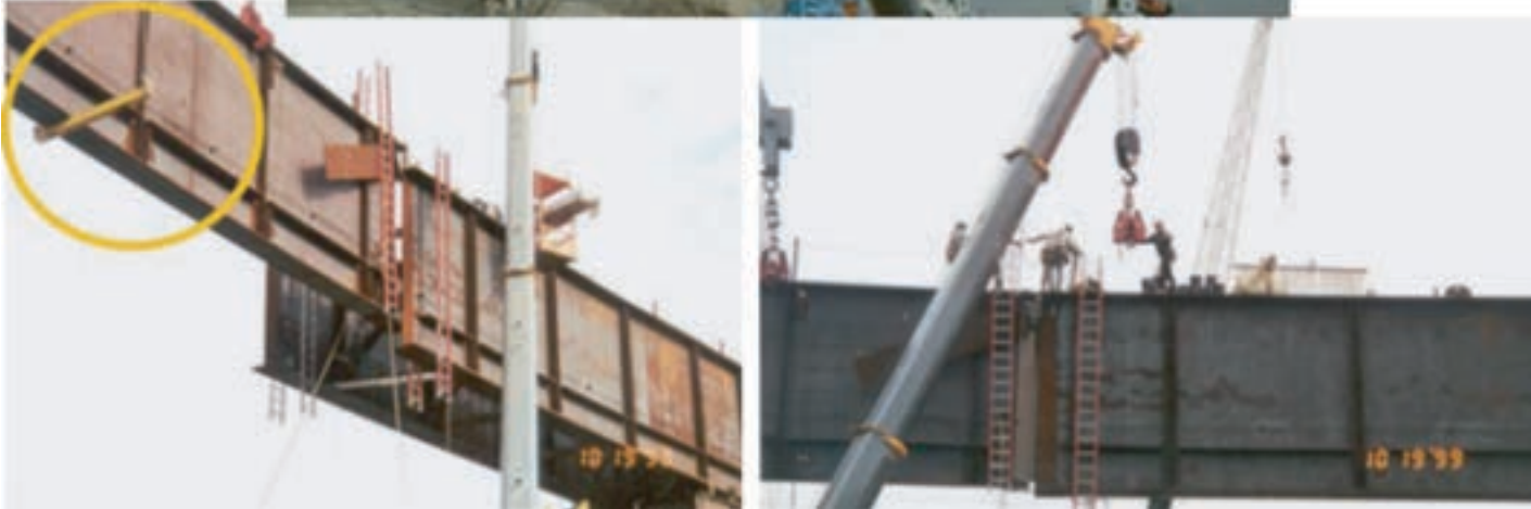
Figure 3-81. Ford City Bridge (EICCR11) installation of drop-in segment (Chavel, 2008).
