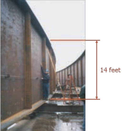
Figure 3-80. Ford City Bridge (EICCR11) girder depth and spacing (Chavel, 2008).
