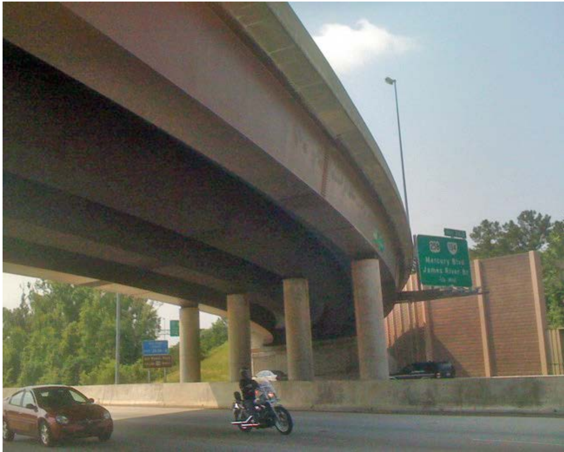
Figure 4.45. ETCCS6, McGruder Blvd. bridge over I-64 in Hampton, VA.
