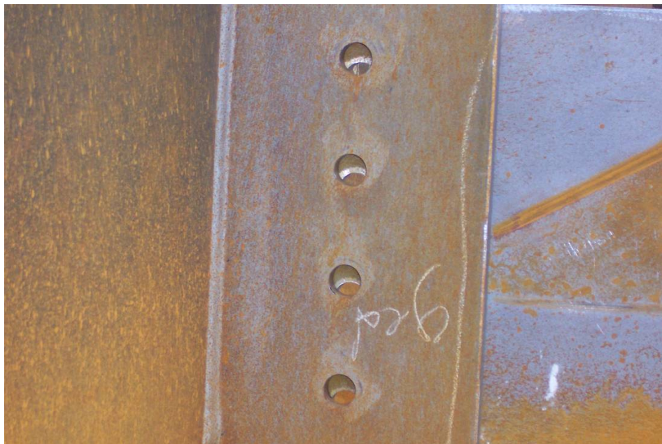
Figure 4.25. EICSS1, Steel Overpass Sunnyside Road I.C. (I-15B) over I-15, Bonneville Co. ID, bolt hole alignment during erection; for this job, drift pins were used to align the holes without mechanical aid (courtesy of Matt Farrar, ITD).
