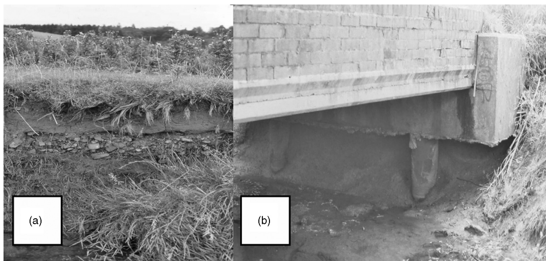
Fig. 1.8 An example of channel incision revealed by exposure of (a) a former bed level in the bank material. (b) Incision in this instance was a result of a land drainage scheme
