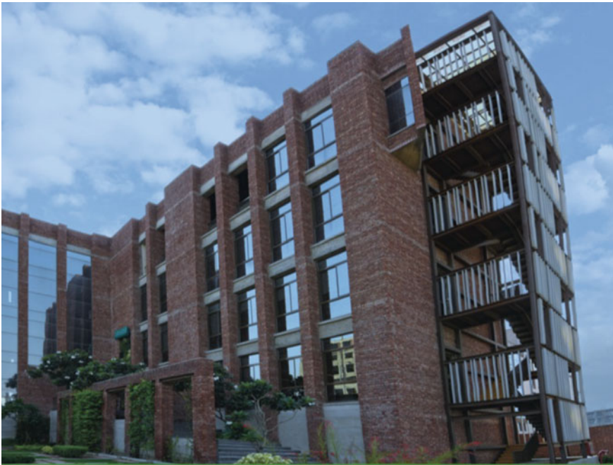
Fig. 9.2 Office Building of Design Associates Inc.—Uttar Pradesh. Source GRIHA India (2017)
