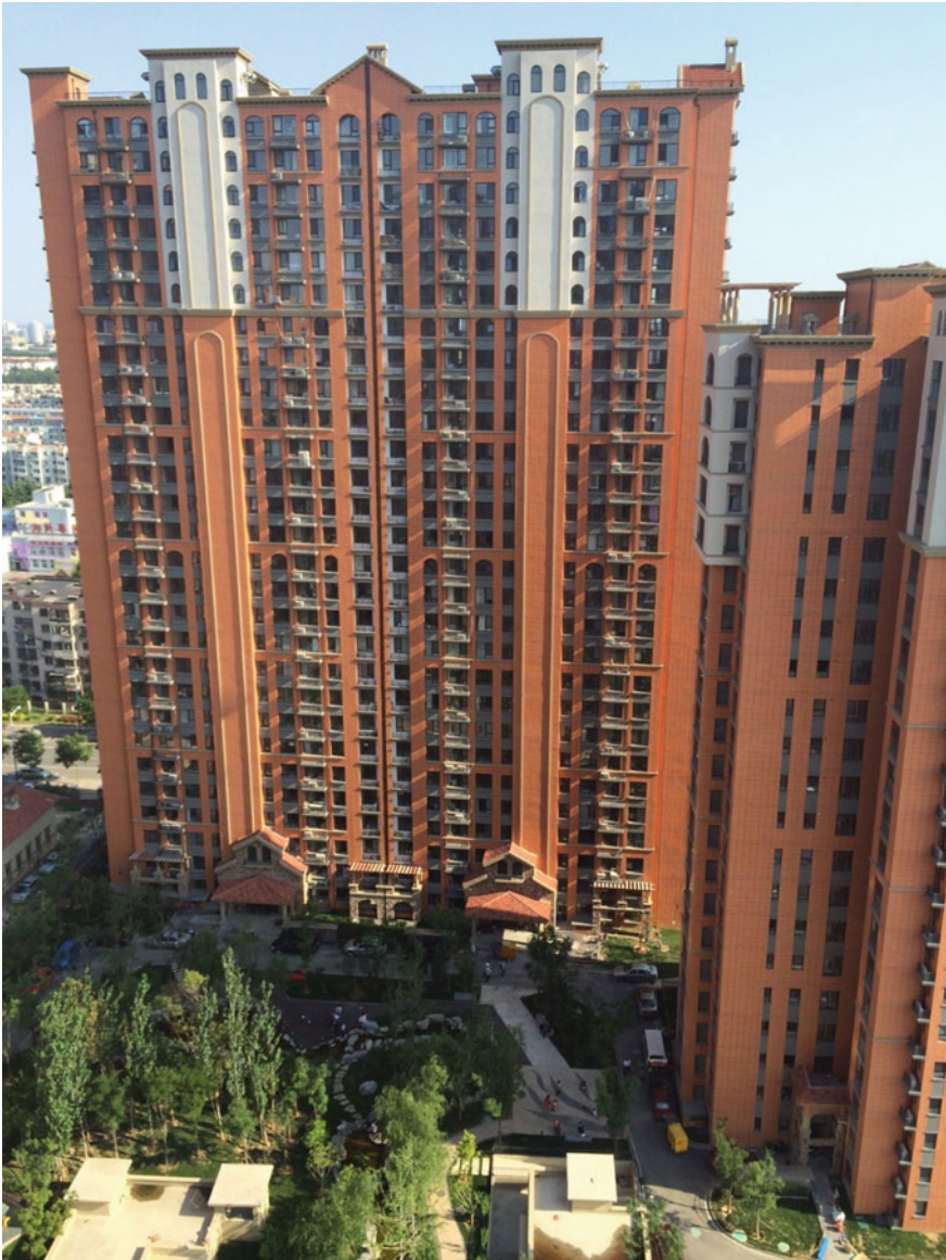
Fig. 7.6 A modern high-rise apartment in a suburban gated community in Beijing. Source Photo by the author, 2015
