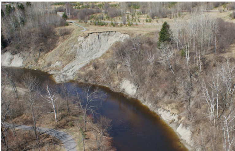
Fig. 26.2 Typical example of the most common types of landslides in Québec and the context in which they occur, namely along the meanders of watercourses where erosion is active (Source MTQ)
