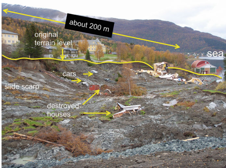
Fig. 27.1 Quick clay landslide in Lyngen in Norway, September 2010 (Photo: F. Oset, NPRA)
