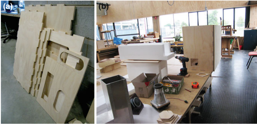
Fig. 13.39 a 12.5 mm plywood after being cut by the CNC router, b assembly and attachment of ironmongery
