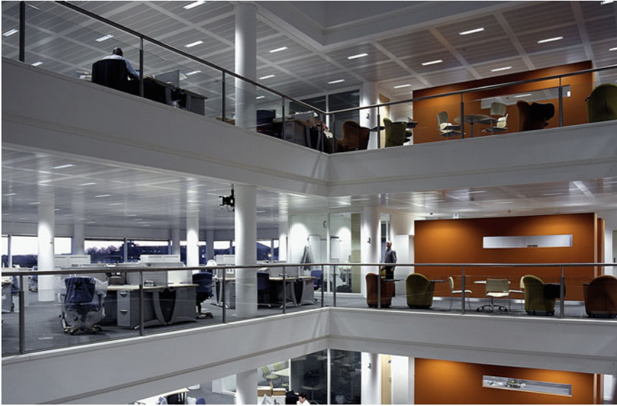
Fig. 8.4 Radiant passive chilled beams above a perforated ceiling system. ©2011 Frenger systems, reproduced with permission
