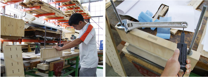
Fig. 13.53 Hanging scale being used to determine torque applied equally to both bolts on threaded rods
