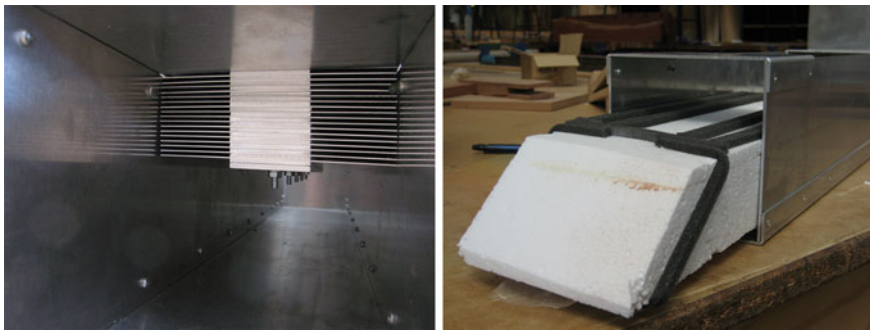
Fig. 13.31 Cooling fins to half the duct height with lower half blocked with polystyrene. Foam tape around the polystyrene block prevented air flow from bypassing the cooling fins
