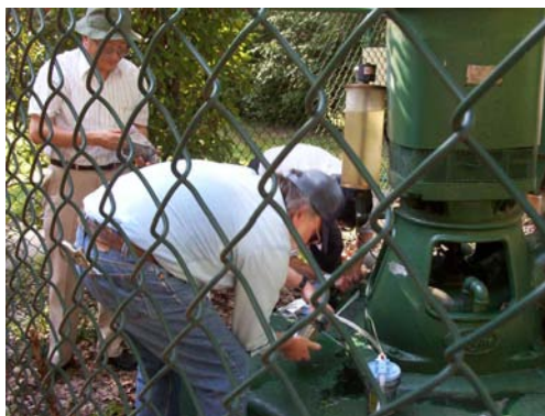
Figure 5.4: Photograph of uranium and thorium radioisotope filter equipment installation at a production well in the Sheahan Wellfield, Memphis, Tennessee. Shown are Dr. Teh-Lung Ku (left), Dr. John McCarthy (center) and Dr. Shangde Luo (right).
